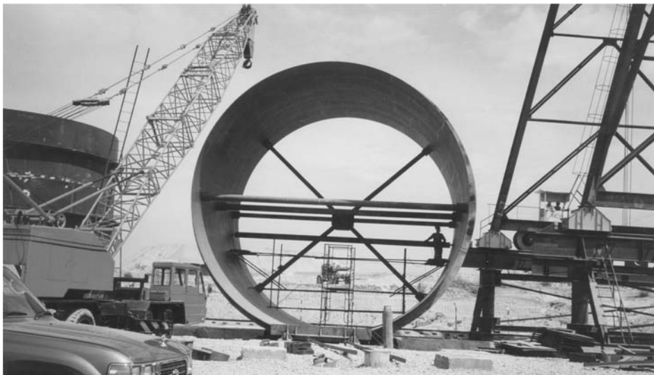
Plate 5a. Ten metre diameter steel can to form hydropower penstock, Ghazi Barotha Hydropower project, Pakistan 2001
