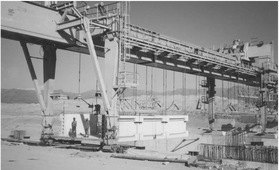
Plate 11b. A sophisticated gantry for handling and placing pre-cast concrete bridge and other units. Ghazi Barotha Hydropower project, Pakistan 2001
