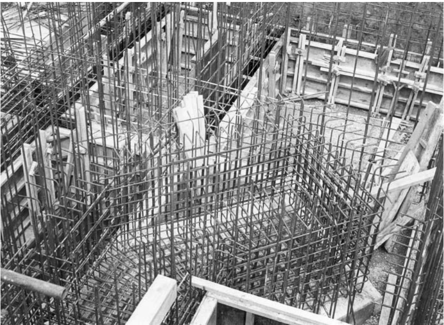
Plate 14b. Reinforcement must be accurately dimensioned and bent, and laps must be provided that permit the steelfixer to make adjustments for unavoidable discrepancies in the concrete work
