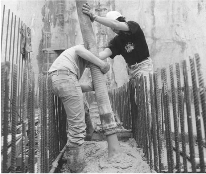
Plate 14a. The typical fluidity of pumped concrete; but it still needs vibrating in place
