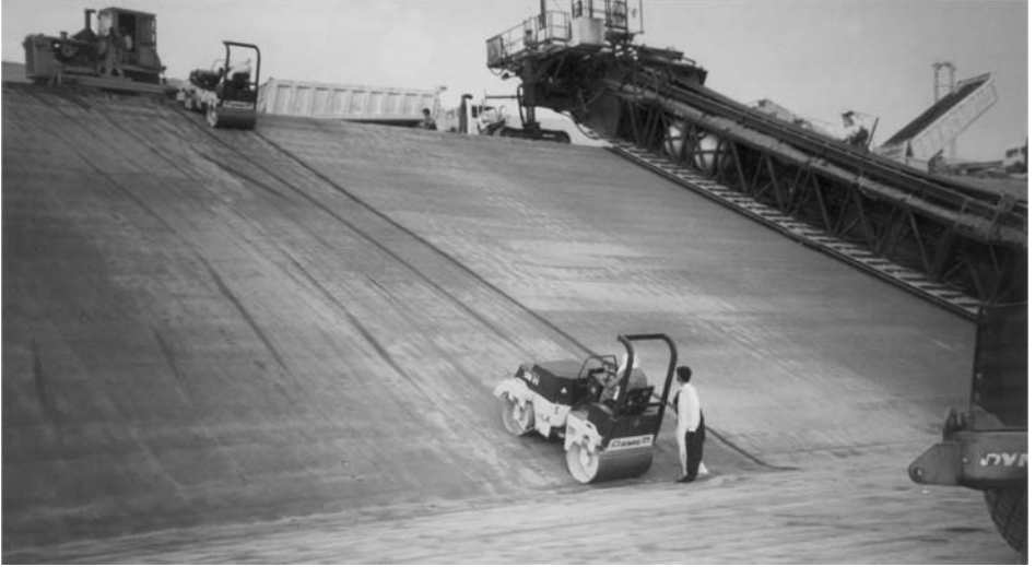
Plate 4a. Rollers compacting side slopes of power channel; filter layers and concrete to follow. Ghazi Barotha Hydropower project, Pakistan 1999
