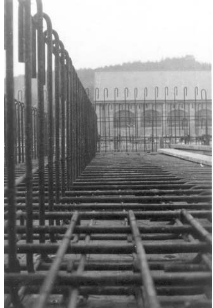
Plate 16b. Accurately placed reinforcement, strong enough to walk on
