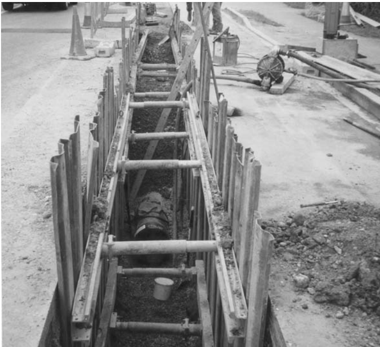
Plate 9b. A properly supported trench
