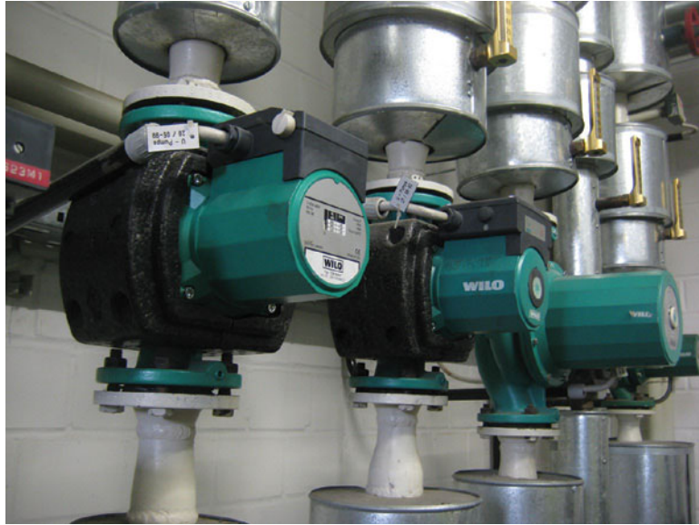
Figure 9.2 Pumps vertically in line
