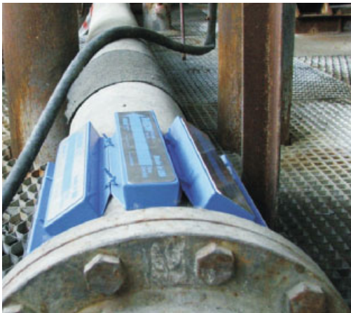
Figure 1.1 Water 'treatment' magnets and 'electronic descaler' – might as well be an ornament
