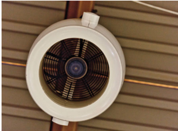
Figure 9.4 De-stratification fans
