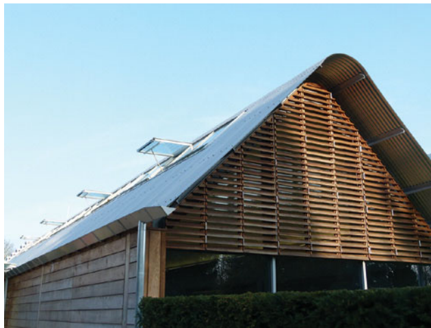
Figure 9.11 A good combination of high level natural cross flow ventilation and effective use of louvres to mitigate passive solar gain
