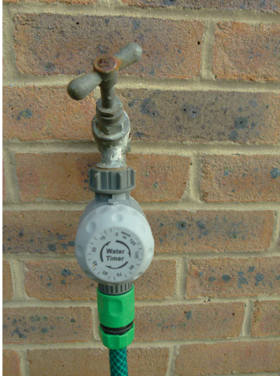
Figure 7.10 A simple 'clockwork' water timer
