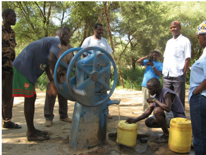
Figure 16.3 An effective hand pump to utilise water from a well (credit: Practical Action)
