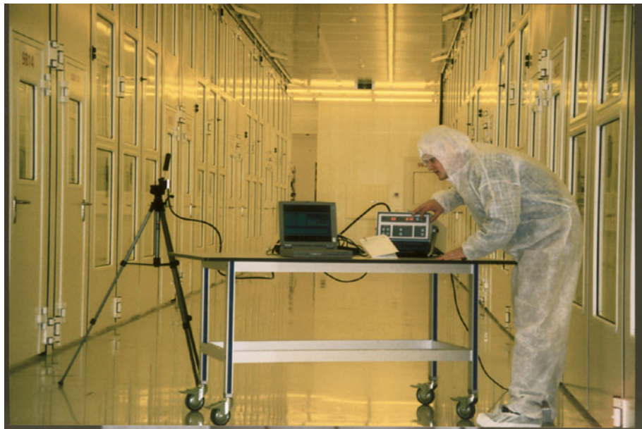
Figure 11.12 Specialist commissioning – cleanroom validation
