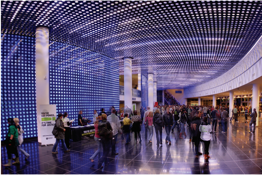
Figure A-5. Arrays of small RGB LED lighting fixtures can be configured to function as low-resolution image display systems, as in the lobby installation pictured above. Photo credit: Moritz Wade/perceptual.de provided courtesy of LightWild. Architects and Designers: Populous, JSK Architects, Tropp Lighting Design, Schmidhuber & Partner, and ICON Venue Group.
