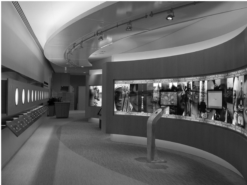
Figure 4-1. Recessed linear cove lighting provides for a visually comfortable environment by illuminating the ceiling and floor, and creates visual interest by outlining and accentuating these curvilinear display walls. Photo & Lighting Design: Michael Stiller Design.
