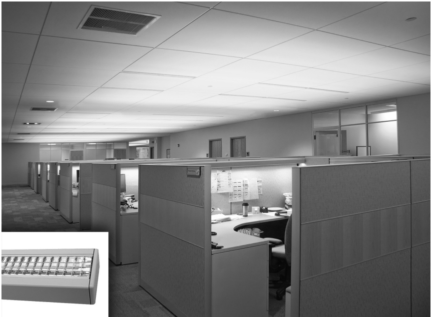
Figure 8-6. Partition mounted direct/indirect fixtures create a complete task-ambient scheme with one fixture type. Photo credit: The Lighting Quotient, Bic Corporation, Shelton, CT., Architect: Fletcher Thompson
