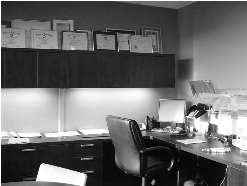
Figure 8-2. Fluorescent strip task lighting mounted to the underside of a cabinet is an easy and cost-effective method to provide greater illuminance on the desktop.
