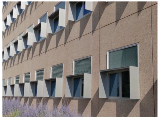
Figure 7-19. Windows on the south side of the RSF buildings. View windows are shaded by surrounds but admit some direct solar heat in winter. Above the view windows are daylight windows, which have no shade but block direct solar heat gain with louvers that reflect daylight toward the ceiling deep in the space. (Photo by the author)
