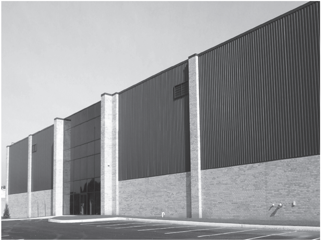
Figure 5-16. South elevation for case study of solar ventilation air preheat on a commercial building at Grant Way Facility, Allentown, Pennsylvania, showing transpired solar collector and by-pass dampers. (Photograph courtesy of Dick Bus, ATAS International Inc.).
