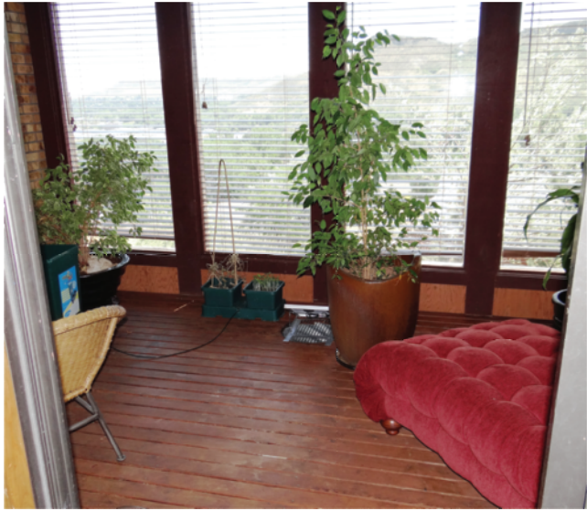
Figure 7-8. Sunspace with rock-bin storage under transpired floor at solar home in Golden, Colorado. Air duct into rock bin is visible in center of the south side of the room. (Photo by the author)
