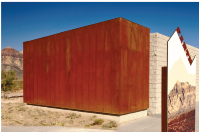
Figure 7-16. The transpired solar collection wall captures as much as 80 percent of available solar radiation to heat ventilation air for the restrooms. (Photo by Robert Reck, courtesy of Line and Space LLC)
