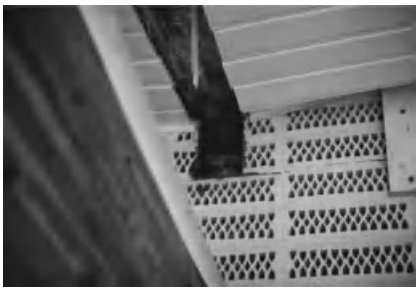
Figure 11.1. In-door swimming pool, low-sloped roof with timber deck, one of the main beams collapsed due to wood rot at the support.
