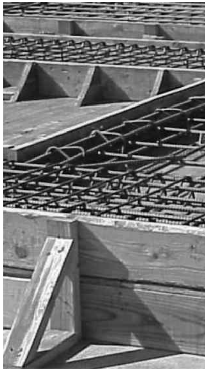
FIGURE 5.4 Strengthening wood form for ground slab.
