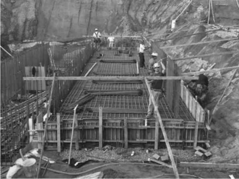
FIGURE 5.14 Steel bars between foundation and wall.
