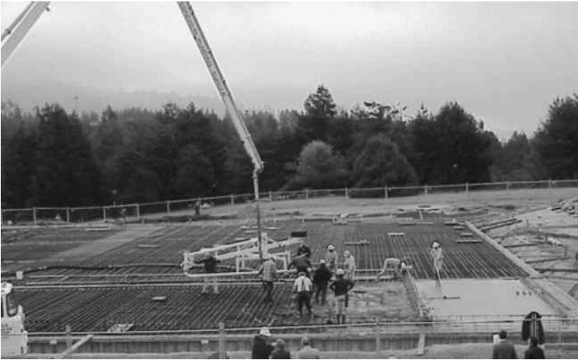
FIGURE 5.24 Pouring raft foundation by using pump.
