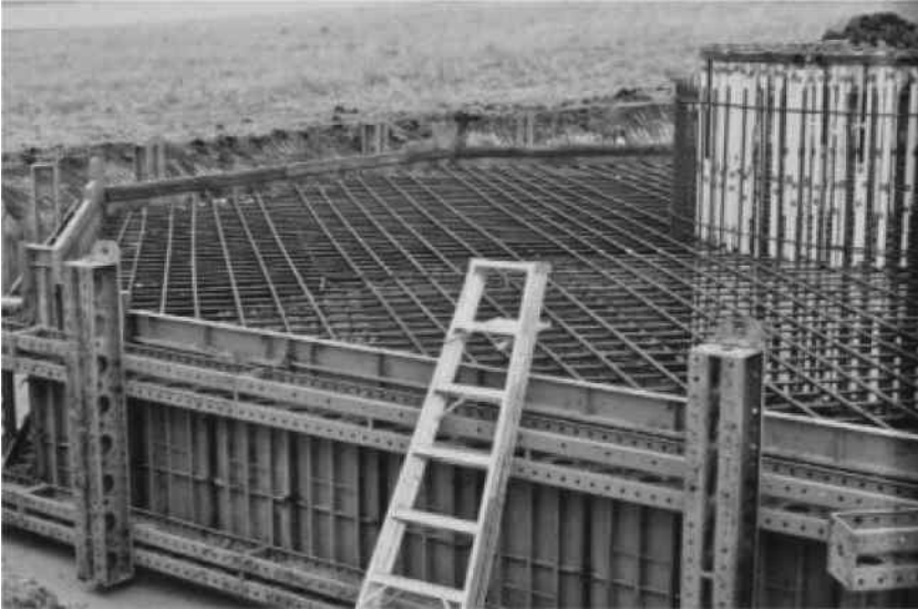
FIGURE 5.5 Steel form for raft foundation.
