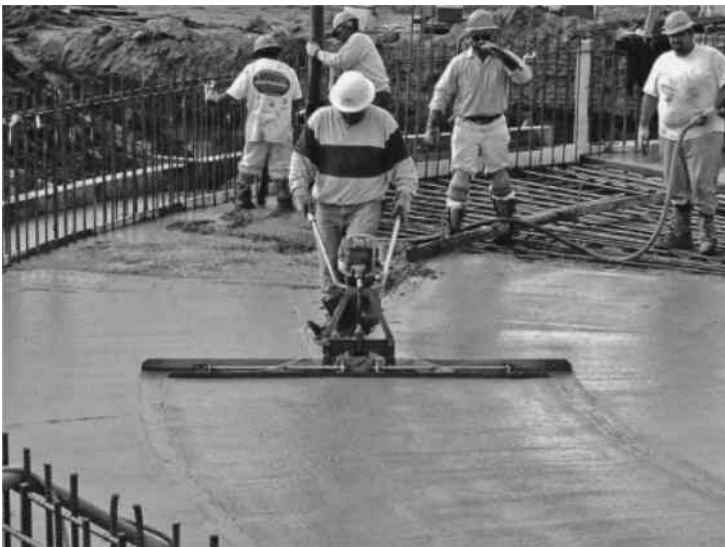
FIGURE 5.29 Finishing the concrete surface.
