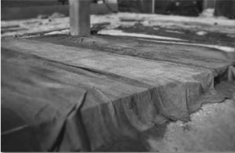
FIGURE 5.35 Curing by using textile.
