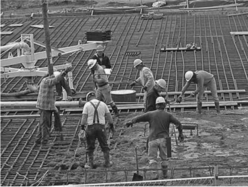
FIGURE 5.25 Pump concrete in pouring a slab.
