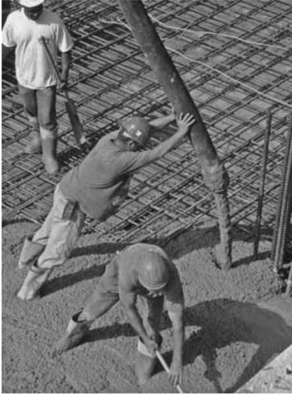
FIGURE 5.28 Preparing concrete surface.
