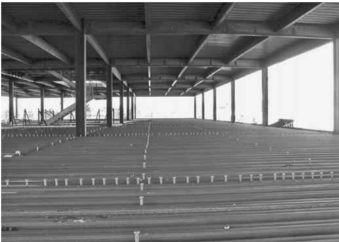
FIGURE 7.58 Stud bolts in roof slab.
