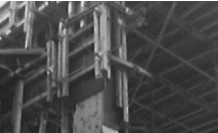
FIGURE 5.7 Steel supports with marine plywood.
