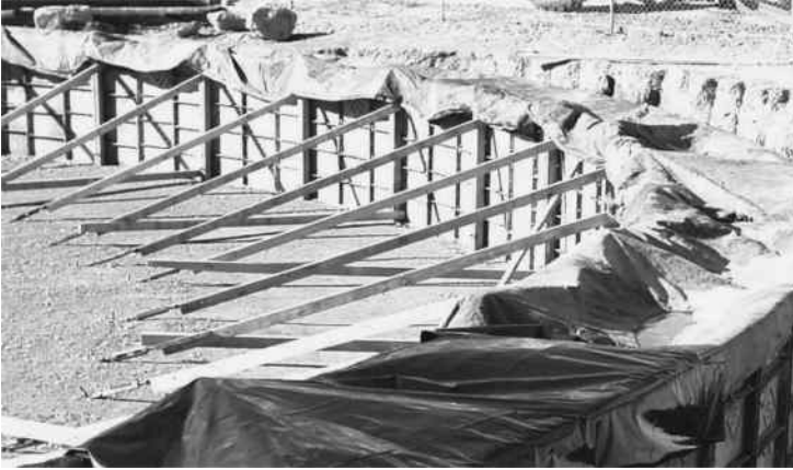
FIGURE 5.37 Plastic sheet to protect from evaporation.
