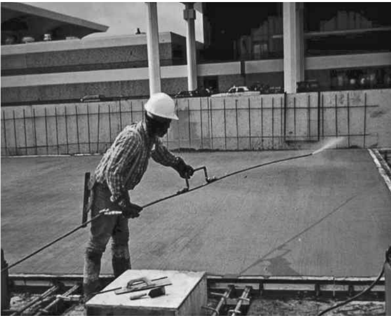
FIGURE 5.49 Spraying chemical compound on the surface.
