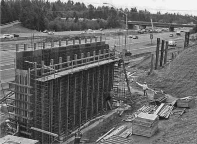
FIGURE 5.1 Formwork for reinforced concrete wall.
