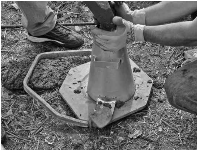
FIGURE 4.12 Pouring concrete in slump.
