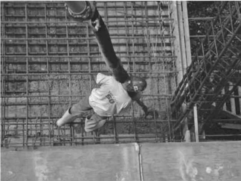
FIGURE 5.26 Pump concrete in pouring a slab.
