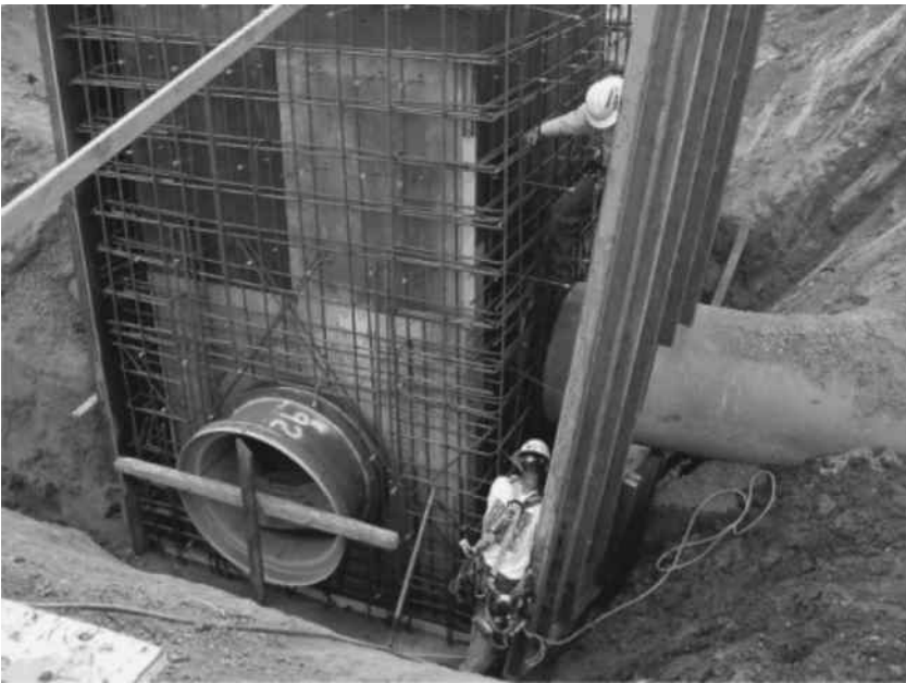
FIGURE 5.13 Wall steel bars with pipe sleeve.
