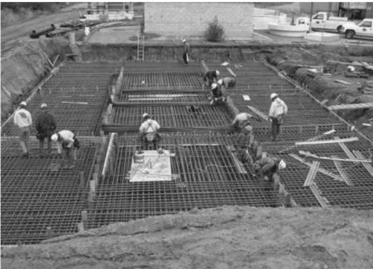
FIGURE 5.15 Distributing steel reinforcement in concrete raft.
