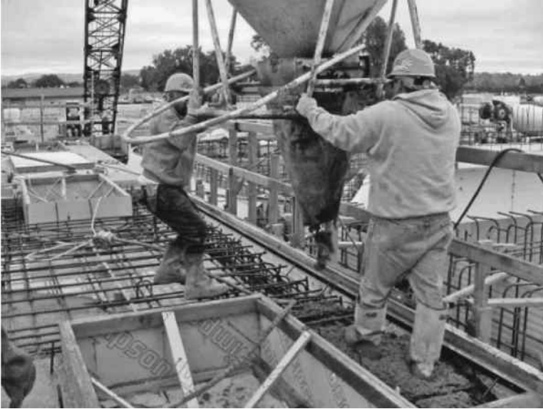
FIGURE 5.27 Pouring beam by using caisson.
