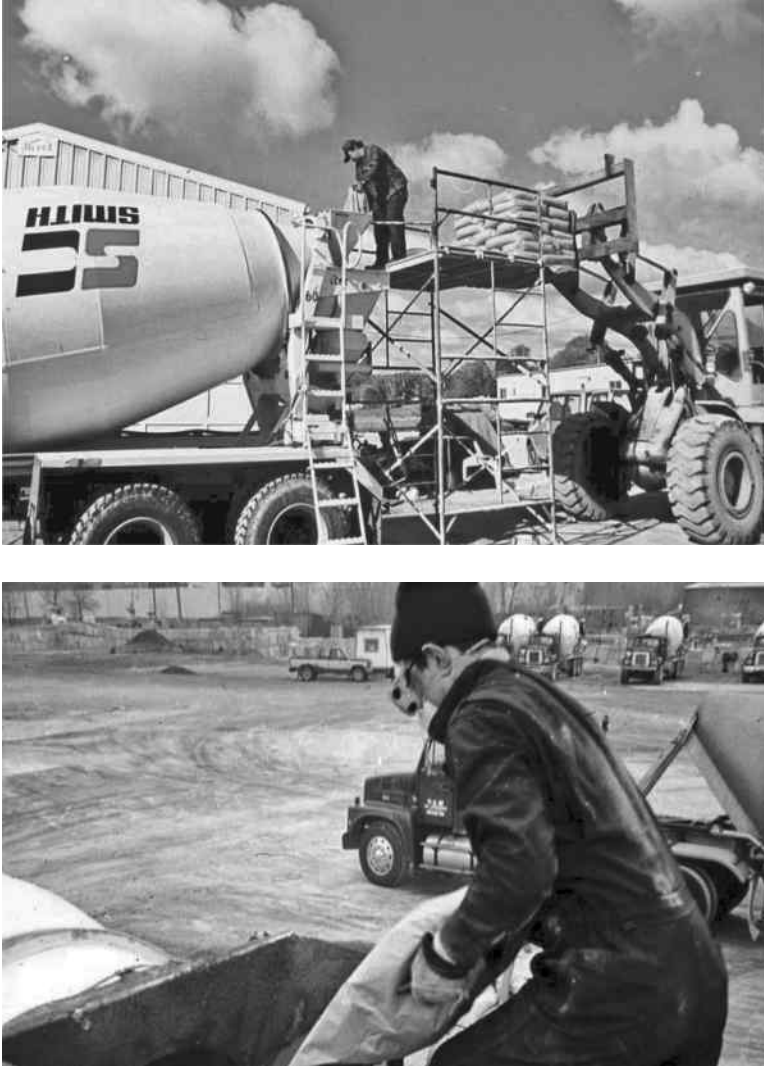
FIGURE 5.47 Putting sacks of silica fume in truck mixer.
