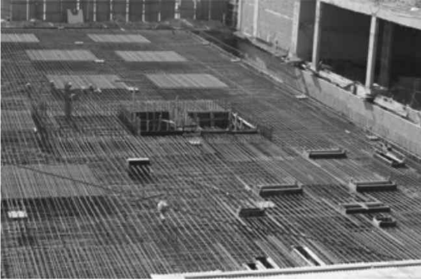
FIGURE 5.12 Steel bars for raft foundation.
