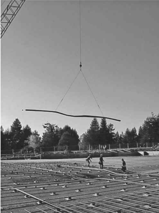
FIGURE 5.11 Distributing steel bars for ground slab.
