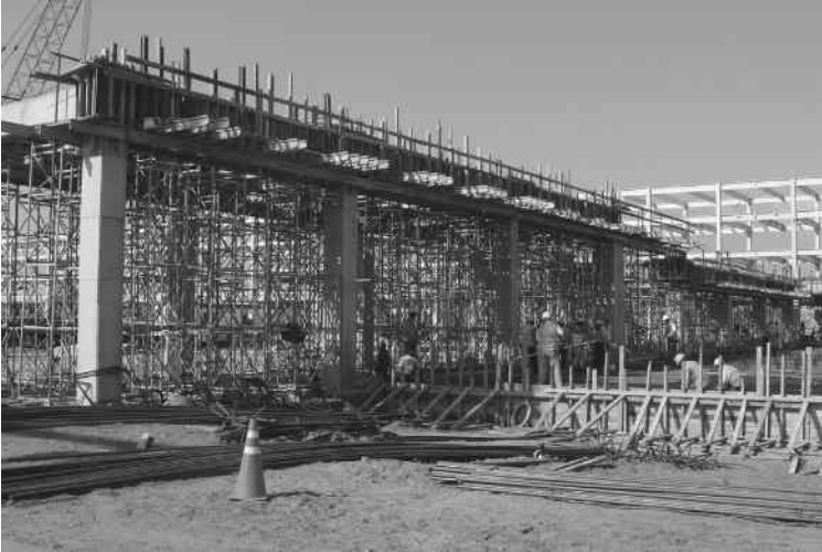
FIGURE 5.3 Wood form for concrete columns.
