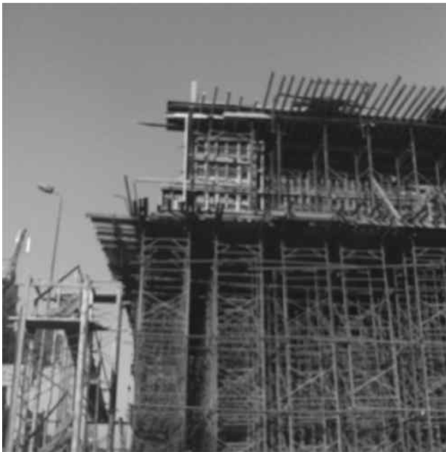
FIGURE 5.2 Bridges and slab form support.
