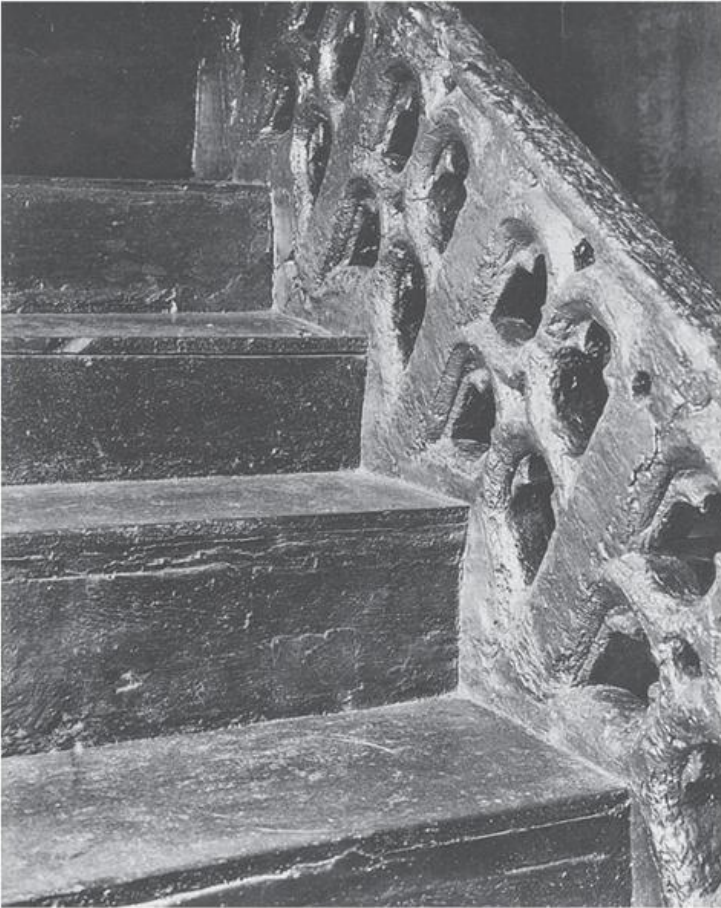
2.12 Downholland Hall, near Ormskirk (early sixteenth century). (Godfrey)
