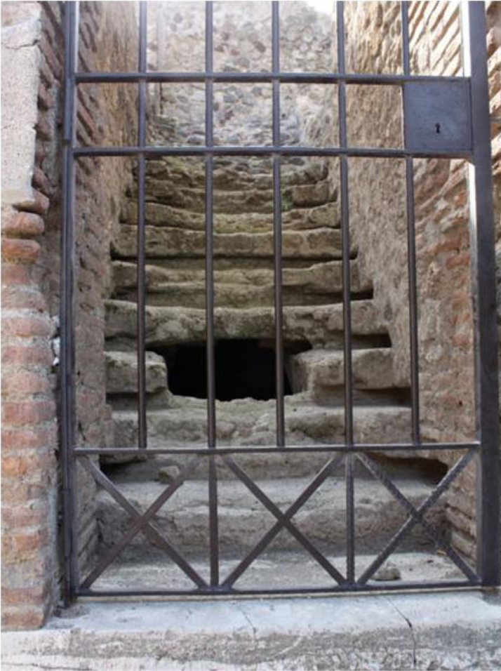
1.21 Staircase in the Vicolo della Terme, Pompeii. There is a chute into, or ventilation for, the cellar below and a staircase down to that cellar immediately to the right. The treads were originally overlaid with a different material, the insets for which can be clearly seen. This has either perished or has been removed or stolen. It may
