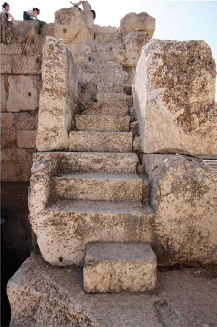
1.16 Baalbek, Lebanon, Temple of Jupiter, ceremonial staircase forming part of the monumental altar, one of a pair either side of the altar. Huge blocks of stone are
