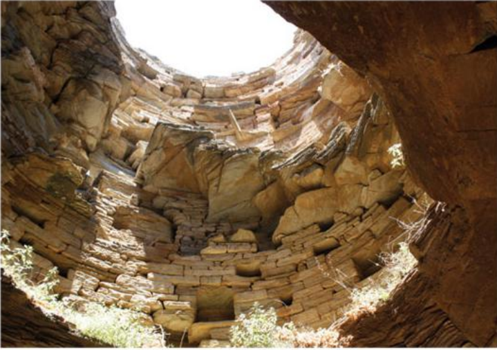
1.4 Remains of the cantilevered staircase in the tower of Agios Petros on the island of Andros. Taken from the ground-floor vaulted room through the collapsed crown of the vault. (Michael Tutton)
