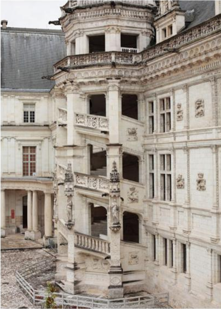
1.42 Blois, France, exterior of the main staircase of the Francois I wing. (Peter Stone)
