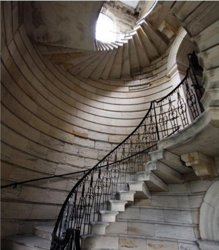
2.21 Winding Staircase c. 1724 at Seaton Delaval. (Michael Tutton)
