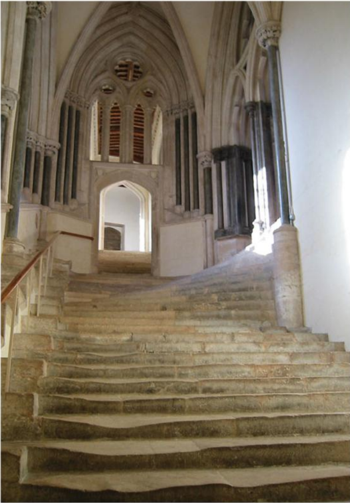
2.7 Cathedral Stair at Wells leading to Chapter House (right). (James Campbell)
