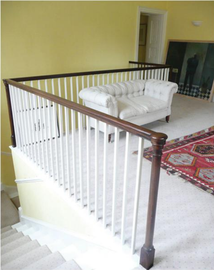
9.7 Dauntsey Park staircase, first floor with well infilled. (Donal Channer)
