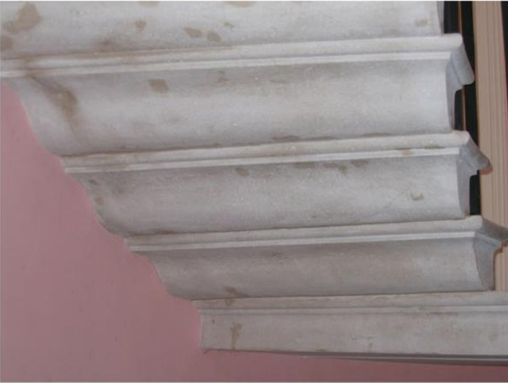
10.10 Beautifully worked soffit to stair treads, showing previous resin patch repairs. (Cliveden Conservation)
