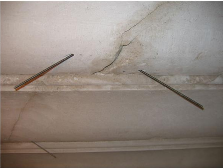
10.10 Beautifully worked soffit to stair treads, showing previous resin patch repairs. (Cliveden Conservation)
