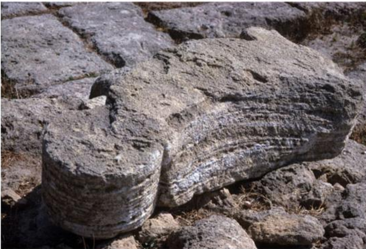
1.8 Temple A at Selinunte, Sicily. Stair tread c. 450 BC. Here is clearly seen the precursor of the newel stair seen in virtually every house, fortress and church of the Romanesque and Medieval periods. (Margaret M. Miles)
