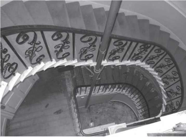
7.6 Stair with later iron column inserted, which the client wished to remove.
