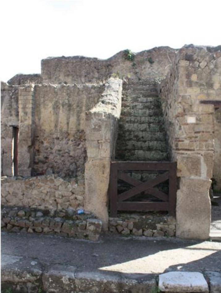
1.22 Staircase leading from the street to an upper floor in Herculaneum. (Michael Tutton)
