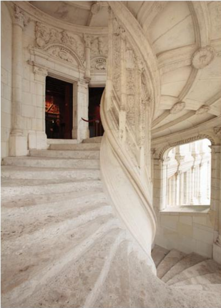
1.41 Blois, France, the main staircase of the Francois I wing. (Peter Stone)
