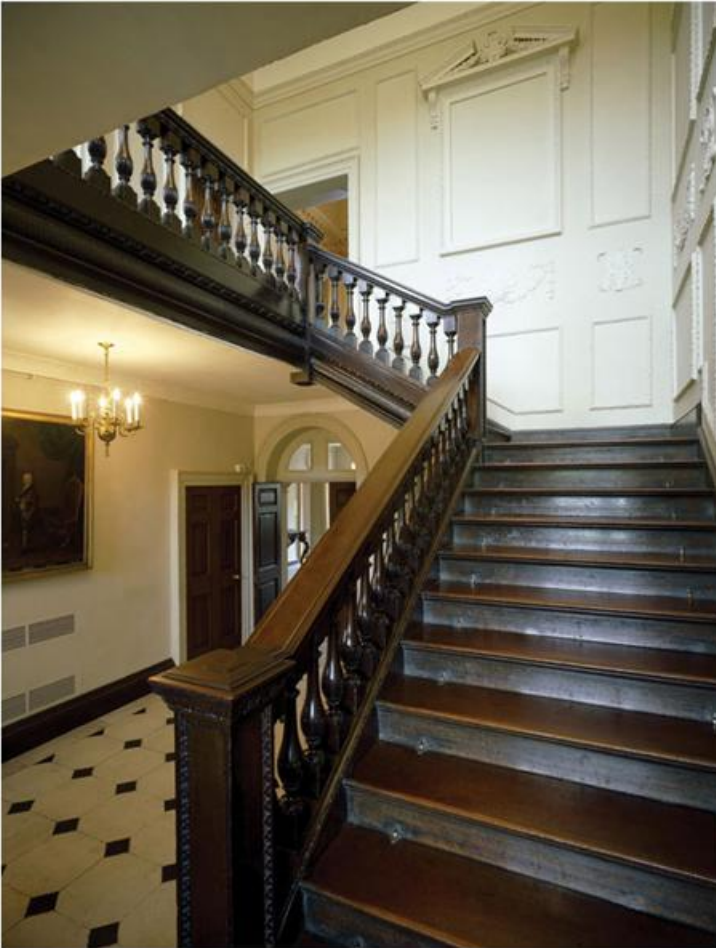
4.12 Marble Hill House, Twickenham, West London. A mahogany closed-string staircase, c. 1730. This is a very old-fashioned design and reflects the taste of at least the 1670s and probably earlier, but it is made of the newly fashionable West Indian mahogany. Even the flooring of the piano nobile is all constructed of this expensive timber. (Courtesy of English Heritage)
