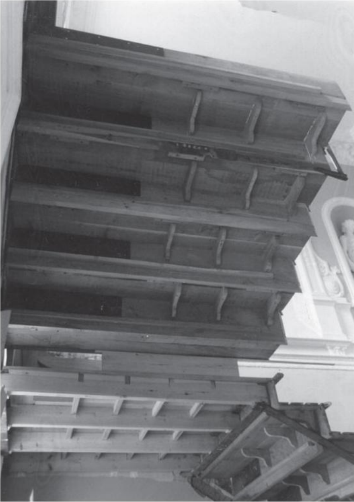
9.11 The Queen Square staircase under construction. (Donal Channer)
