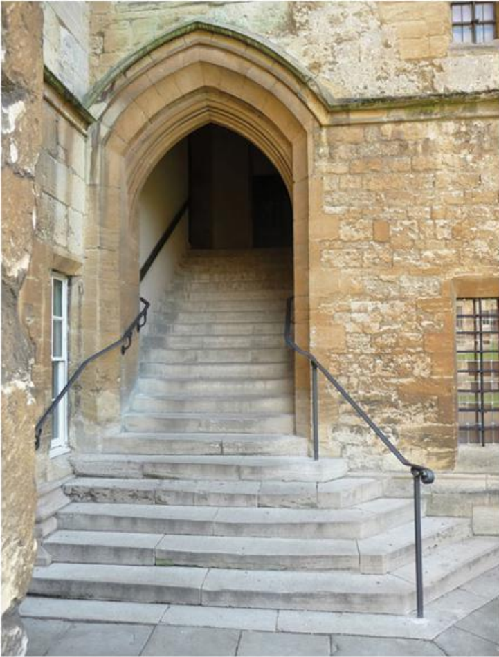
2.11 Staircase to dining hall, New College, Oxford. (Stephen Oliver)
