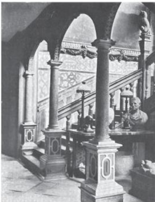
2.15 Knole in Kent, with decorated newels, but here the balusters are turned. (Lloyd)
