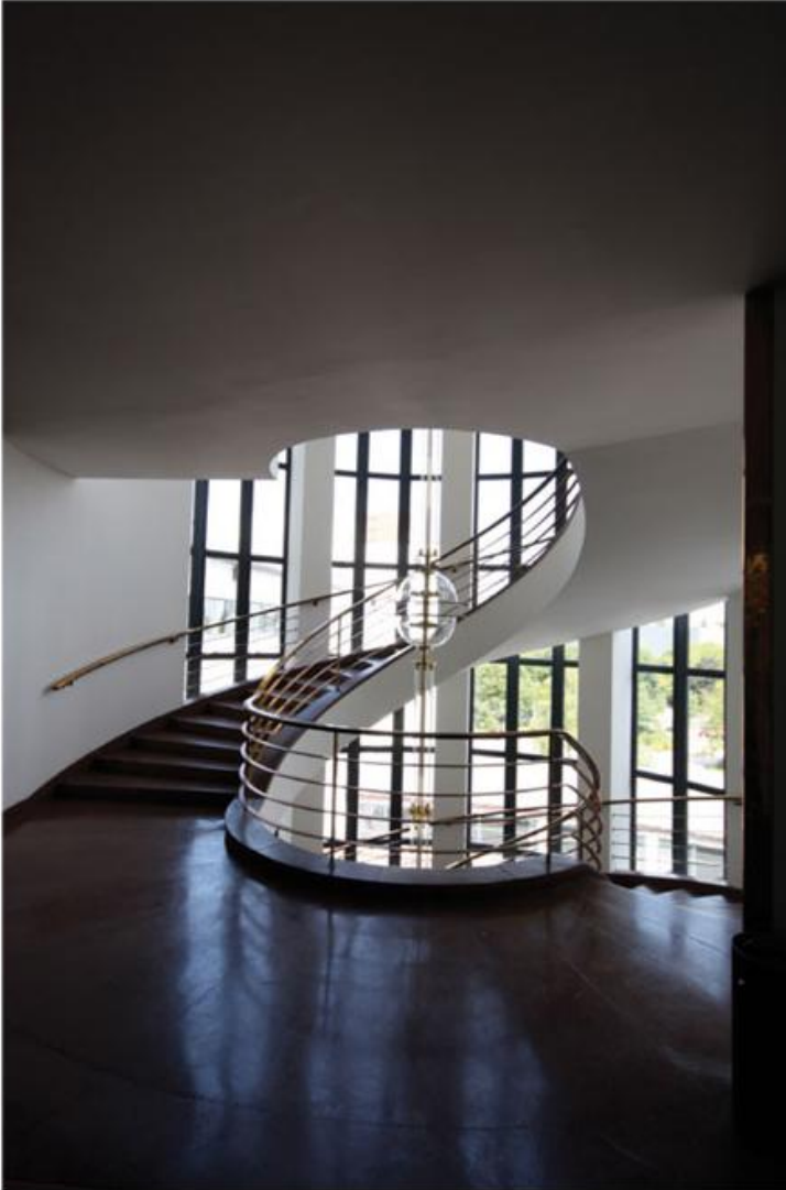
1.70 Berlin, Metal Workers Union building, Erich Mendelsohn. The balustrade and central light fitting, which is suspended throughout its full height of six
