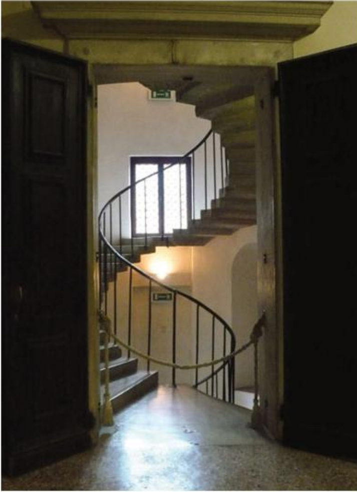
1.49 Cantilevered staircase, c. 1561, in the Convento della Carita in Venice, by Andrea Palladio. (Helen Rogers, www.stonestairs.net )
