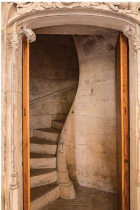
1.30 Palma de Mallorca, Llotja, spiral vault staircase designed by Guillem Sagrera, built 1426–1446. (Jose Calvo-Lopez and Alberto Sanjurjo-Alvarez)
