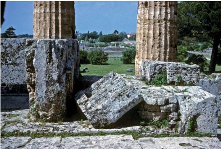
1.10 Paestum, Temple of Hera II. Block of three stair treads, resting at an angle, in the middle foreground. (Margaret M. Miles)
