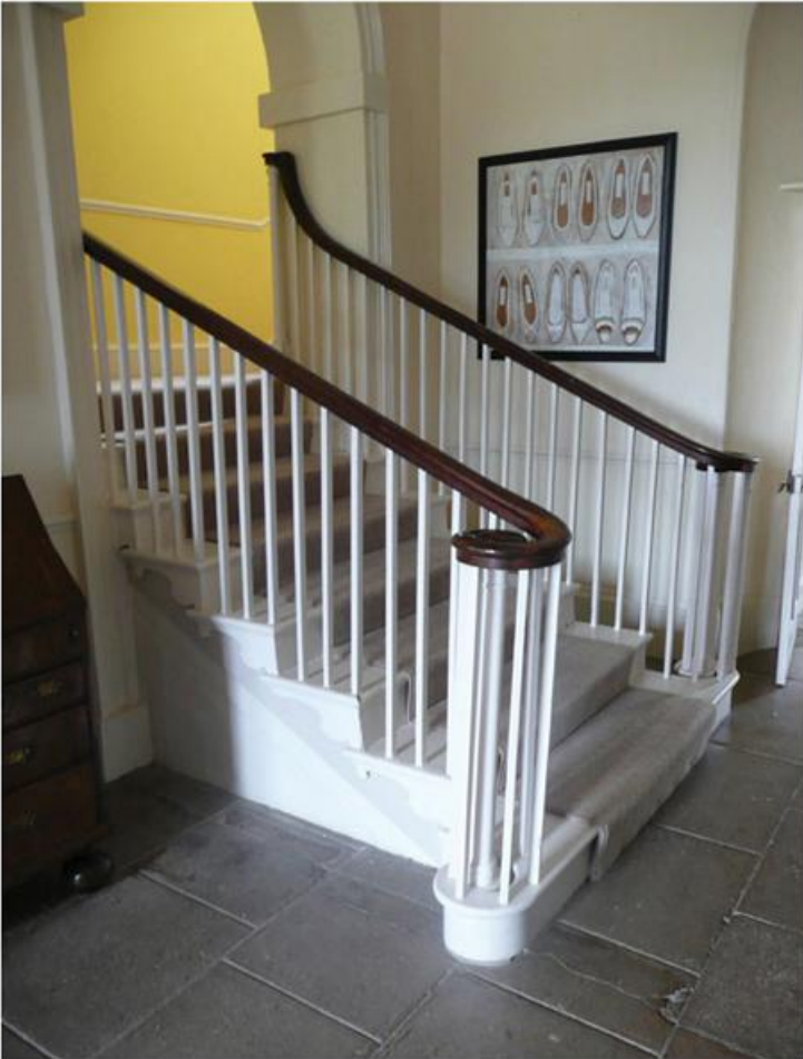
9.6 Dauntsey Park staircase before intervention. (Donal Channer)
