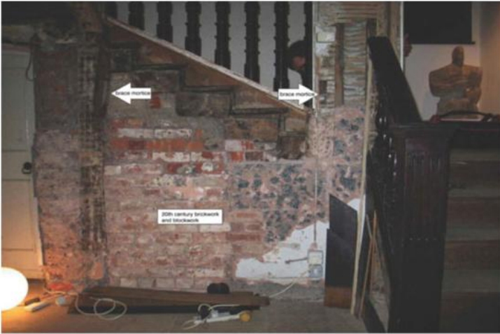
5.10 Second flight at Whitestaunton, showing the complete structural history. (Michael Heaton)
