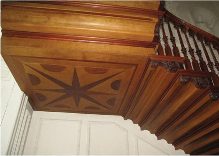
9.12 Queen Square, the completed staircase showing the soffit of the second quarter-landing. (Donal Channer)
