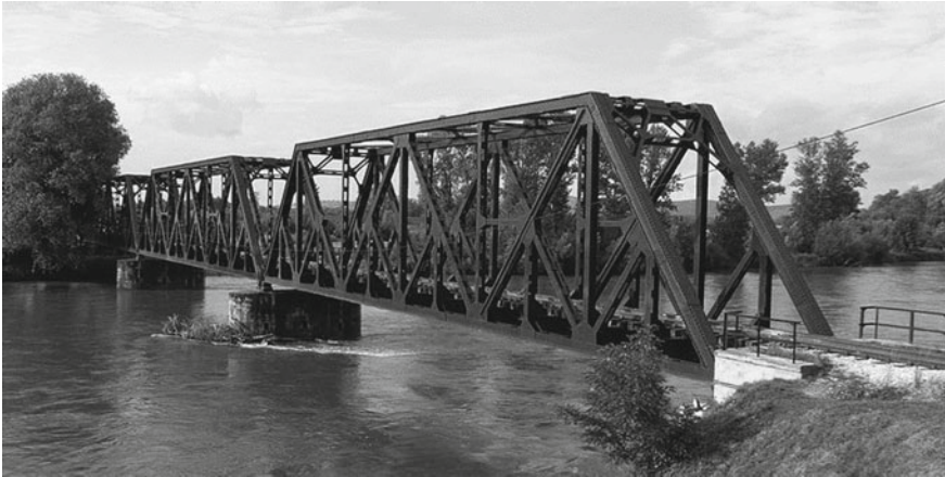
Fig. 9.24 Through truss bridge
