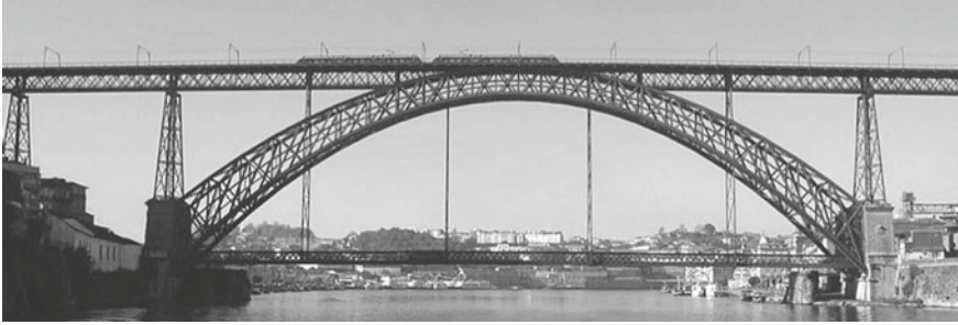
Fig. 9.1 A railway track above the bridge superstructure
