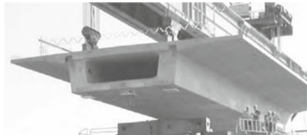
Fig. 9.15 Deck with two prefabricated box girders and cast-in place slab. Source Cirillo et al. [6]
