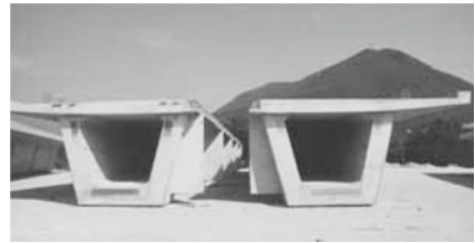
Fig. 9.15 Deck with two prefabricated box girders and cast-in place slab. Source Cirillo et al. [6]
