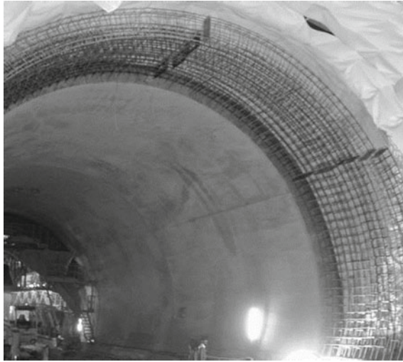
Fig. 10.12 Concrete casting
