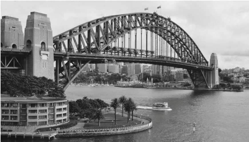
Fig. 9.2 Railway track and deck placed below the arch of the bridge
