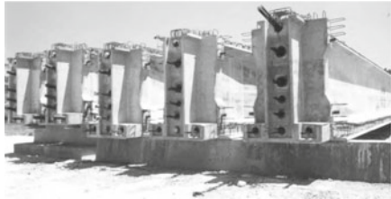
Fig. 9.14 Deck with four prefabricated I-beams and cast-in place slab. Source Cirillo et al. [6]
