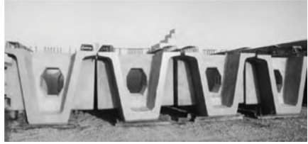
Fig. 9.13 Deck with four prefabricated box girders and cast-in place slab. Source Cirillo et al. [6]
