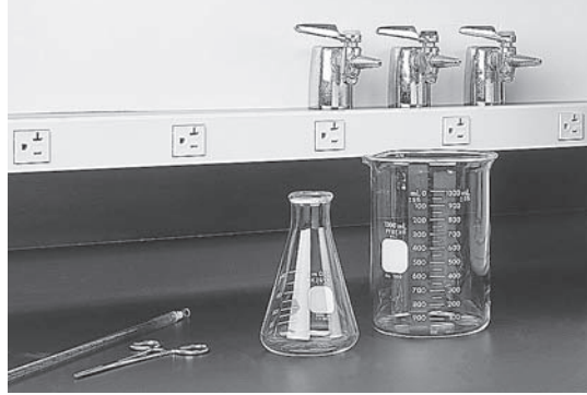
Fig. 27–23 A typical installation of the multioutlet assembly shown in Fig. 27–21. ( Wiremold )
