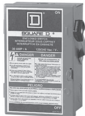
Fig. 30–2 This 30-amp switch may be used as the disconnecting means for small motors. This switch also has a horsepower rating and qualifies as a motor-circuit switch. (Square D)
