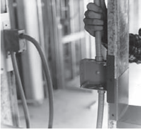
Fig. 11-24 This shows the corrugations on ENT, which allow it to be bent by hand (a “pliable” raceway according to the NEC definition). A snap-on connector has been added, which will lock in place when it goes into one of the knockouts in the box. (Carlson, a Lamson & Sessions company)
