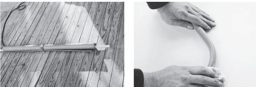
Fig. 11-22 A heating blanket for nonmetallic conduit. After making the bend, set it with a wet rag, as at right.
