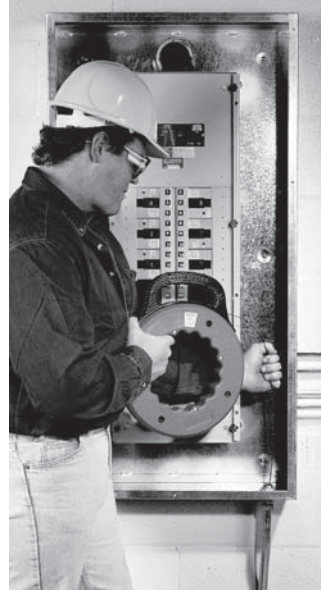
Fig. 11-13 Using fish tape to pull wires into conduit. (Klein Tools, Inc.)
