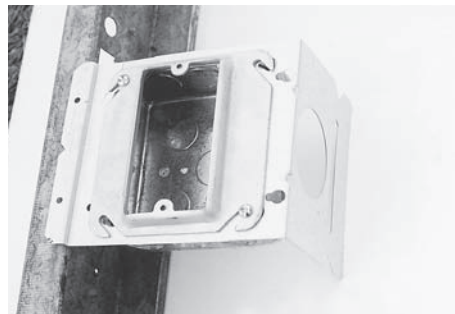
Fig. 10-21 These boxes have brackets that snap into metal framing members. The sheet metal bracket is arranged to bottom on the wallboard on the back side of the partition, providing additional stiffness to the box. This feature is particularly helpful at receptacle outlets.
