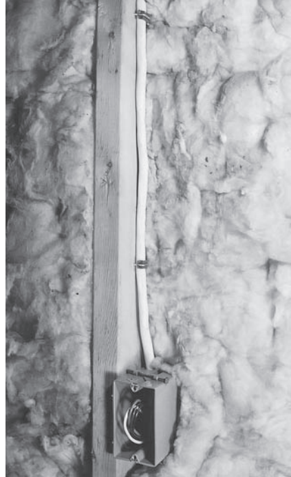
Fig. 11–30 Insulated staples help prevent damage to Type NM cable.
