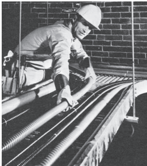
Fig. 27-31 Metal-clad cable, Type MC, being installed in a ventilated trough cable tray. (MP Husky Corp.)
