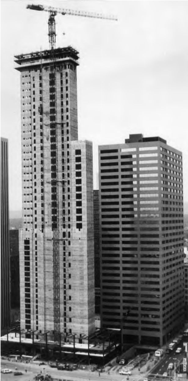
FIGURE 15-11 ARCO II Building in Denver, Colorado: 544-ft-high slipformed elevator shaft. (Source: Sundt Corporation)
