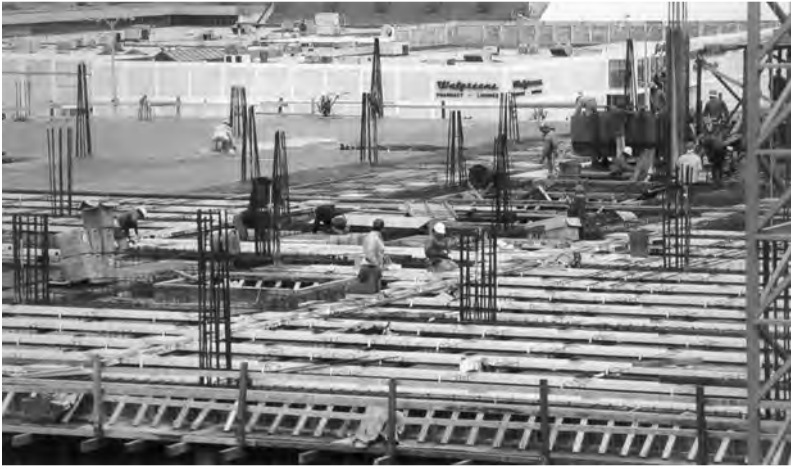
FIGURE 12-12 Installation of cellular units for an elevated floor system. (Source: H. H. Robertson Company)
