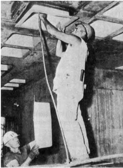
FIGURE 12-10 Removing a plastic mold with compressed air. (Source: MFG Concrete Forms Co.)
