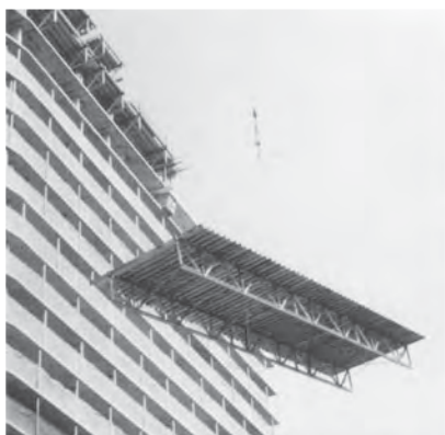
(a) Lifting a flying form table
