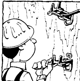
(5) Attach Quick-Lock brackets on all Quick-Lock ties and install lengths of 2 X 4 walers (see next picture).
