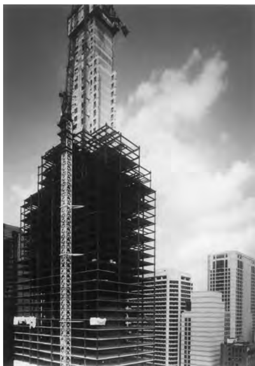
FIGURE 15-12 Slipform core of 785 ft for Two Liberty Place in Philadelphia, Pennsylvania.
