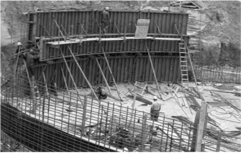
FIGURE 9-46 Gang forms for constructing a curved wall. (Source: EFCO)
