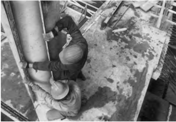
FIGURE 10-22 Opening form after pour. (Source: Symons Corporation)
