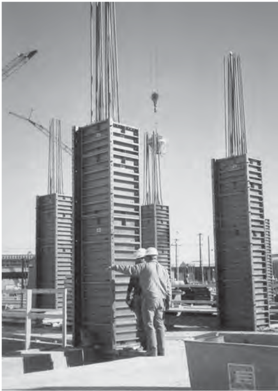
(a) Positioning all-metal column form
