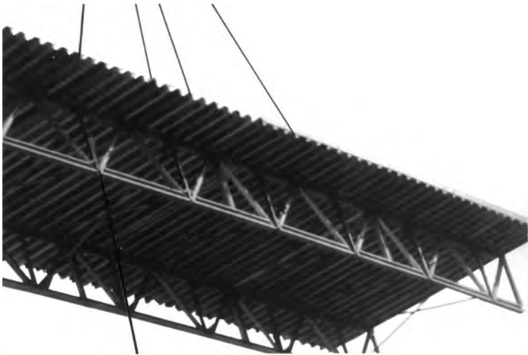
FIGURE 17-13 Lifting a flying form table unit to a new location. (Source: Patent Construction Systems)
