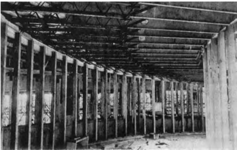
FIGURE 12-14 Installation of horizontal shores. (Source: Patent Construction Systems)
