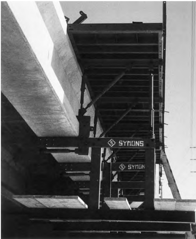
FIGURE 16-9 Adjustable bridge deck and overhang forming system. (Source: Symons Corporation)
