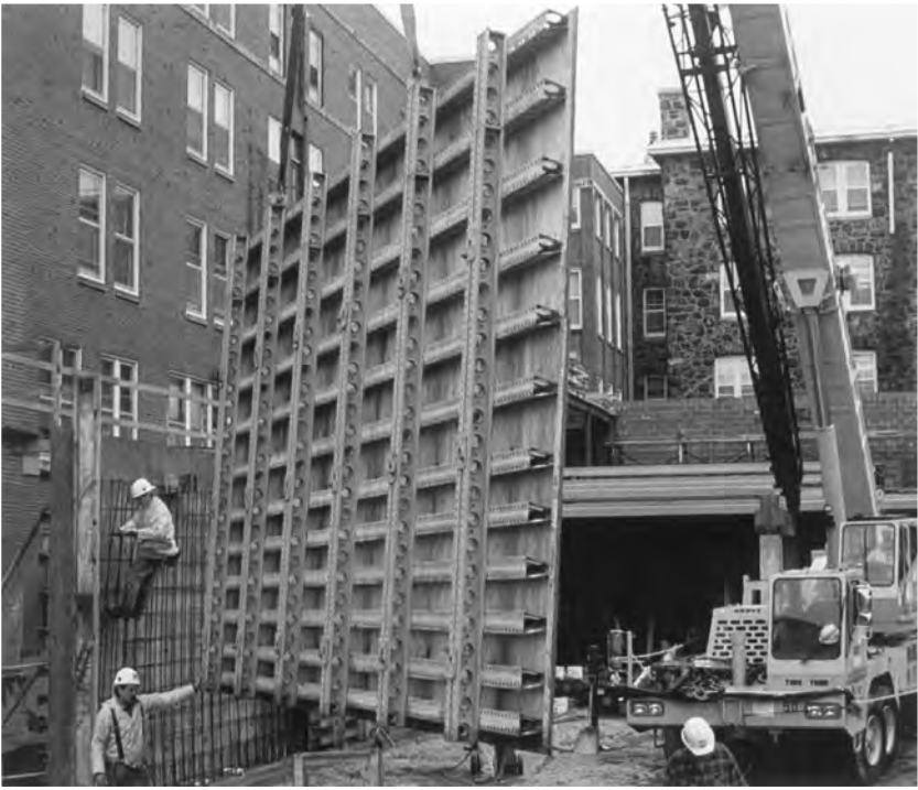
FIGURE 9-44 Wall-forming system. (Source: EFCO)
