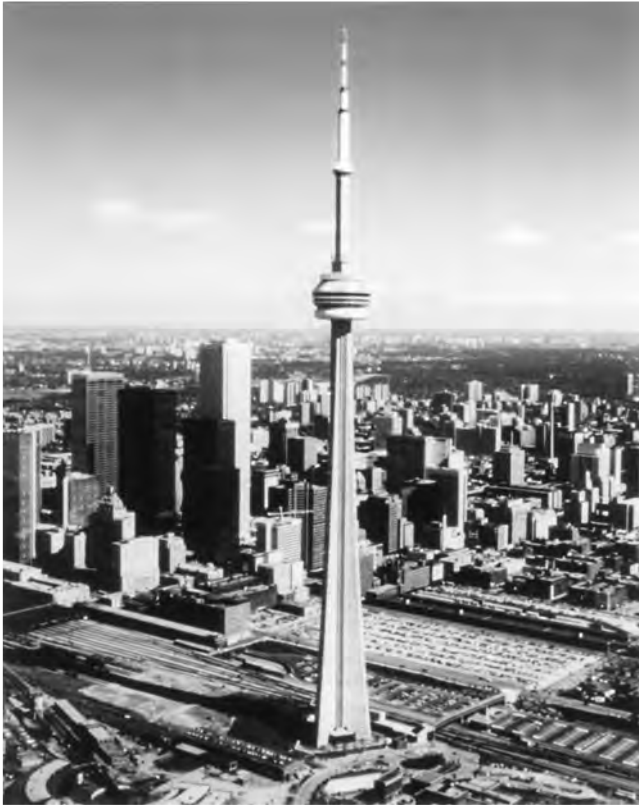
FIGURE 15-10 CN Tower in Toronto, Canada: 1,815 ft total height, 1,476 ft slipform height.
