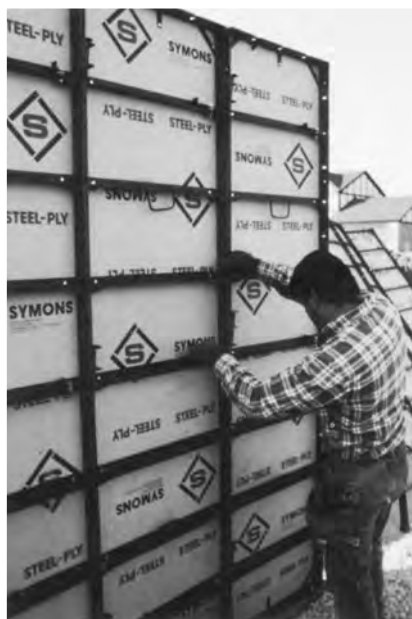
FIGURE 9-41 Hand setting modular panels. (Source: Symons Corporation)
