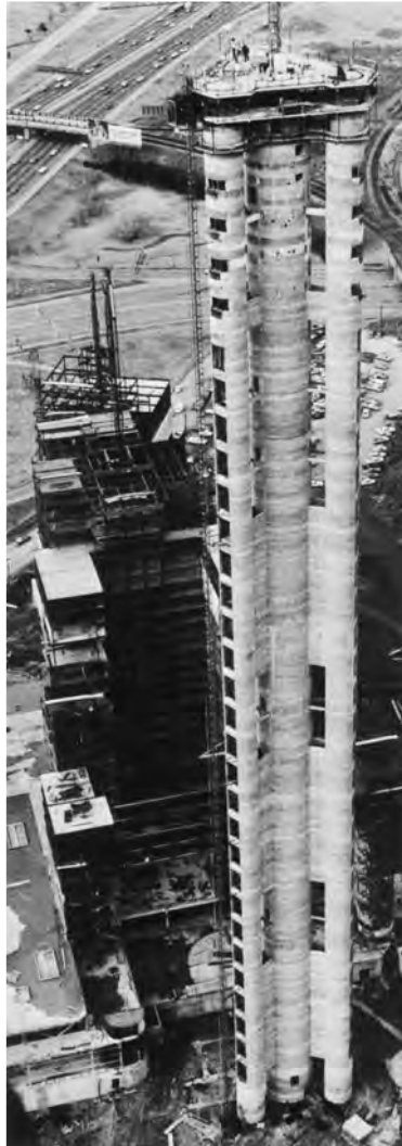
FIGURE 15-1 Reunion Tower constructed by slipform method. (Source: Sundt Corporation)
