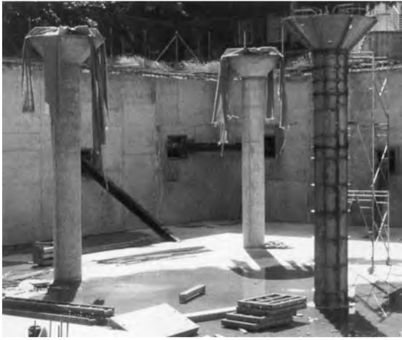
FIGURE 10-19 Steel column forms with capitals. (Source: EFCO)
