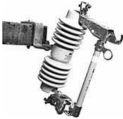
FIGURE 5.8 Typical pole-mounted fuse.
