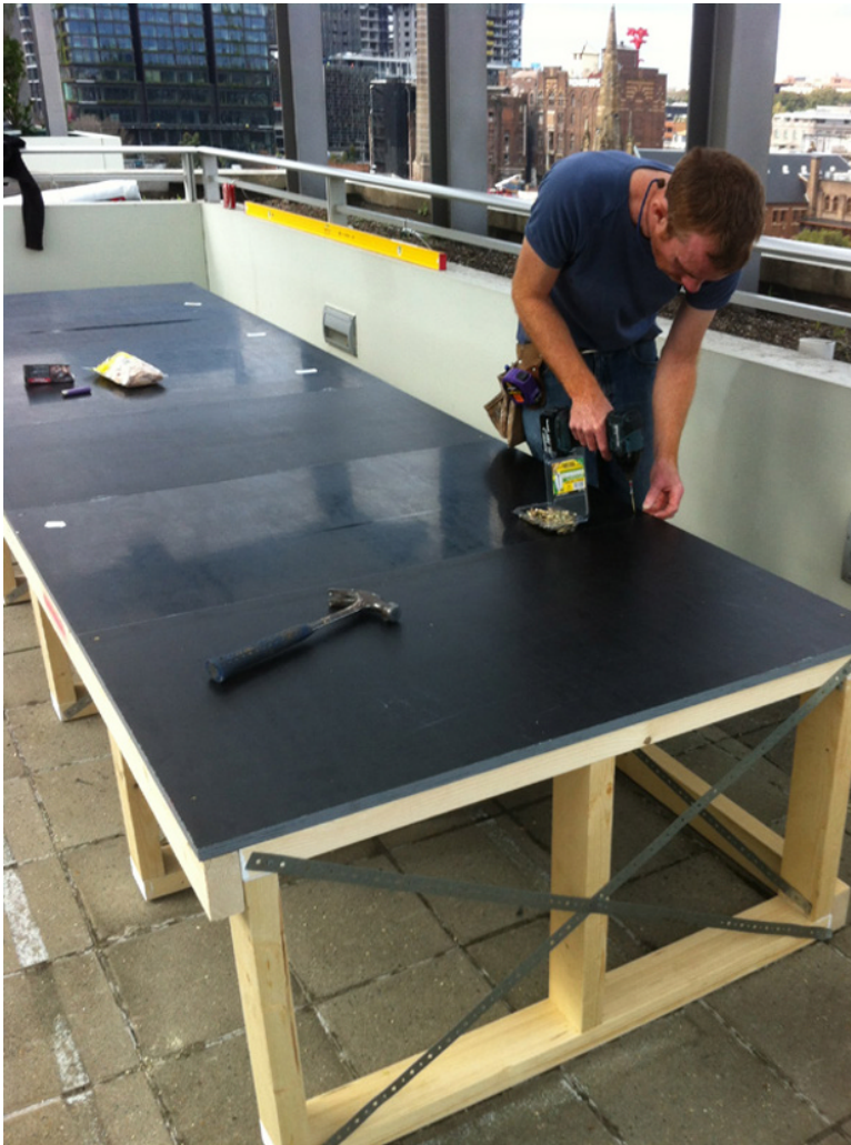
Figure 9.2 Gumal bed under construction.
