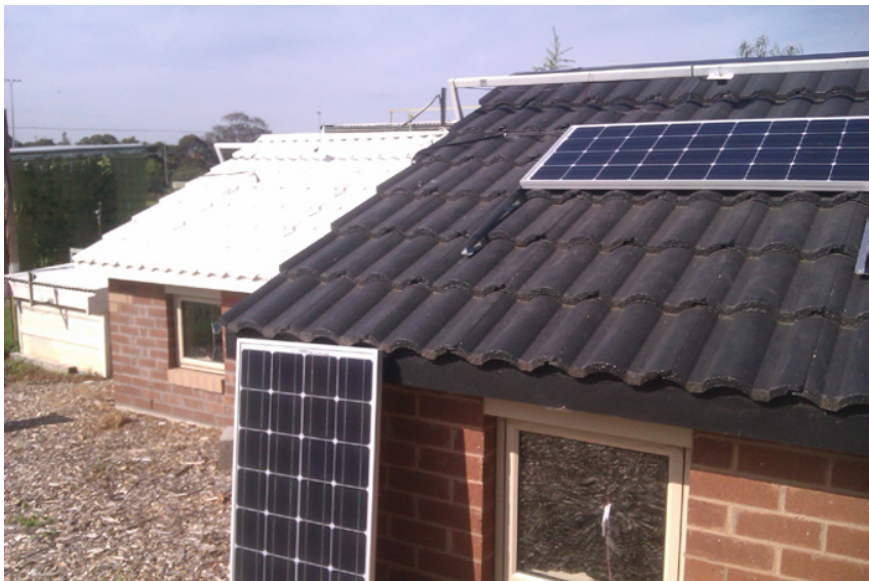
Figure 11.16 Buildings J and H, and test PV panels.
