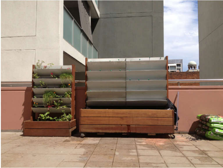
Figure 9.6 V Gardens on level 5 roof.
