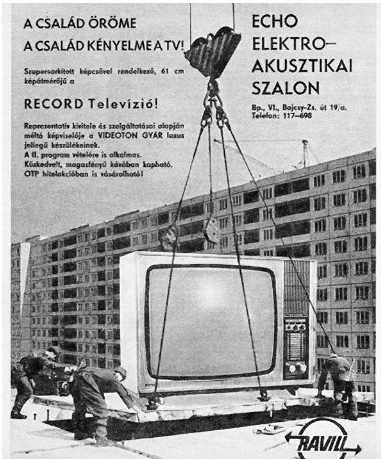
Figure 3.1. Advertisement for the new Videoton television set, circa 1970, with a television replacing the concrete panel on a construction site. “The family’s happiness, the family’s comfort: The TV!” http://retronom.hu/node/6967 . Accessed April 30, 2012.
