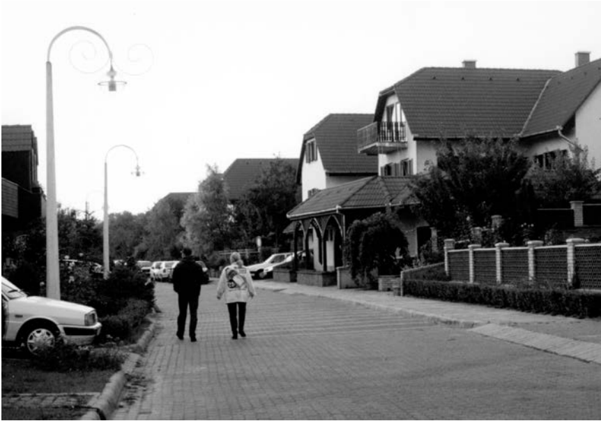
Figure 5.3. Late 1980s, cooperative, self-built housing development in Dunaújváros.
