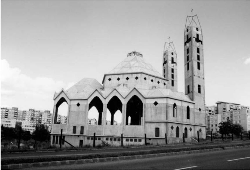
Figure 1.3. Catholic cathedral under construction in 1996, made of concrete panels and steel and designed by an architect trained in Hungarian Organicist school principles. Photo by Matthew Hull.
