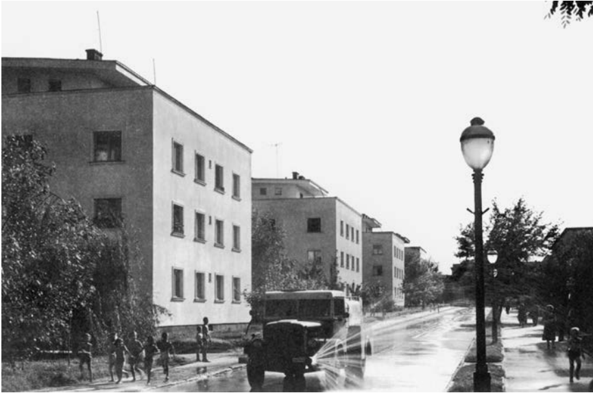
Figure 2.3. Modernist, free-standing housing cubes from the early 1950s. Photo used by permission of the Intercisa Museum, Dunaújváros.
