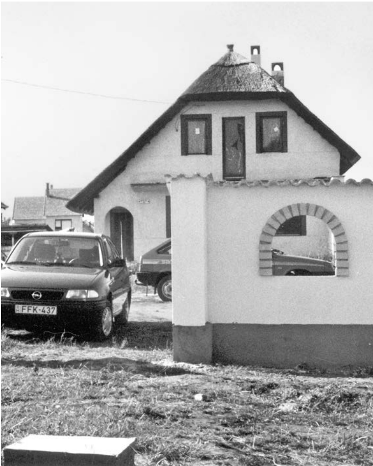
Figure 7.3. New houses under construction in suburbanizing village near Dunaújváros. The house shown has the mark of professional labor and sports a trendy thatched roof. Next door, a family is building a “square house,” a much simpler form of construction, and park their Trabant out front. These house forms and cars exemplify the gulf between new suburban residents. Photo by author, 1997.
