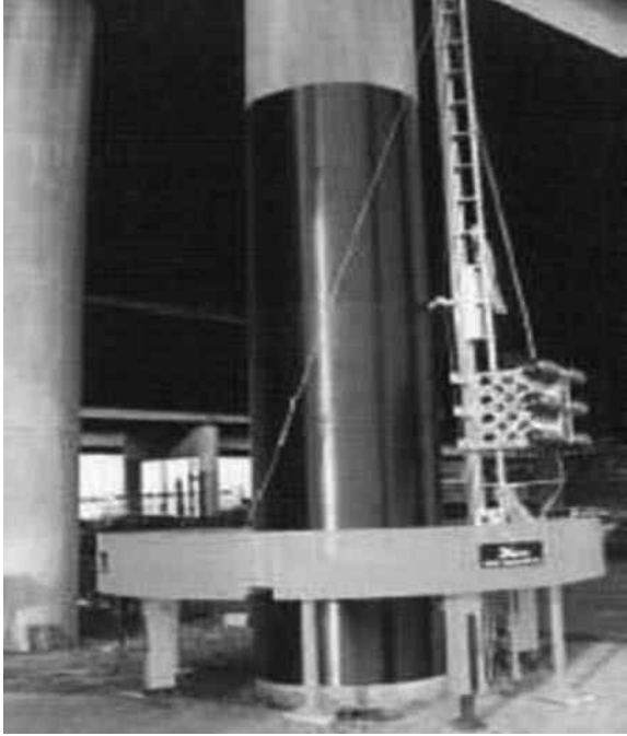
7.13 In situ strengthening of columns (The ROBO Wrapper I™).
