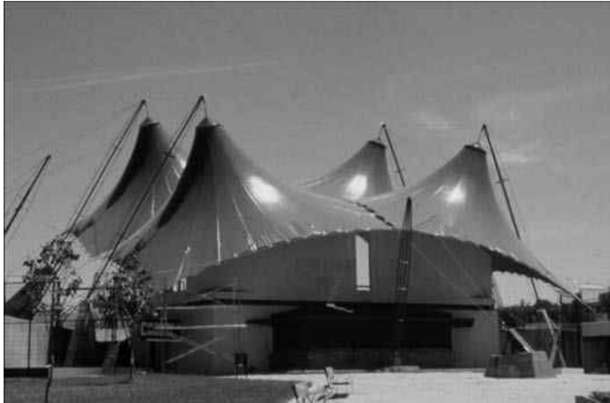
12.26 External masts to hang the fabric directly.
