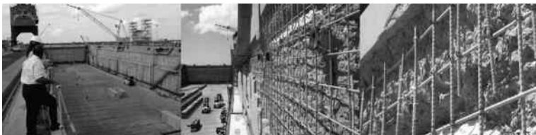
8.16 Pearl Harbor, dock rehabilitation ( http://www.hughesbros.com ).
