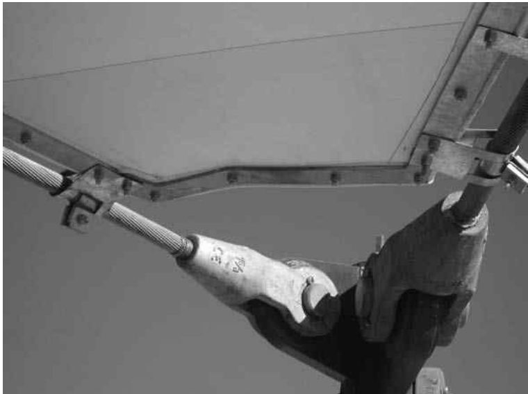
12.61 Repairing works needed after lifting process (CC Almenara, Lorca. BAT, Spain).
