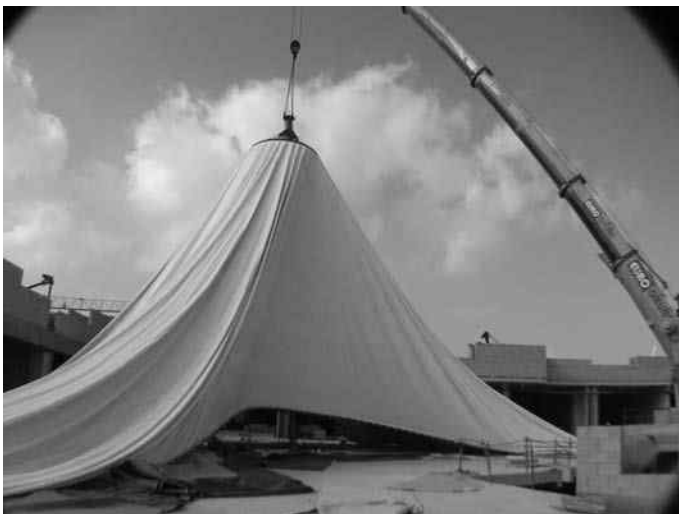
12.59 Lifting the membrane (CC Almenara, Lorca. BAT, Spain).
