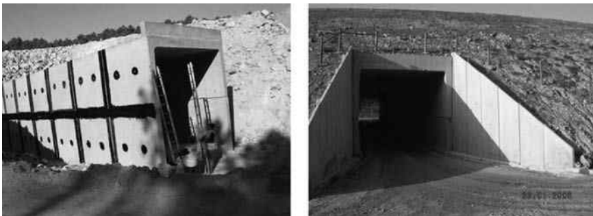
4.38 Examples of application of a box culvert.
