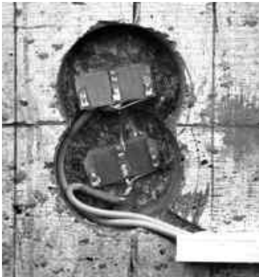
9.7 The ER probes installation on existing structure elements (Škedenj viaduct).
