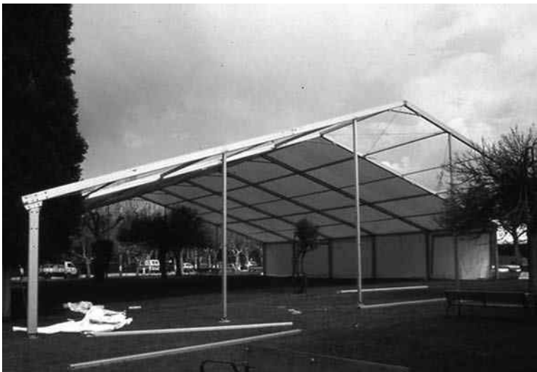
12.22 Internal portal frames.
