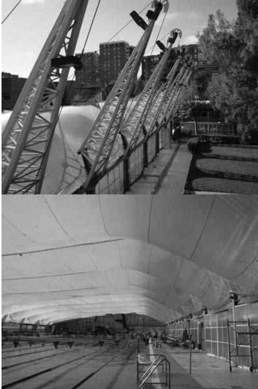
12.19 Swimming pool with external structure.
