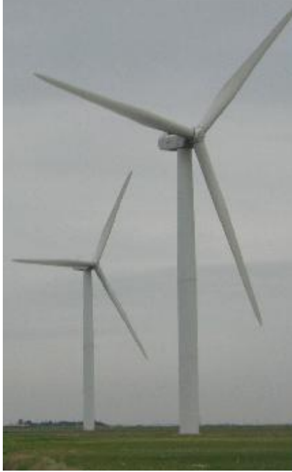
Figure 4.42. Doubly-fed induction machine wind turbine (parc de Bouin, Vendée, France). 2.5 MW, 660 V machines. The three-bladed turbine has a diameter of 80 m, and its speed is between 11 and 19 rpm. The generator rotation speed is near 1,500 rpm. The induction machine is connected to the blades by a mechanical device multiplying the speed
