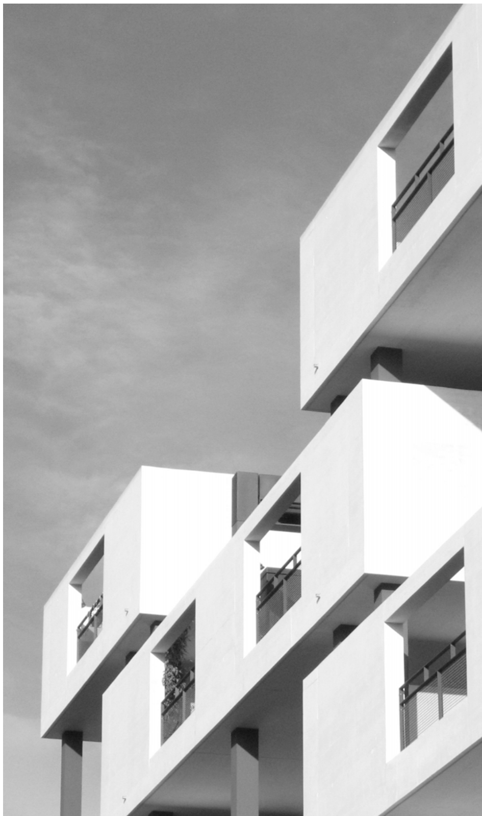
Paul-Clairmont-Straße multi-storey housing, Zurich, 2006, Gmür & Steib Architekten
