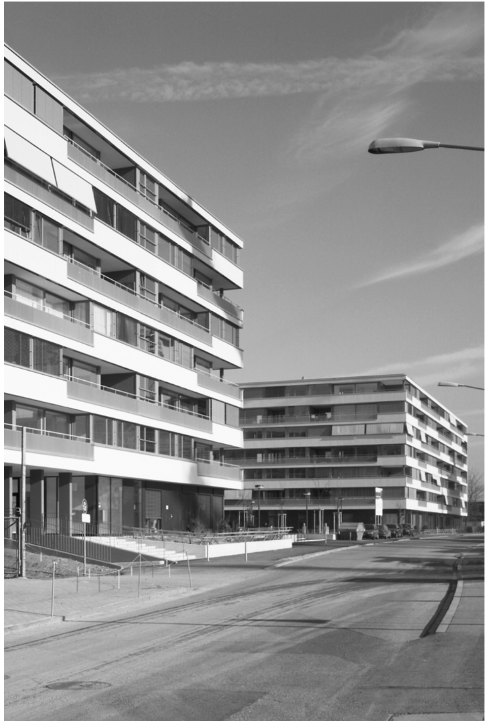
Aspholz-Nord residential housing Zurich, 2005 pool Architekten
