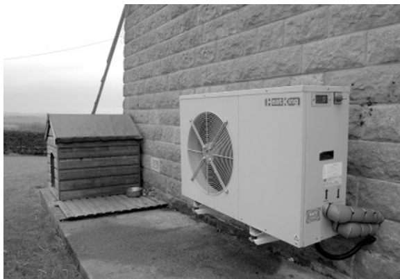
Figure 27.4 Wall mounted ASHP delivering 8 kW heating to a farmhouse in Appleton le street, North Yorkshire (HeatKing)
