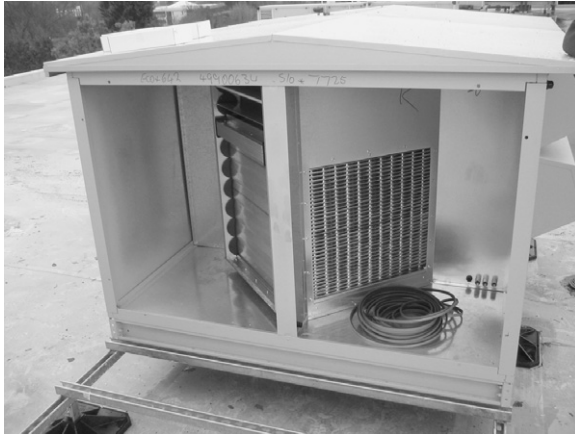
Figure 23.4 Air-to-air heat exchanger (Business Edge)
