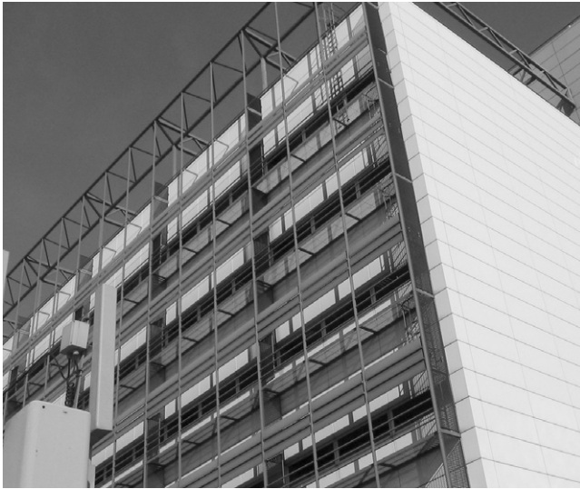
Figure 23.2 Solar shading (Business Edge)
