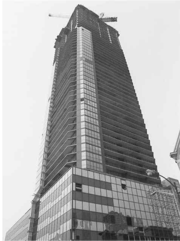
Office building under construction, Chicago, Illinois.
