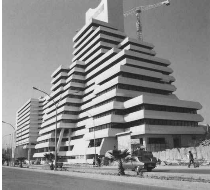
Reinforced concrete office building, Amman, Jordan.
