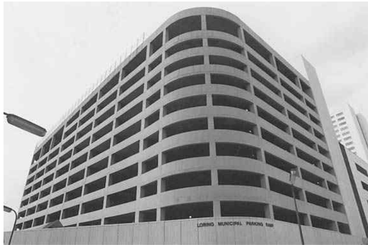
Reinforced concrete parking structure, Minneapolis, Minnesota.
