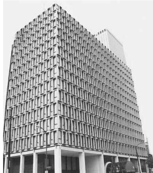
Office building, Chicago, Illinois.
