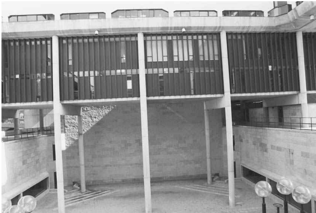
Columns, University of Wisconsin, Madison, Wisconsin.
