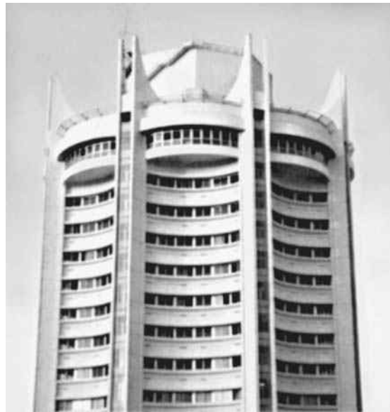
Circular beams in an office building.
