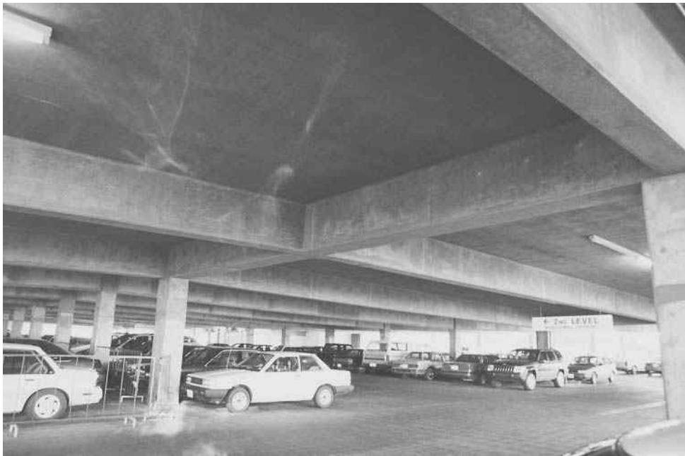
Slab on beams.
