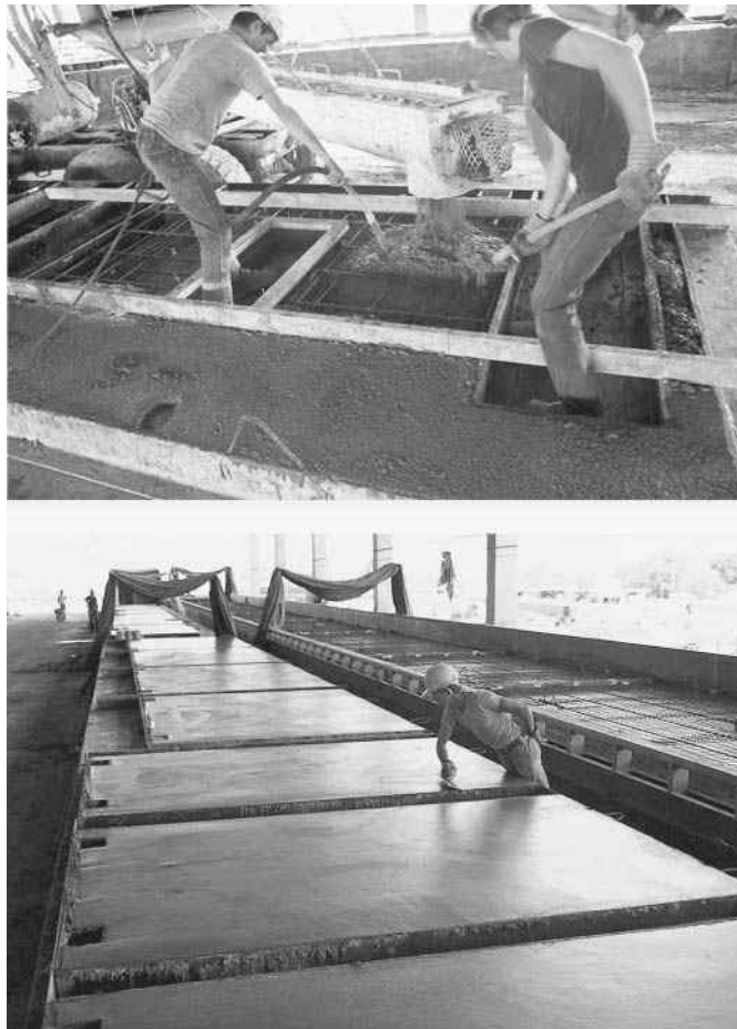
Casting and finishing precast concrete wall panels.
