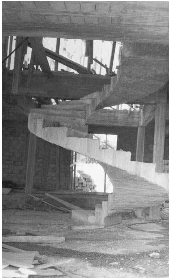
Reinforced concrete helical staircase.
