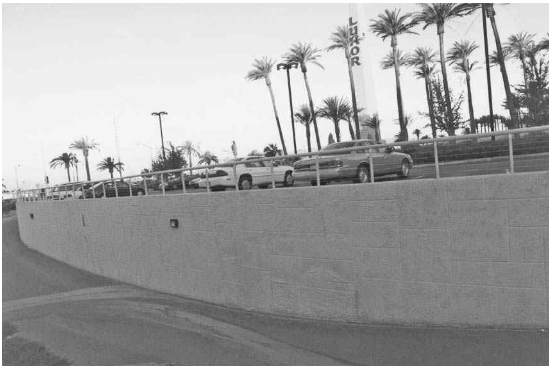
Retaining wall in a parking area.
