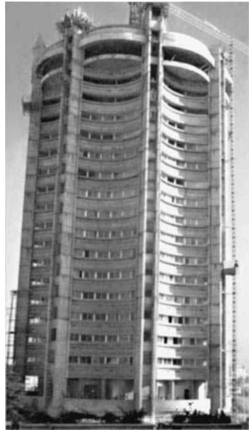
Curved beams in an office building.
