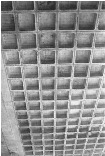
Waffle slab (looking upward).
