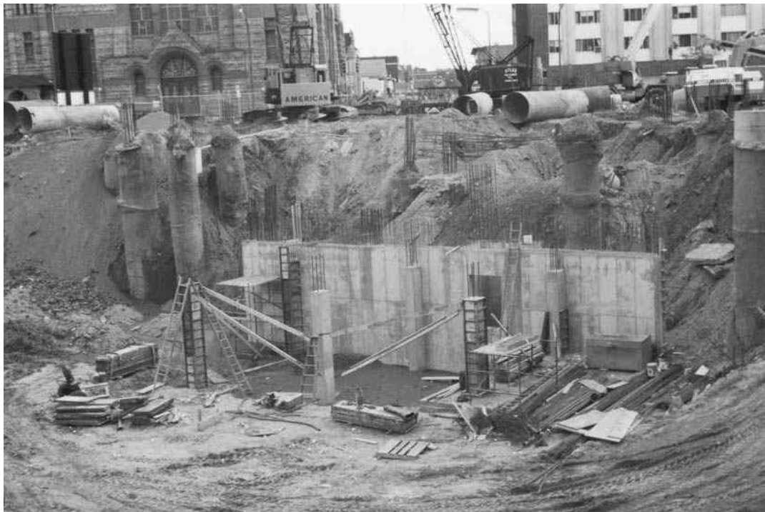
Wall and column footings, partly covered.
