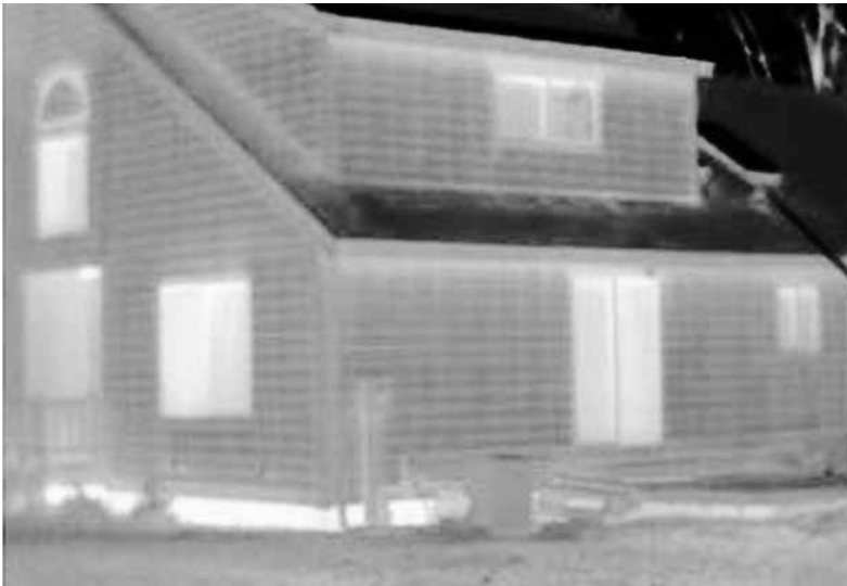
FIGURE 4.3. This thermal image shows heat loss through poorly insulated areas of the home. Credit: The Renewables RouteMap Team, The Scotland Government, UK.
