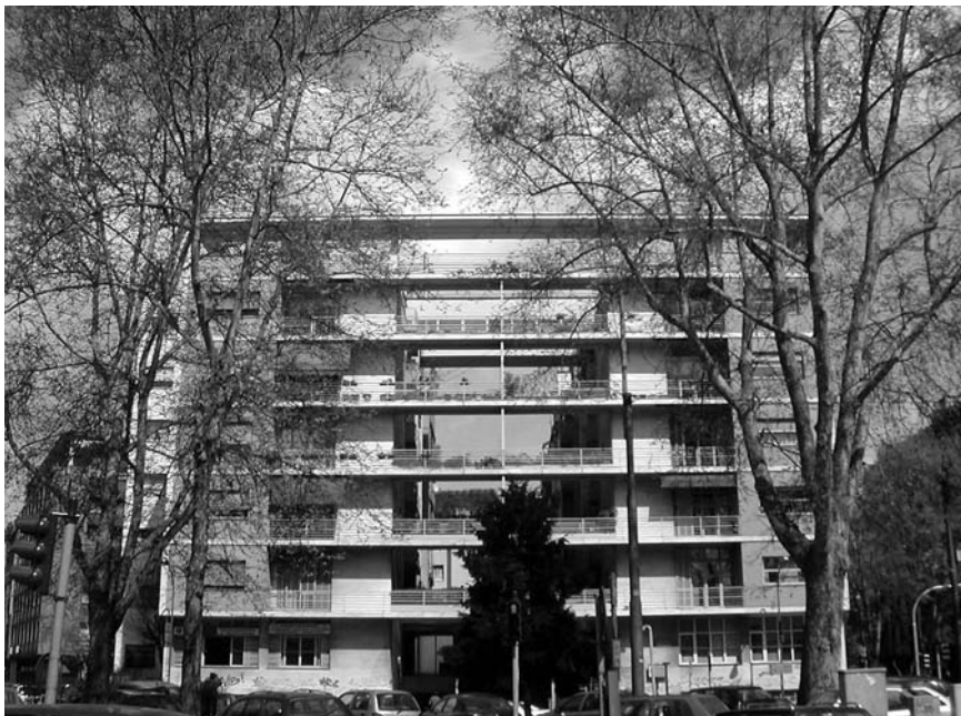
Casa Rustici, Milan. A poetic approach to modern apartment building design on Corso Sempione by Lingeri and Terragni (1933–1936).
