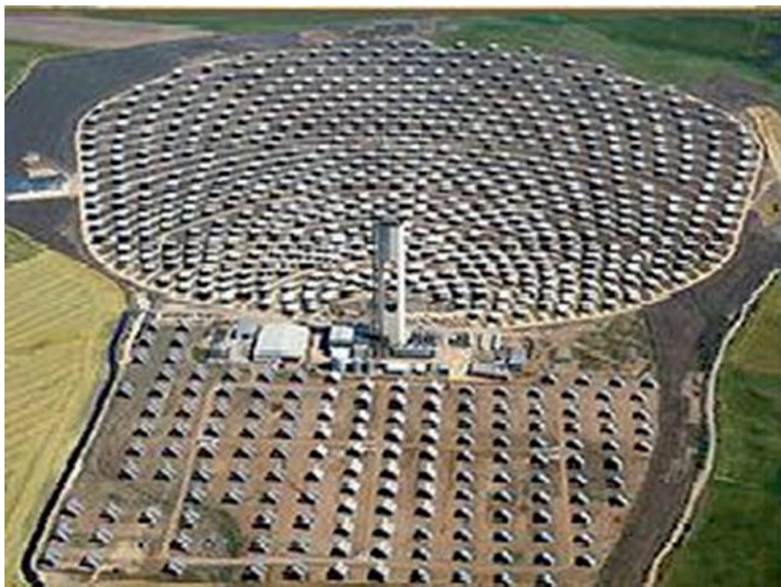
Fig. 4.18 Europe's first commercial CSP plant (11 MW) was inaugurated near the sunny Southern Spanish city of Seville. Source Photograph courtesy Abengoa
