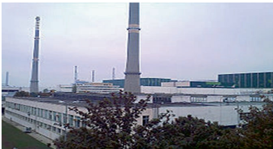
Fig. 8.17 Kozloduy nuclear power plant. Source Photograph courtesy of Wikipedia (Courtesy Ивайло Борисов)
