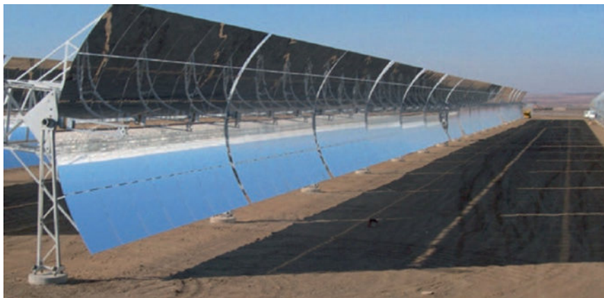
Fig. 4.2 Solar collector elements of a parabolic trough system. Source Concentrating solar power from research to implementation, European Commission
