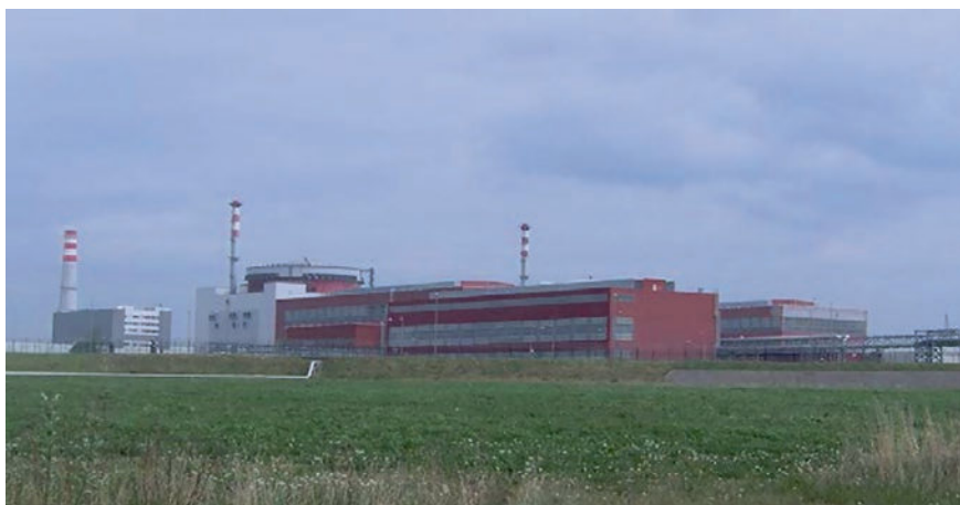
Fig. 8.48 Temelin nuclear power plant. Source Photograph courtesy of Wikipedia (User: Japo)
