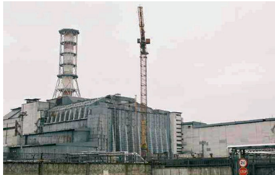
Fig. 8.39 Chernobyl nuclear power plant with the sarcophagus. Source Photograph courtesy of Wikimedia Commons (Elena Filatova)
