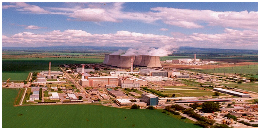
Fig. 8.29 Bohunice nuclear power plant. Source Photograph courtesy of IAEA
