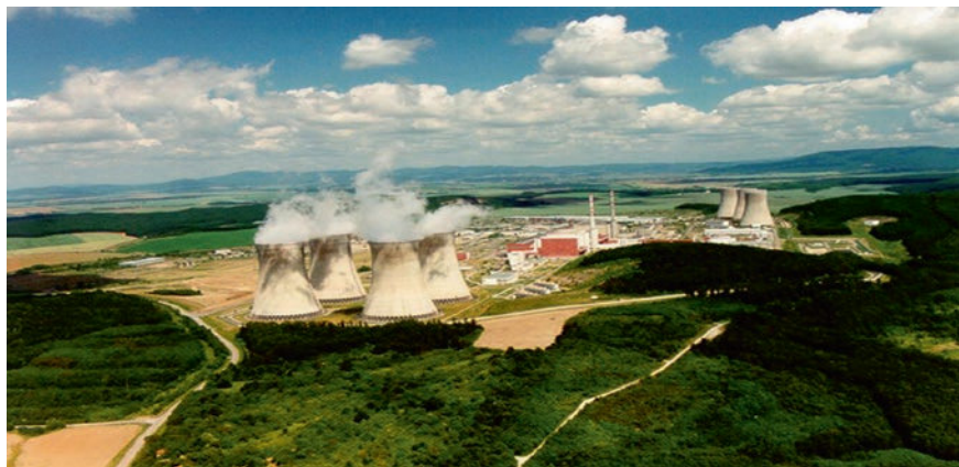
Fig. 8.28 Mochovce nuclear power plant. Source Photograph courtesy of the IAEA
