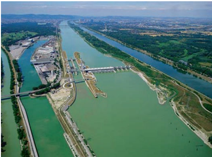
Fig. 3.3 Freudenau run-of-river power plant in Austria (a low-head run-of-river power plant). Source Verbund
