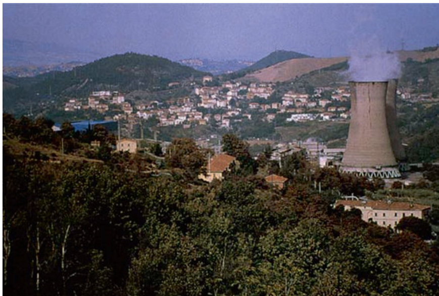
Fig. 6.7 The first modern geothermal power plants were also built in Lardello, Italy. Source Geothermal Education Office
