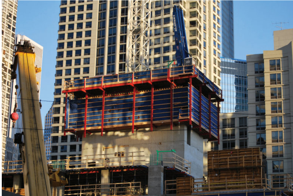
Figure 12-3 Climbing forms result in more efficient construction.
