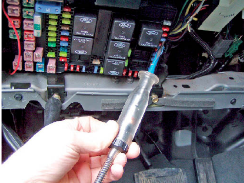
A seriously large fuse board in a new American monster.
