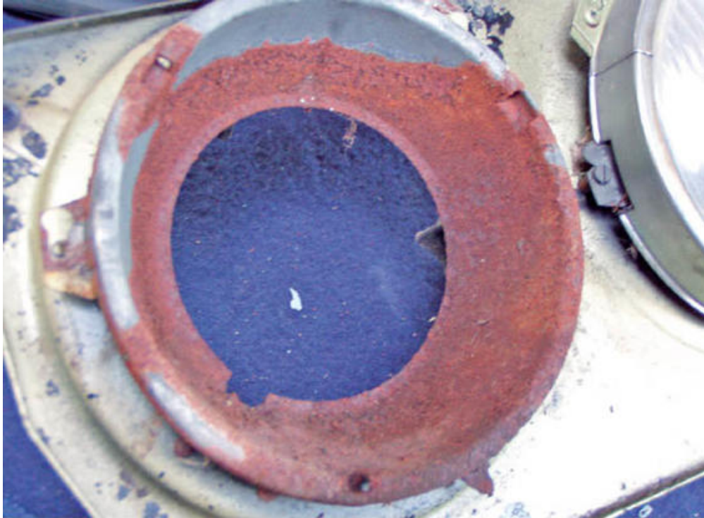
Rusty lamp holders benefit from a coat of red oxide primer.
