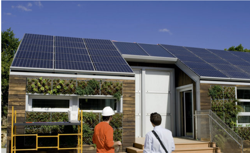
Figure 2.4 PV system in a domestic situation.
