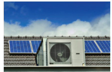
Figure 2.3 Solar photovoltaic (PV)
