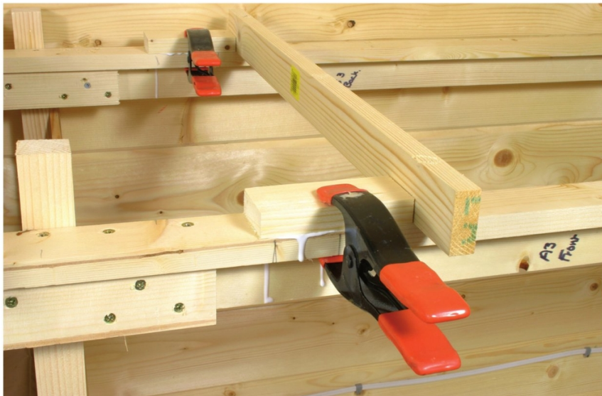
Belt and braces: another block of wood on the top of the girders and that join is never going to move.
