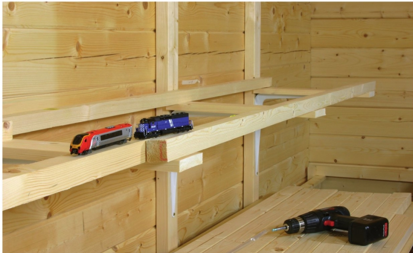
A view of the long girders during construction. The N scale models seen in this shot offer a perspective on the additional space and running length that the shelf layout and second deck concepts offer layout designers.
