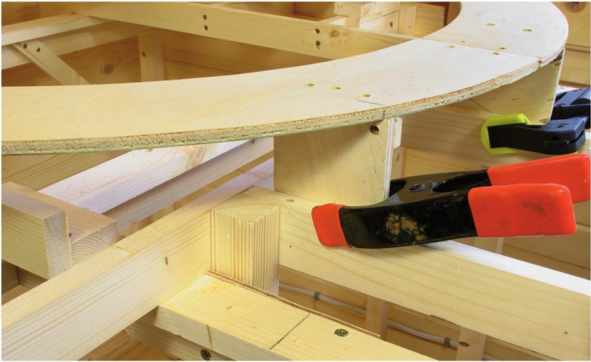
Clamping each riser and segment subassembly to the joists before committing to a more permanent fixing allows for adjustments to be made to the gradient.
