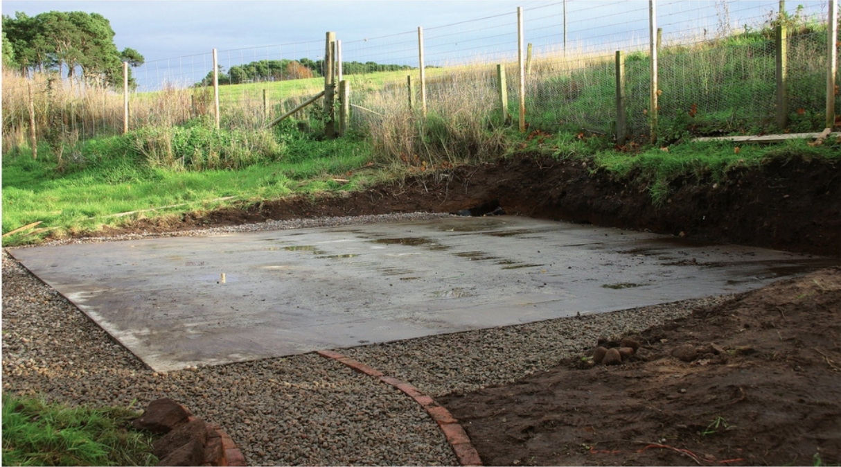
Finding a home: the start of my grand project was marked by the ground works for the cabin base, which was composed of a slab of concrete 100mm thick placed on a prepared base of aggregate, sand and a water-bar membrane.
