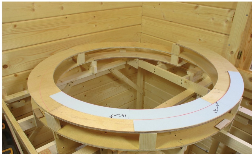
This view shows the risers and blocks used to achieve the second turn of the helix.
