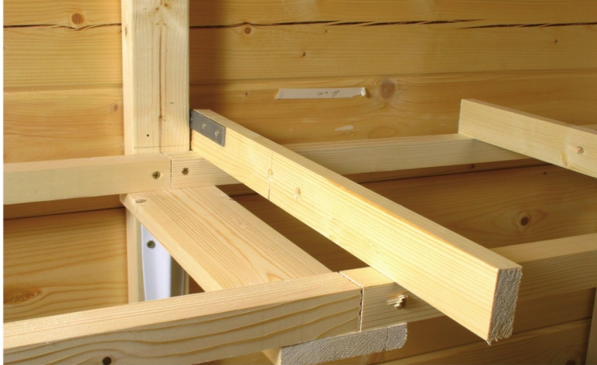
Each joist fitted over the shelving brackets is fitted with a steel angle plate for additional rigidity.
