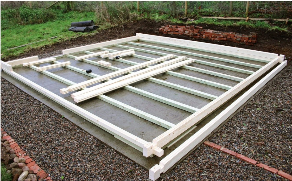
The cabin base is seen placed on the slab and squared off. Note the gravel around the concrete slab for drainage.
