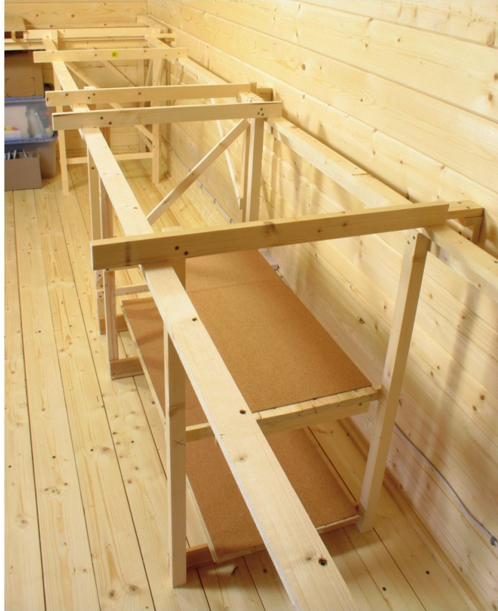
Three spans of L-girder were used along the side wall, the fourth, smaller baseboard frame being of a different size and shape to support the helix.
