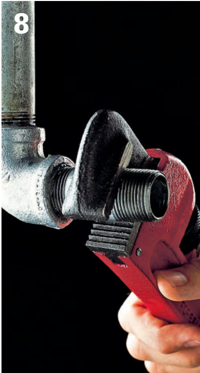
8 Screw the first nipple into the fitting, and tighten with a pipe wrench.
