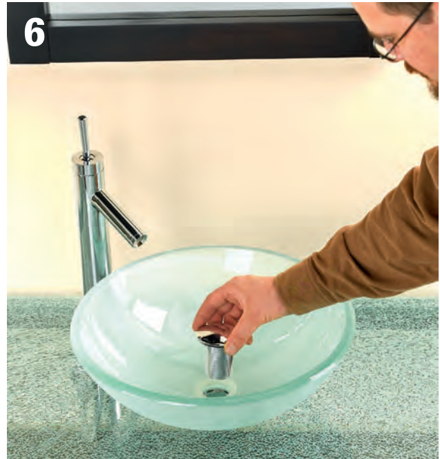
6 Put the small rubber gasket over the drain hole in the vessel. From the top, push the pop-up assembly through the drain hole.
