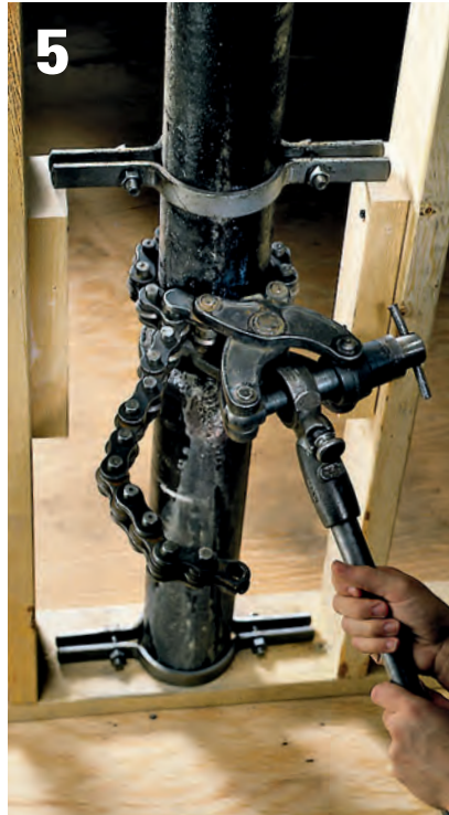
5 Tighten the chain and snap the pipe according to the tool manufacturer's directions.
