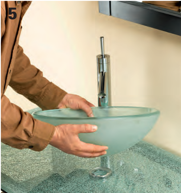
5 Place the vessel bowl on top of the O-rings. In this installation, the vessel is not bonded to the countertop.
