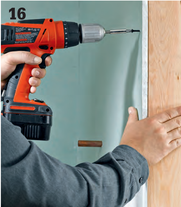
16 Install wallcovering material above the enclosure panels and anywhere else it is needed. Use moisture-resistant materials, and maintain a gap of \frac{1}{4} " between the shoulders of the top panel flanges and the wallcovering.
