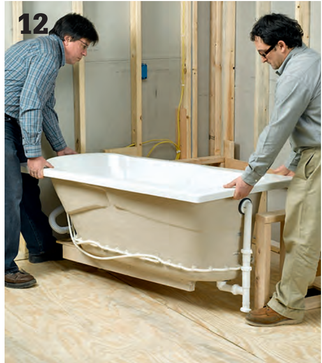
Slide or lower the tub into the installation area , taking care not to disturb the drain/overflow assembly. Make sure the drain tailpiece aligns exactly over the P-trap opening.
