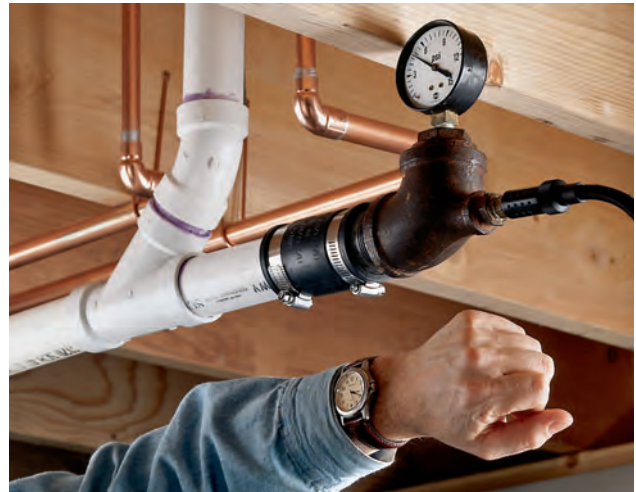
A pressure gauge and air pump are used to test DWV lines. The system is first blocked off at each fixture and at points near where the new drain and vent pipes connect to the main stack. Air is then pumped into the system to a pressure of 5 pounds per square inch (psi). To pass inspection, the system must hold this pressure for 15 minutes.
