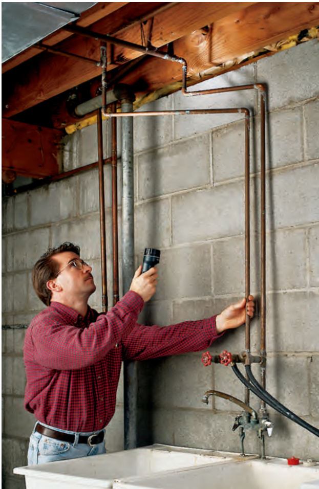
Snoop around your basement for clues about the locations of supply, drain, vent, and gas pipes in your walls.
