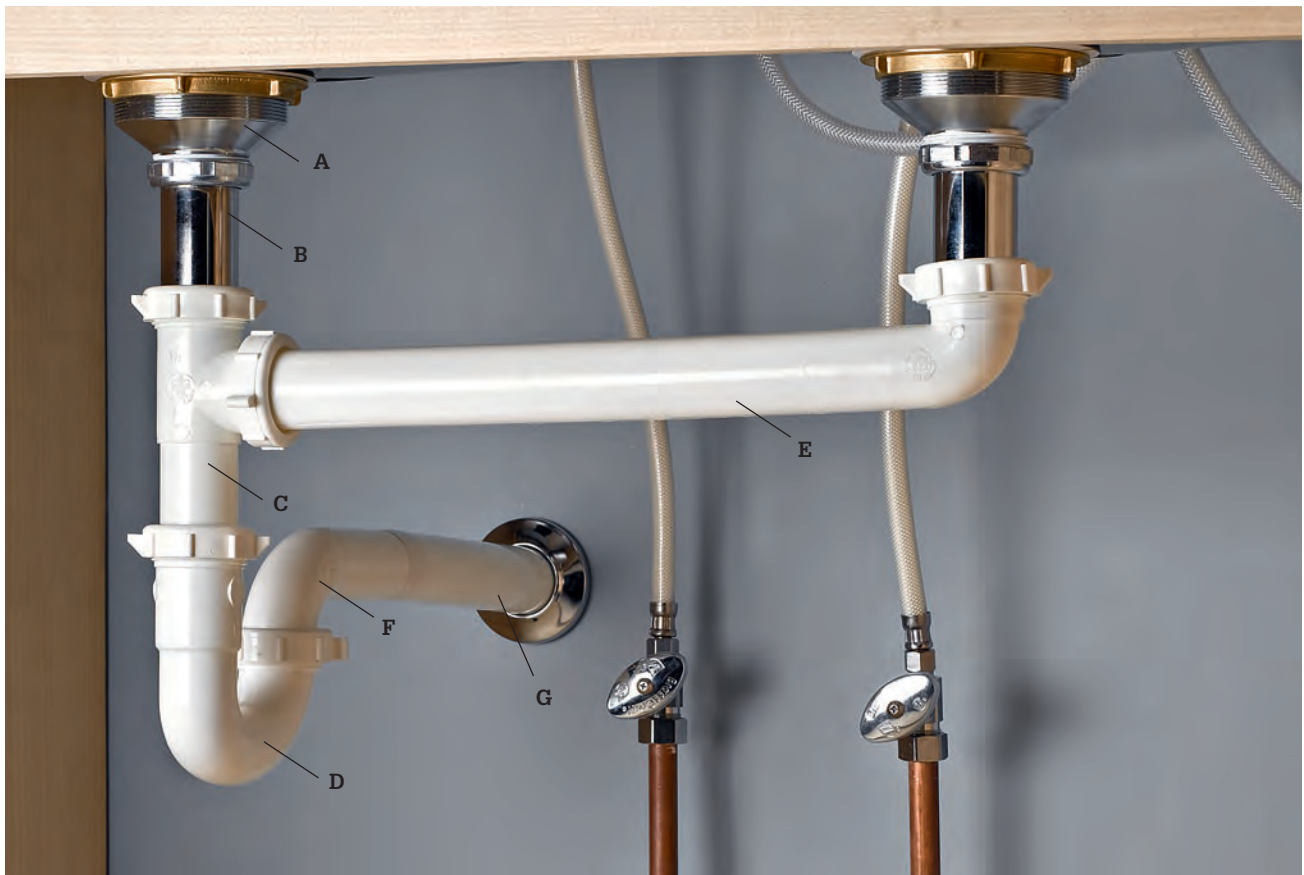
Kitchen sink drains include a strainer basket (A), tailpiece (B), continuous waste T (C), P- or S-trap (D), outlet drain lines (E), trap arm (F), and wall stubout (G).
