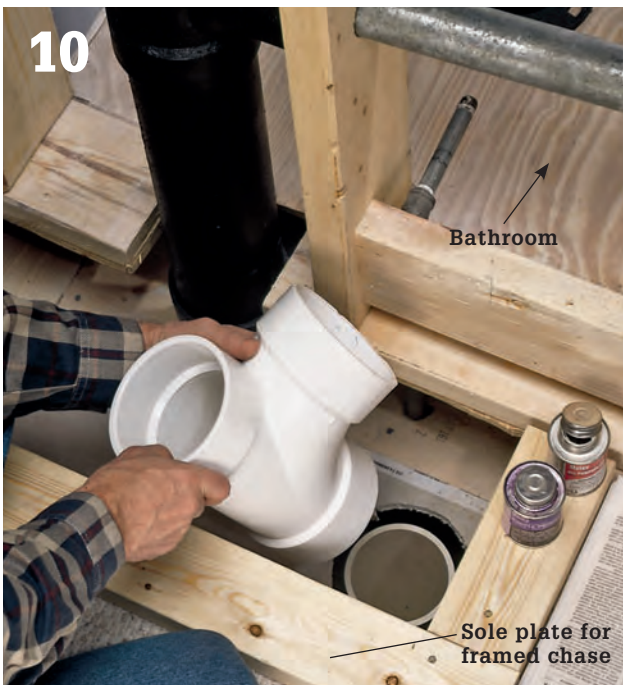
10 Attach the next waste T-fitting to the stack. In our demonstration project, the waste-T lay between floor joists and was used to connect the toilet drain. Make sure the waste-T is positioned at a height that will allow for the correct \frac{1}{4} " per ft. downward slope for the toilet drain.
