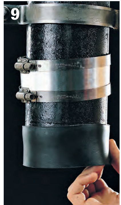
9 Make sure the cast-iron pipe is seated snugly against the rubber separator ring molded into the interior of the sleeve.
