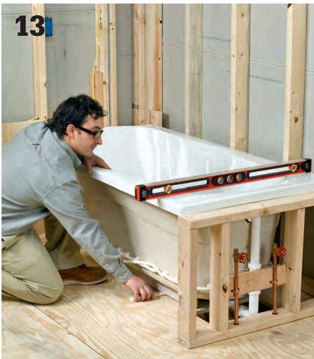
Check the tub for level. If it is not level, check to make sure it is resting cleanly on the subfloor all around. If needed, shim underneath one of the feet to level the tub. Do not shim under apron if your tub has one that is already installed.
