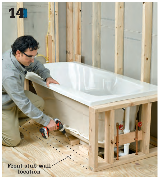
Secure the leveled tub in place as directed in your installation manual. Here, 2 × 4 block are screwed to the floor around the perimeter of the bathtub basin to create small curbs that prevent the tub from shifting. Build a 2 × 4 stub wall to support the front tub rim.
