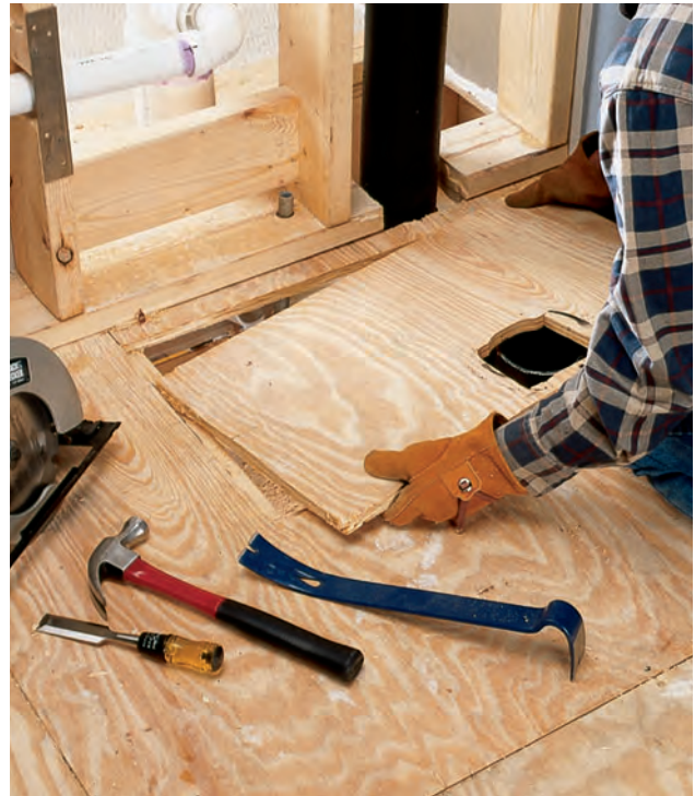
Replacing a toilet drain usually requires that you remove flooring and wall surface to gain access to the pipes.
