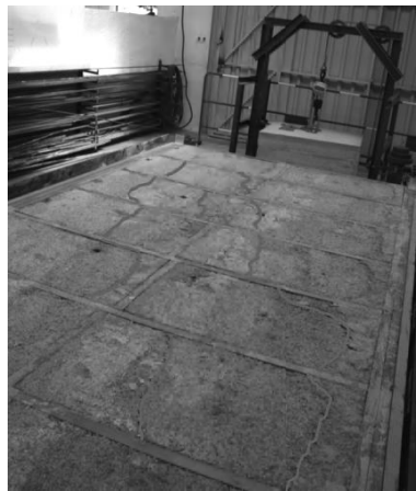
Figure 8.21. Cracking of the hempcrete at the end of the test (photo taken from the point of horizontal loading)
