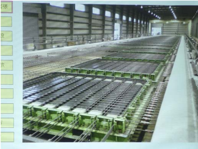
Figure 27.19 Installation of the pre-tensioned reinforcing system.
