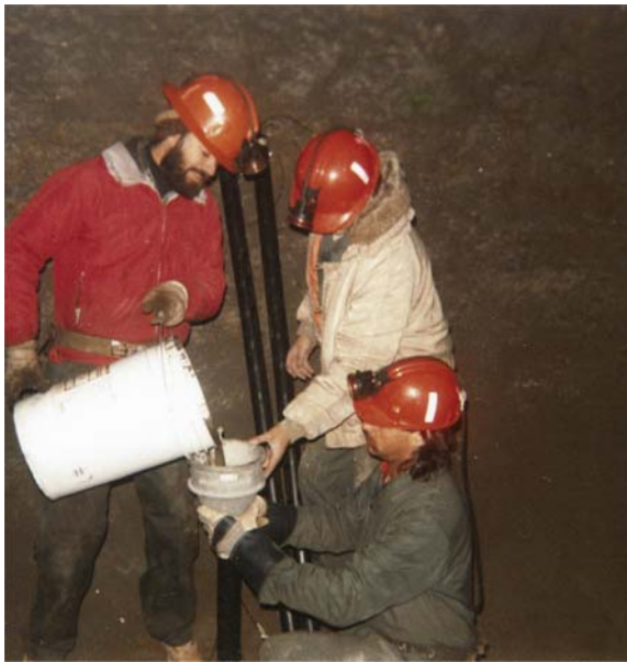
Figure 21.3 Grouting the anchors in the mine gallery.
