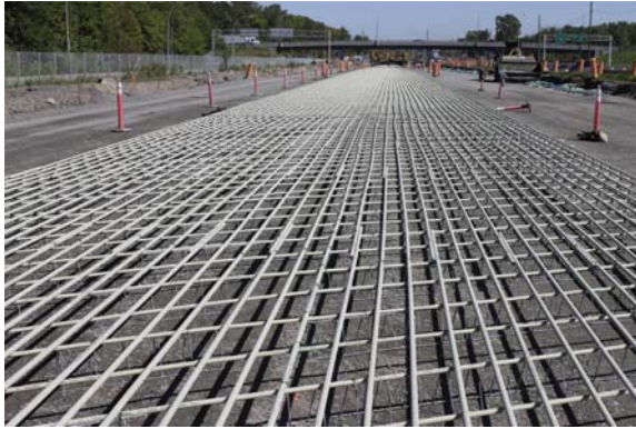
Figure 24.5 The use of glass fiber reinforced bars in a continuously reinforced pavement. Courtesy of Brahim Benmokrane.
