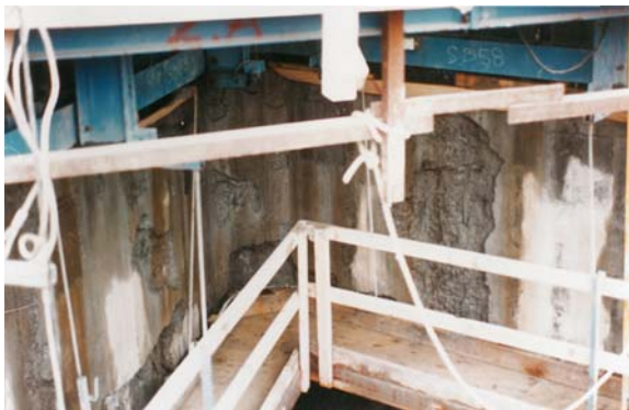
Figure 18.3 External surface of an offshore platform due to the fact that the slipforming occurred too late.
