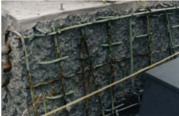
Figure 24.2 Example of the consequence of a very rough handling of epoxy-coated rebars. Courtesy of Daniel Vézina.
