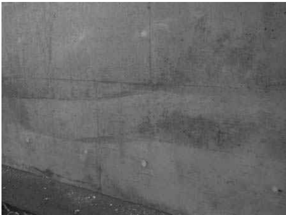
Figure 20.16 Retaining wall at Les Escoumins in Quebec.
