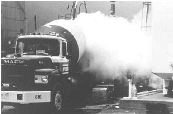
Figure 18.1 Cooling concrete with liquid nitrogen.
