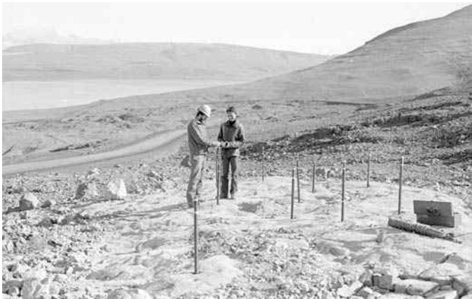
Figure 21.4 Installation of the 12 anchors.
