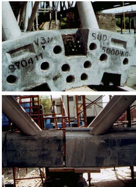
Figure 27.11 Assembling two prefabricated elements (dry joint).
