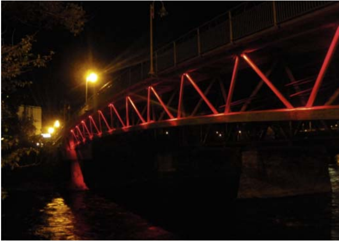
Figure 27.14 The Passerelle at night.
