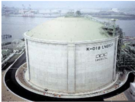
Figure 26.6 Finished 60 MPa post-tensioned concrete tank. With Courtesy of Osaka Gas CO., LTD.
