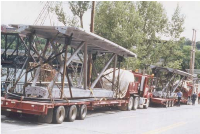
Figure 27.9 Transportation of the prefabricated elements.
