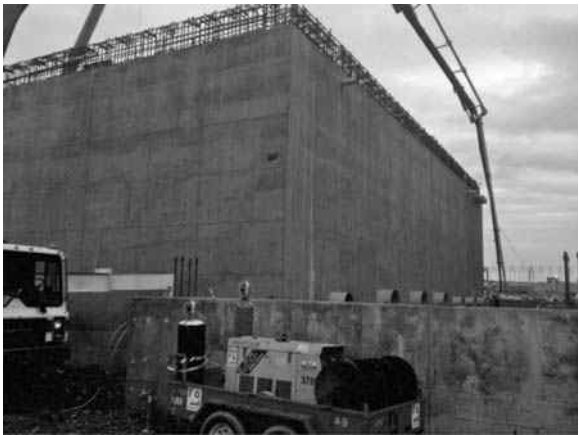
Figure 20.15 Construction of Fermont tank in Quebec using SSC1.
