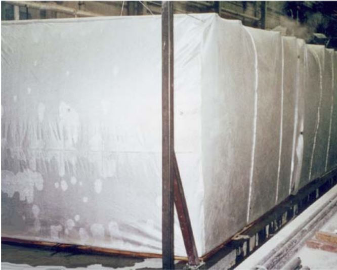
Figure 27.8 Curing of a pre-cast element.
