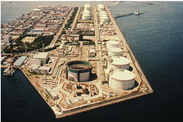
Figure 26.5 Construction of post-tensioned concrete LNG storage tank with a 60 MPa SCC in Senboku Terminal II in Osaka.
