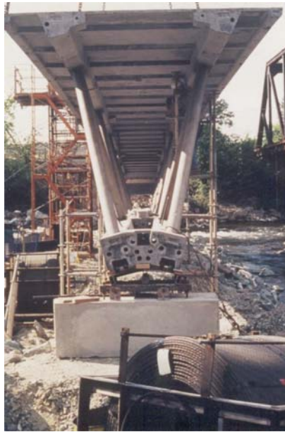
Figure 27.10 Assembling the northern part of the bridge.
