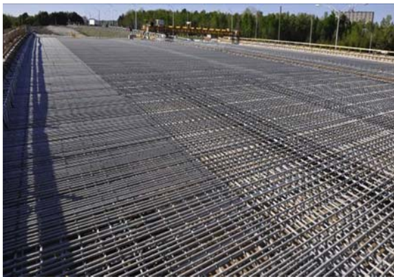
Figure 24.3 The use of glass fiber reinforced bars in a bridge deck. Courtesy of Daniel Vézina and Brahim Benmokrane.
