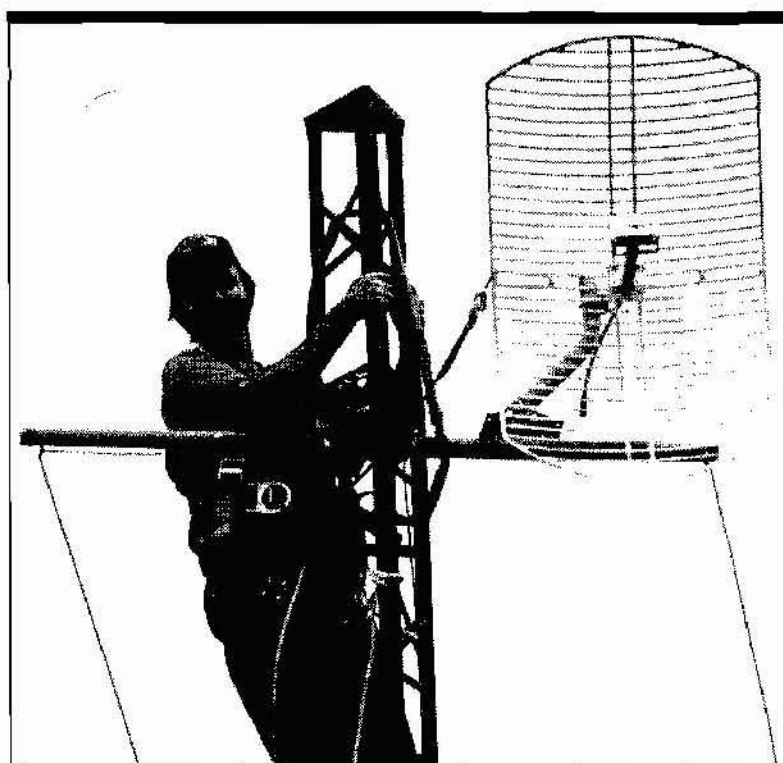
Daryl, KG4PRR, installs a microwave reflector array.
