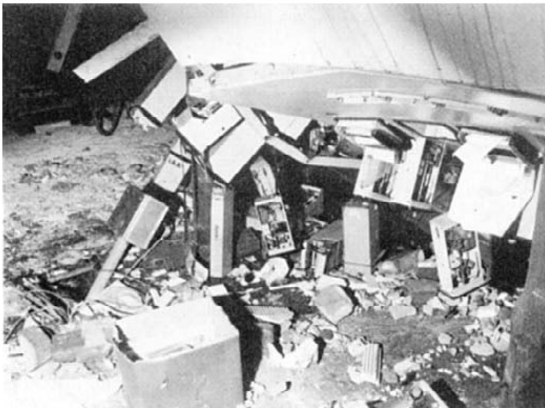
Figure A1.13 Beek, 1975: damage to instrumentation in the control room (Ministry of Social Affairs, 1976)
