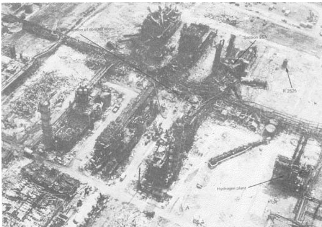
Figure A2.7 Works of Nypro (UK) Ltd at Flixborough after the explosion—2 (R.J. Parker, 1975) (Courtesy of HM Stationery Office)
