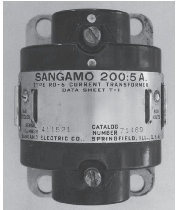
► Figure 3–14 Current transformer used to meter large AC currents. (Source: Delmar/Cengage Learning)
