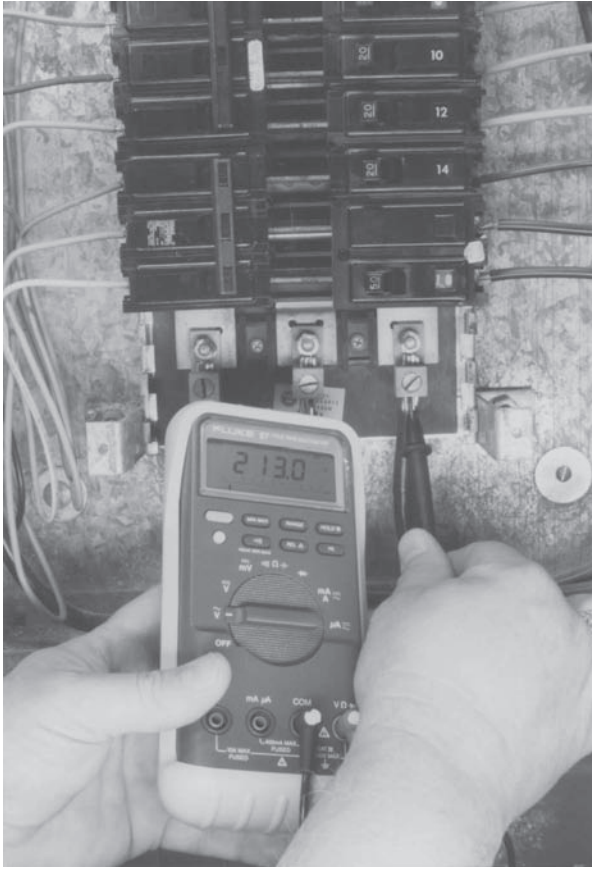
► Figure 3-1 Voltmeter being used to test the voltage of a panel. (Source: Delmar/Cengage Learning)
