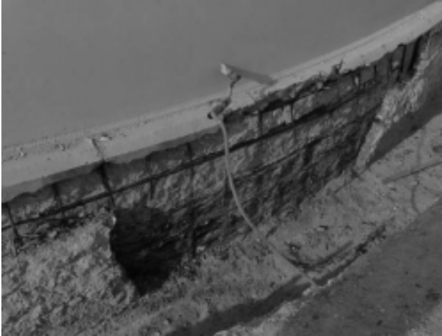
FIGURE 10.2 Removal of delaminated concrete from ring beam.
