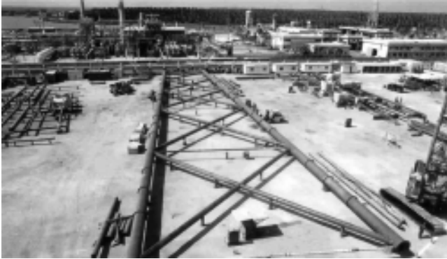
FIGURE 12.29 Jacket fabrication on the yard.
