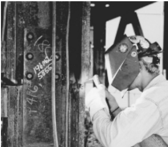
FIGURE 7.24 Welding in an existing building.
