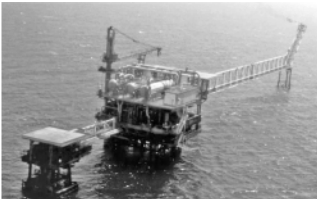
FIGURE 12.1 Production platform with bridges.
