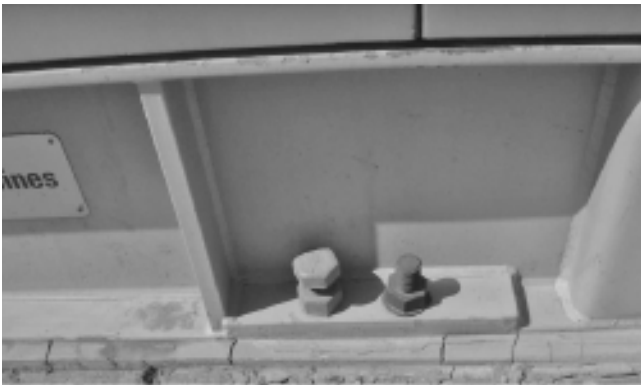
FIGURE 4.3 Fixing the skid to concrete.
