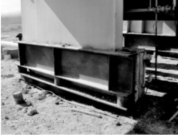
FIGURE 10.1 Temporary repair using steel sections.
