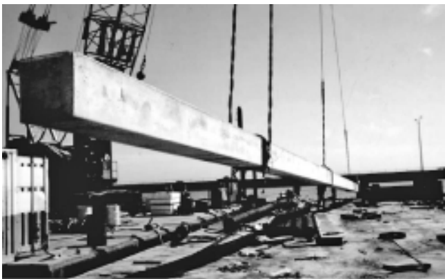
FIGURE 13.15 Lifting of the concrete pile.
