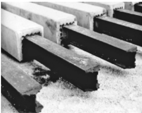
FIGURE 13.16 Composite section piles.
