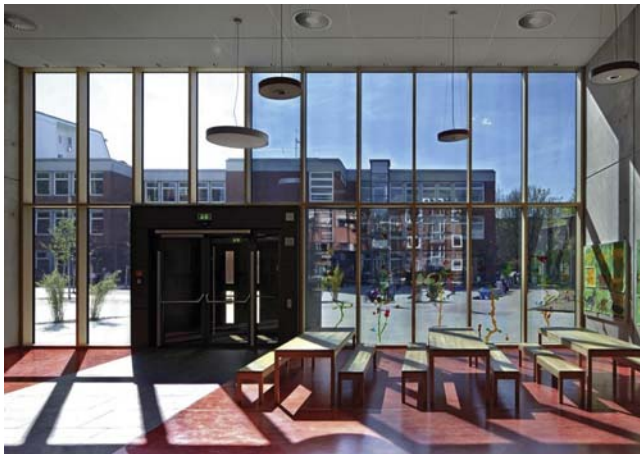
Figure 9.5 Electrochromic façade (half-tinted). Courtesy of EControl-Glas GmbH.
