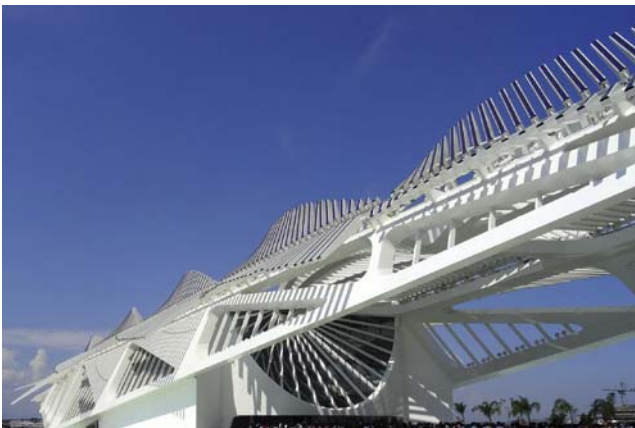
Figure 8.23 Museu do Amanhã, detail of PV-integrated movable roof components. Courtesy of Santiago Calatrava llc ©.
