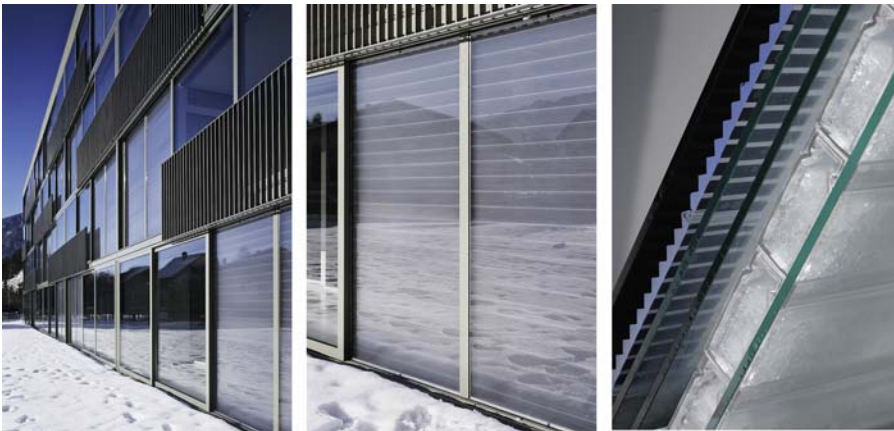
Figure 5.26 Retirement residence community, Schwarz Architekten, Domat Ems CH (left and center), and GlassX phase-change material glazing section (right). Courtesy of Gaston Wicky Photography ® and GlassX AG.
