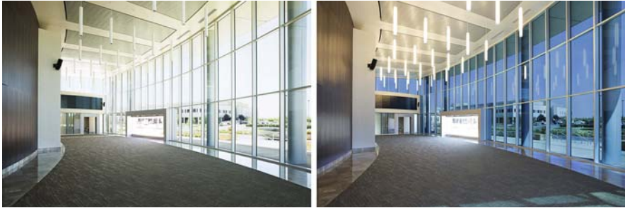
Figure 9.15 Electrochromic dynamic glazing control states. Courtesy of View Inc.
