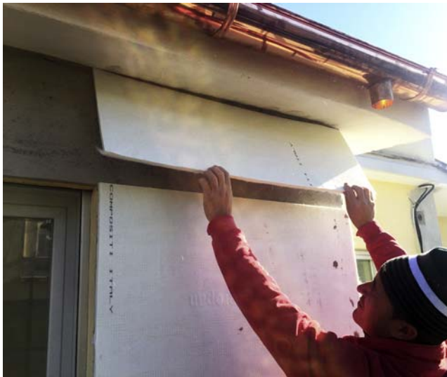
Figure 4.17 Aeropan installation.
