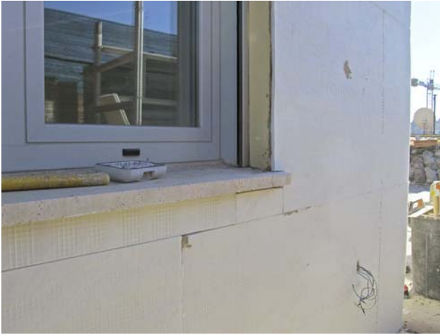
Figure 4.18 Installed Aeropan. Photo by the author.
