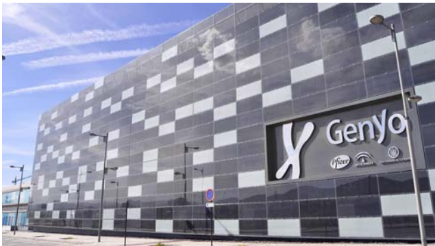
Figure 1.3 Semitransparent a-Si building-integrated photovoltaic facade, GenYo Center, Granada.
