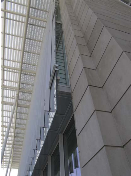
Figure 7.10 Glazed double-skin façade, exterior view, Chicago Art Institute, RPBW, Chicago. Photo by the author.
