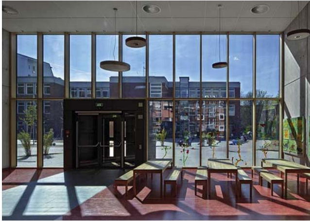
Figure 9.6 Electrochromic façade (fully tinted). Courtesy of EControl-Glas GmbH.
