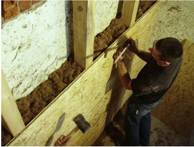
Figure 4.37 Algae-based insulation. Courtesy of Neptutherm GmbH.
