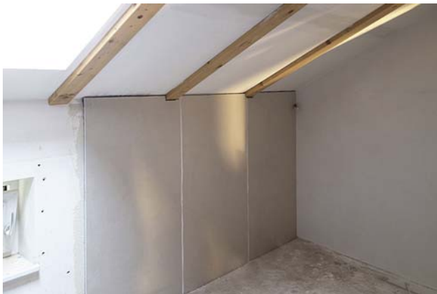
Figure 4.21 Installed Aerogips panels. Courtesy of AMA Composites s.r.l.
