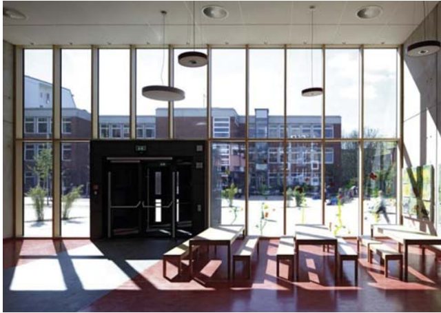
Figure 9.4 Electrochromic façade (clear). Courtesy of EControl-Glas GmbH.
