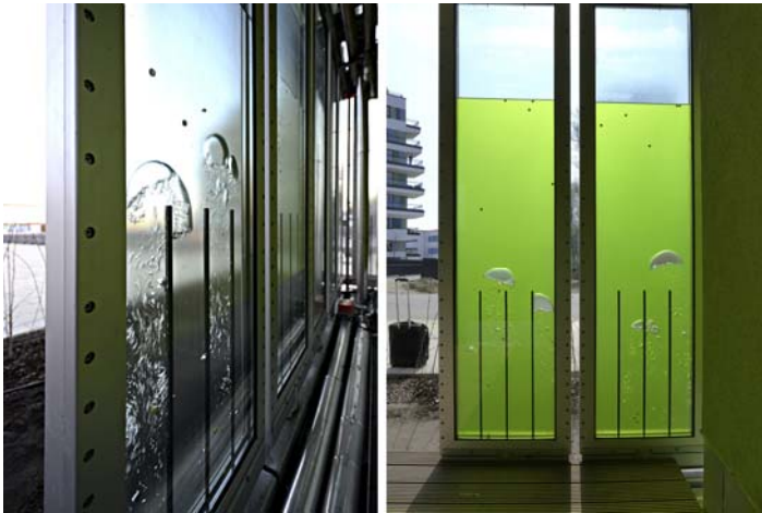
Figure 10.28 BIQ House algae reactors. Courtesy of Arup.
