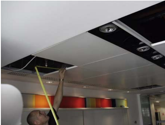
Figure 5.18 ThermaCool ceiling tile installation. Courtesy of Datum Phase Change Ltd.
