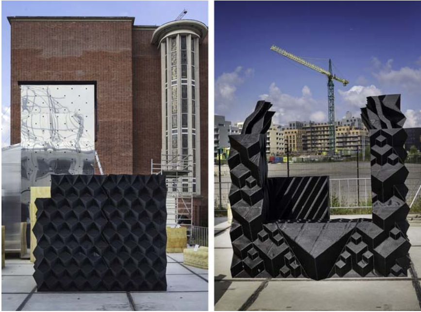
Figure 2.19 3D Print Canal House printed sections. Courtesy of Olivier Middendorp/Hollandse Hoogte ©.
