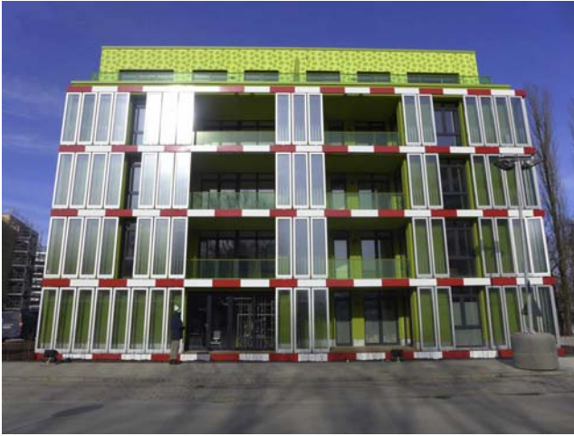
Figure 10.26 BIQ House, Arup, Hamburg. Courtesy of Arup.
