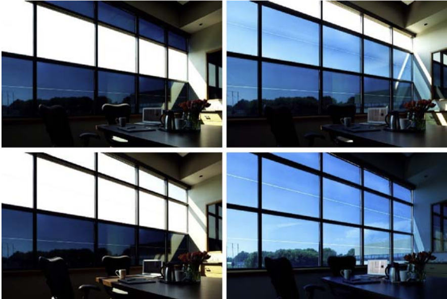
Figure 9.11 Electrochromic dynamic glass control states. Courtesy of Vetrotech Saint-Gobain International AG.
