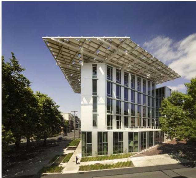
Figure 1.13 Bullitt Center, Miller Hull Partnership, Seattle. Courtesy of Nic Lehoux/Bullitt Foundation ©.
