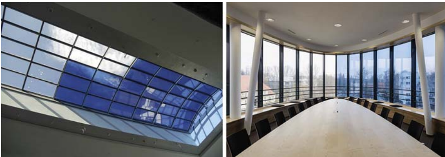
Figure 9.8 Electrochromic dynamic glazing. Courtesy of EControl-Glas GmbH.
