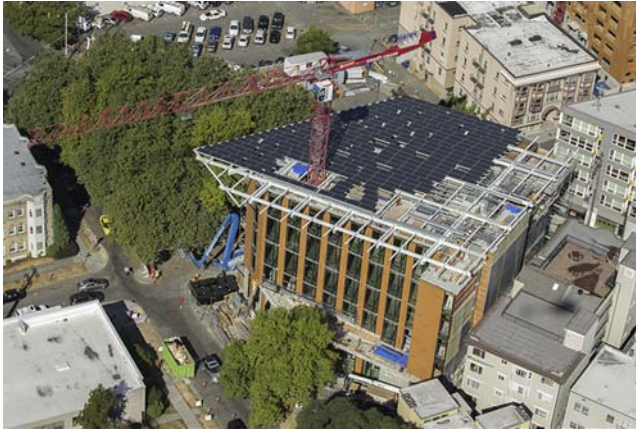
Figure 1.14 Bullitt Center, photovoltaic roof. Courtesy of John Stamets/Bullitt Foundation ©.
