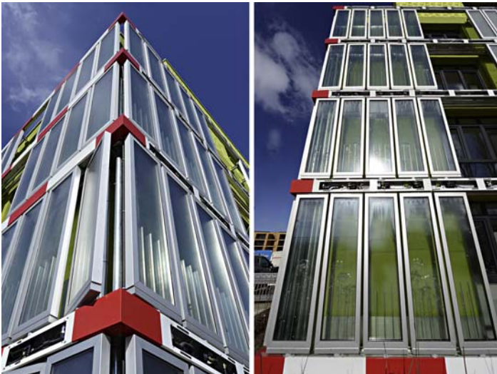
Figure 10.27 BIQ House bioadaptive facade. Courtesy of Arup.
