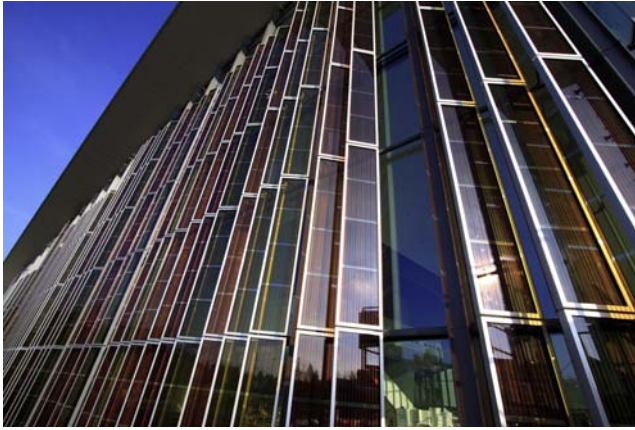
Figure 1.2 DSSC building-integrated photovoltaic facade, SwissTech Convention Center, Geneva.
