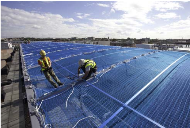
Figure 7.26 ETFE roof installation, King's Cross Station, London. Courtesy of John Sturrock/Vector Foiltec ©.
