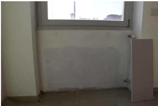
Figure 4.24 Window thermal bridge correction with Aerogips panels. Photo by the author.
