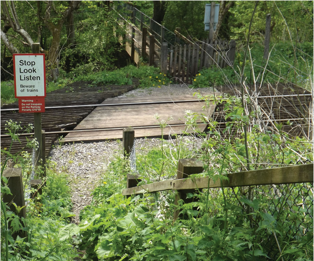
A crossing for a footpath, showing the wicket gate at the far side and the warning notice. There are also slatted wooden pieces on the sides of the crossing to prevent cattle from straying on the track.
