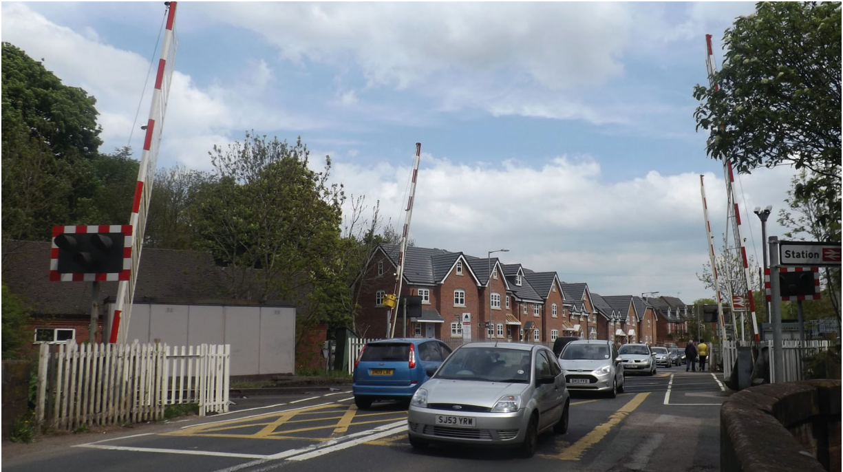
A CCTV camera can be seen above the direction sign to Blyth Bridge Station on the right hand side. This allows the signalman in his power box to check that the crossing is not blocked and the signals can be cleared for the trains to go through.
