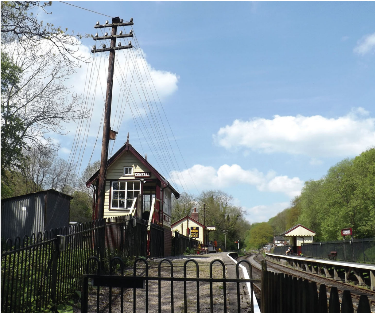
The railway had their own telegraph and later telephone system between signal boxes. Wires were also required for the block instruments to be interconnected between signal boxes.
