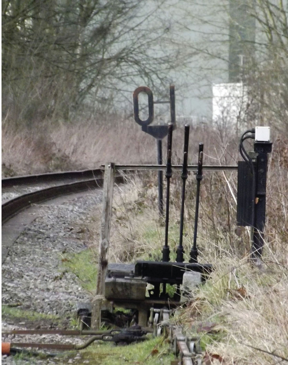
A ground frame with three levers for operating three points. The numbers in front are not part of the ground frame but are a speed limit for the engine driver.
