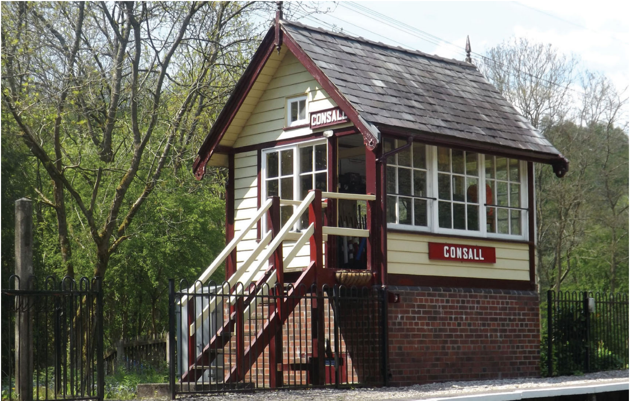
A small signal box positioned at the end of a station platform. On the upper floor, where the signal levers are, many windows were provided to give the signalmen a good view of what was going on. The interlocking equipment is located on the lower floor of the signal box.
