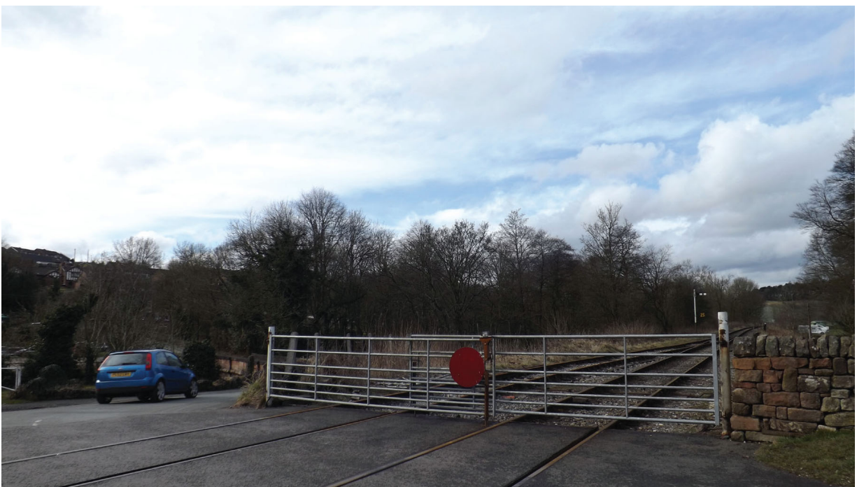
The crossing gates at Cheddleton Station, Staffordshire. Unlike a private road, the gates on this public road remain closed to trains when not in use. Note the characteristic red target shape on the gates, which overlap here as the road is wider than the railway tracks.
