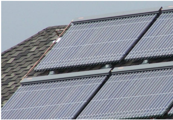
Figure 8.4. Vacuum tube collector.
