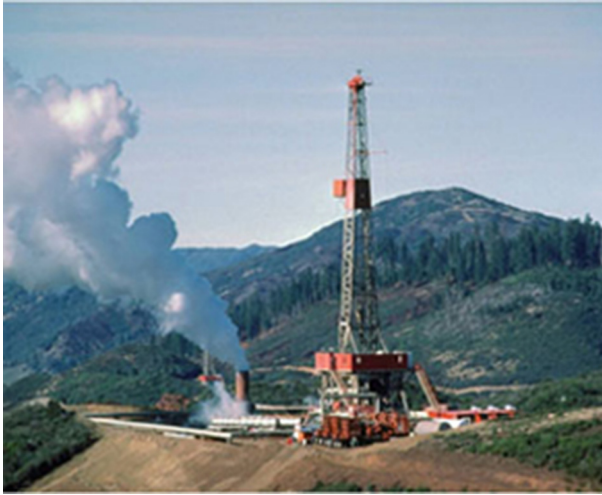
Figure 2.4. Geothermal plant. (Source: Courtesy of NREL.)
