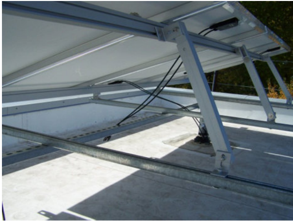
Figure 9.5. Tilt racking.
