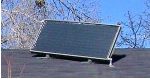
Figure 8.3. Flat-plate collector.
