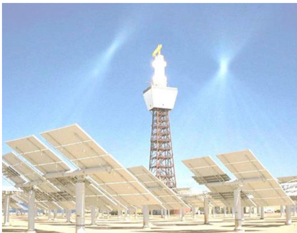
Figure 8.7. Solar thermal plant.
