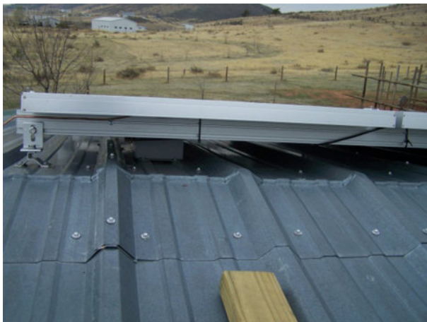
Figure 9.6. Roof-mount brackets.
