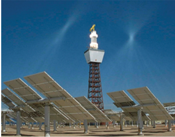
Figure 2.2. Solar thermal plant. (Source: Photo courtesy of NREL.)
