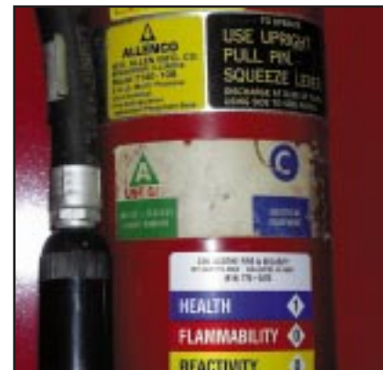
This extinguisher can only be used on Class A and Class C fires.
