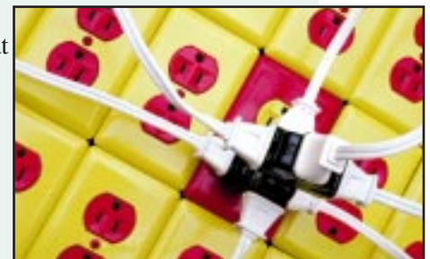
Overloads are a major cause of fires.
