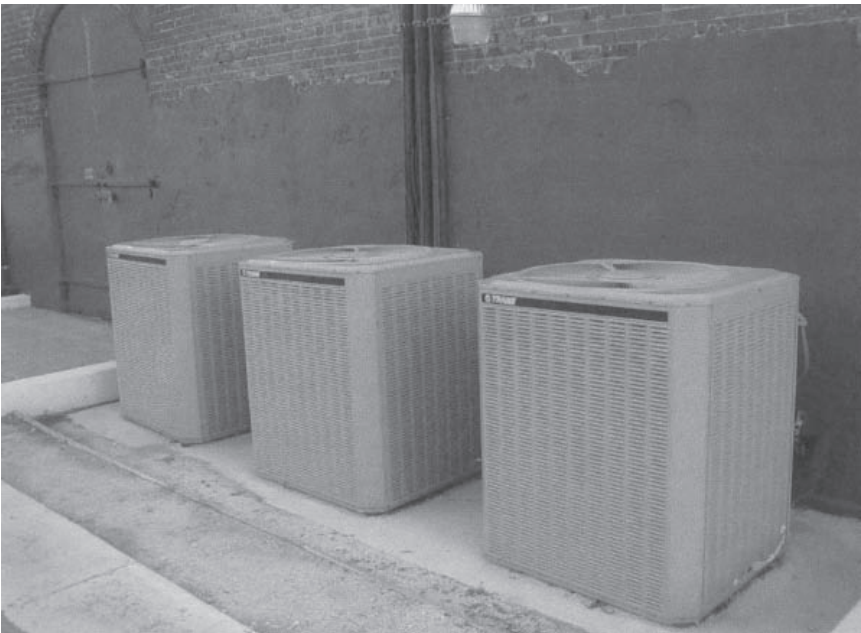
Figure 14-1. HVAC heat exchanger. Air-cooled condenser (refrigerant to air).
