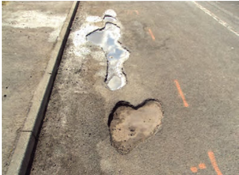
Figure 7.38 Potholes
