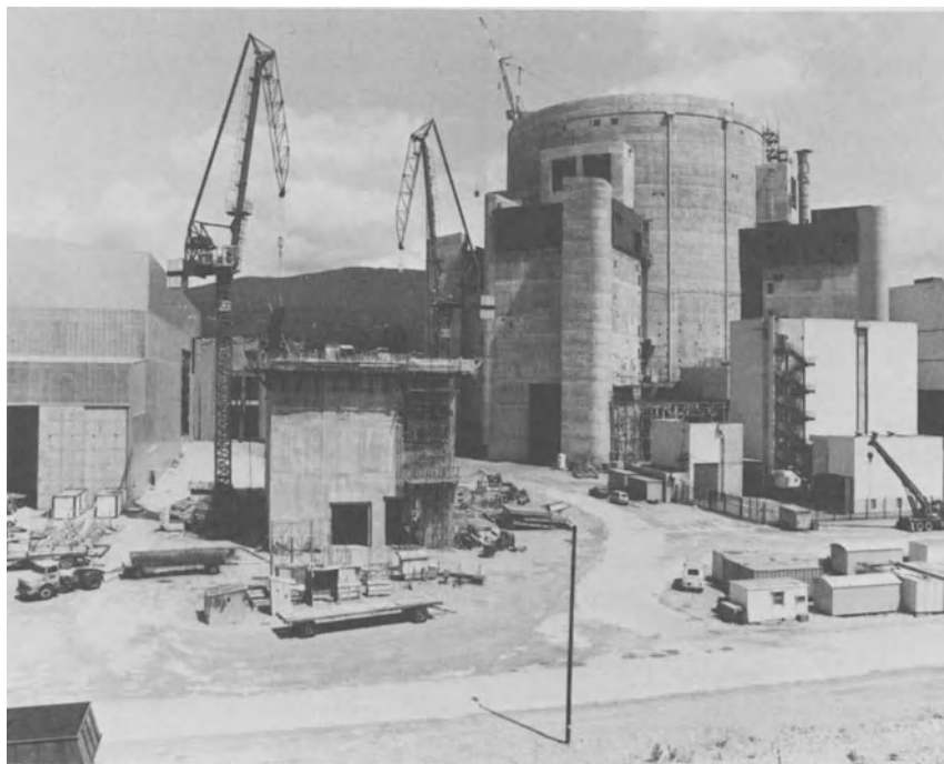
FIGURE 4. Super-Phenix: Creys-Malville site, reactor building, August 1982. (Courtesy Novatome.)
