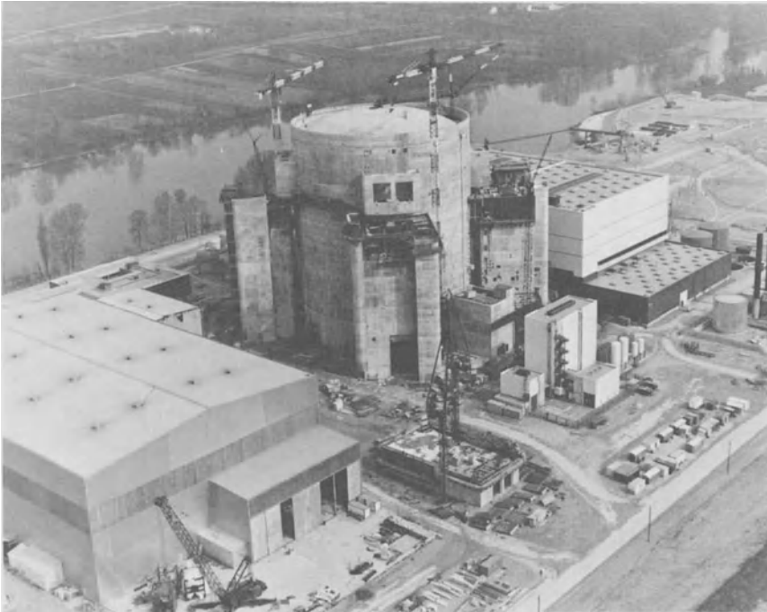
FIGURE 5. Super-Phenix: General views of the Creys-Malville site, April 1982. (Courtesy Novatome.)
