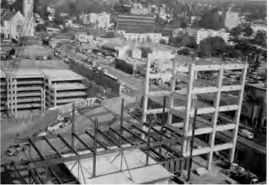
Photo 3.5 Precast DDC frame tower, Hollywood Highland Project, Hollywood CA. (Courtesy of Englekirk Partners, Inc.)
