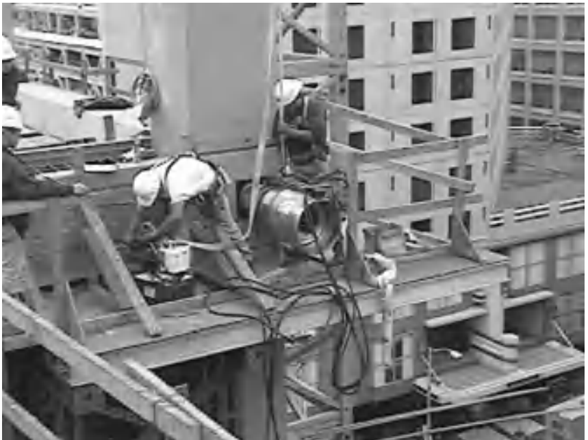
Photo 2.5 Preparing to stress a hybrid frame beam, Paramount Apartments, San Francisco, CA. (Courtesy of Charles Pankow Builders.)
