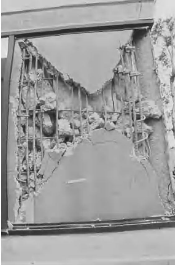
Photo 1.6 Overreinforced wall panel shear failure, Northridge earthquake, 1994. (Courtesy of Englekirk Partners, Inc.)
