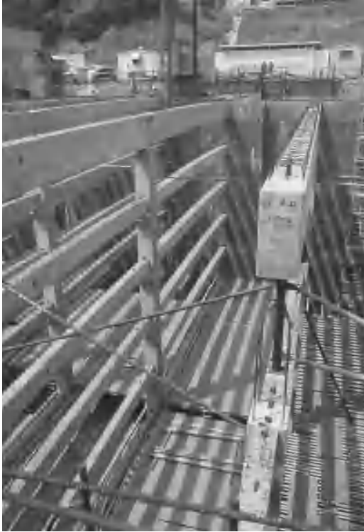
Photo 3.4 Nine-story precast concrete column, Getty Center Parking Structure, Brentwood, CA. (Courtesy of Englekirk Partners, Inc.)
