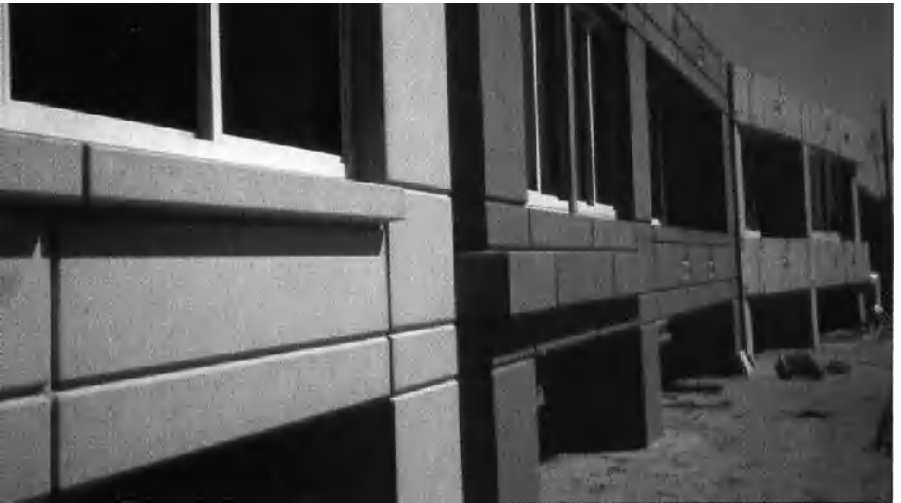
Figure 3.1.16 (Continued) Concrete finishes. Details incorporated into precast concrete frame beams. (Courtesy of Pankow Builders.)
