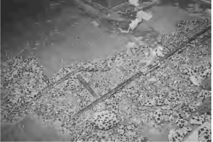
Photo 1.4 Flat slab with shear head shear failure, Northridge earthquake, 1994. (Courtesy of Englekirk Partners, Inc.)
