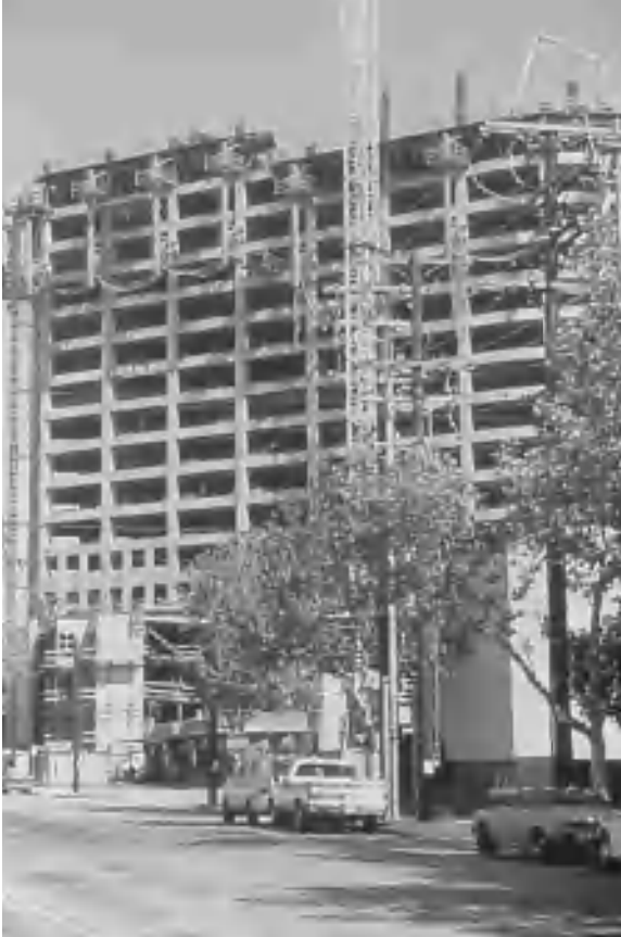
Photo 3.2 Cast-in-place concrete ductile frame construction, jump form framing. (Courtesy of Englekirk Partners, Inc.)
