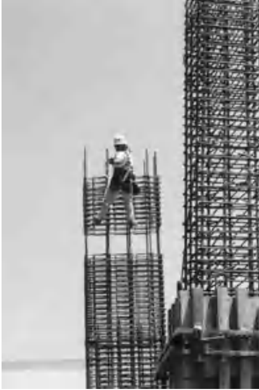
Photo 3.3 Placing a two-story column cage, The Remington, Westwood, CA. (Courtesy of Morley Construction Co.)
