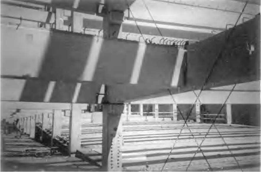
Figure 2.1.39 Precast framing for a composite system.
