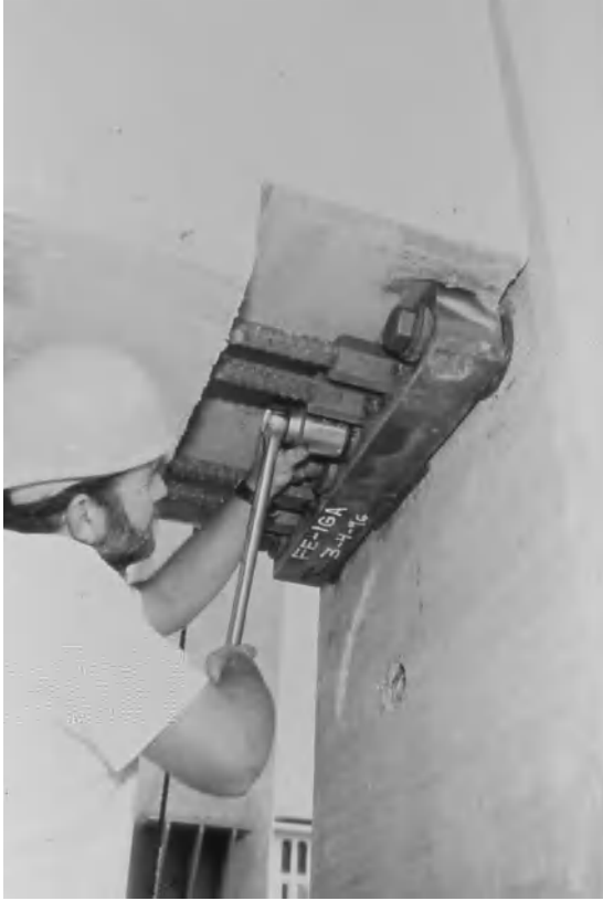
Photo 2.6 Assembling a DDC frame beam, Wiltern Parking Structure, Los Angeles, CA. (Courtesy of Englekirk Partners, Inc.)
