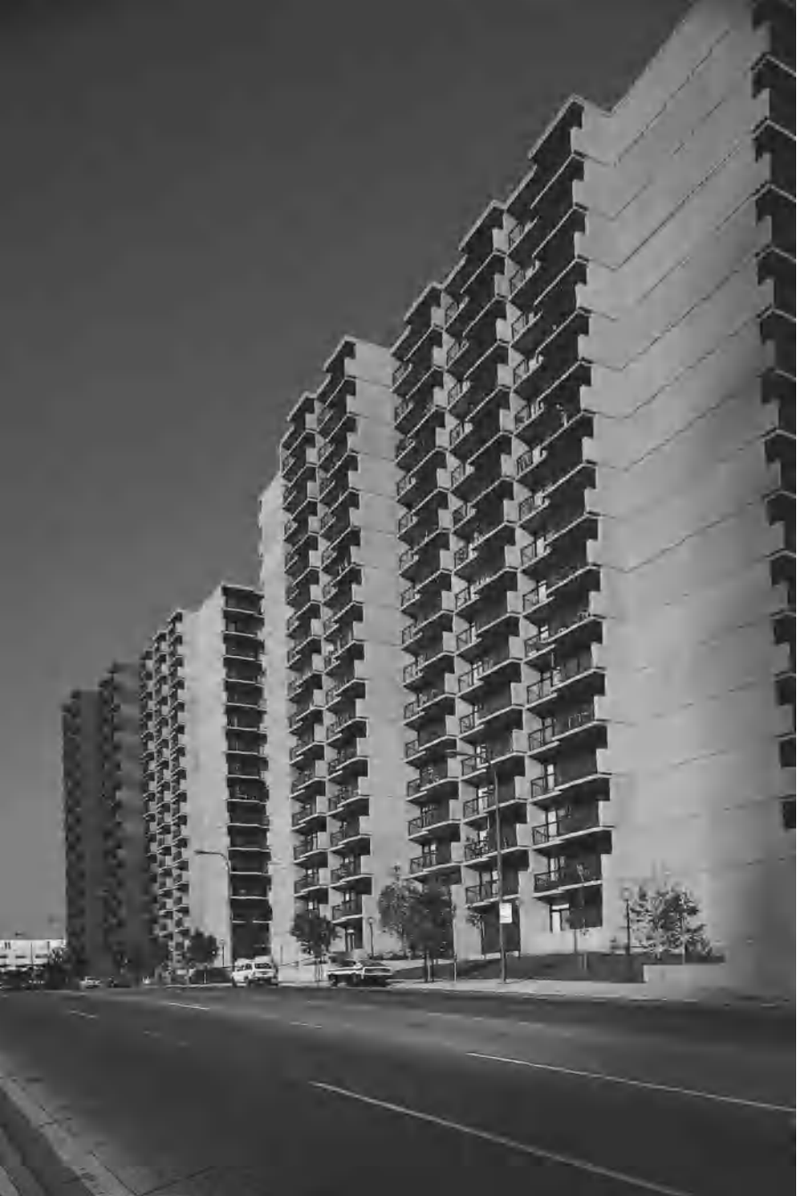
Figure 3.1.15 Precast concrete residential building. (Courtesy of Clark-Pacific.)
