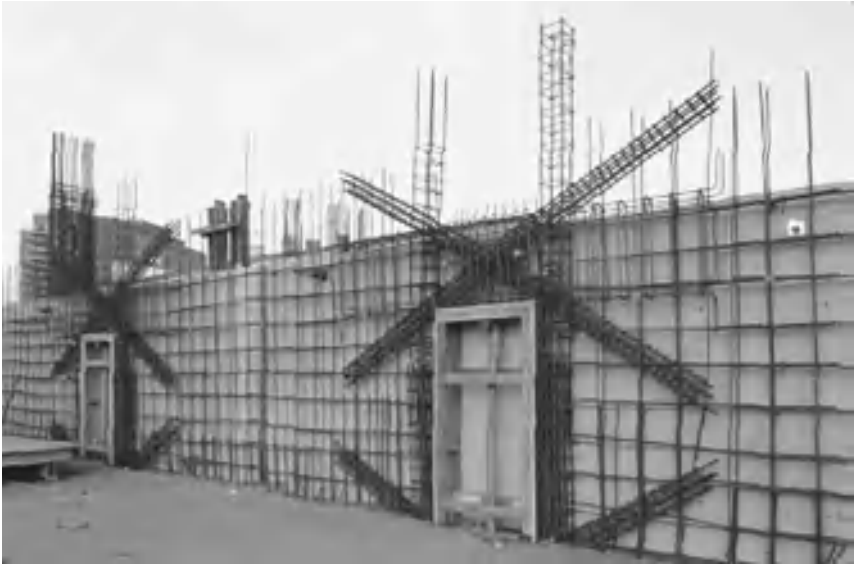
Photo 2.10 Diagonally reinforced coupling beam. (Courtesy of Morley Construction Co.)
