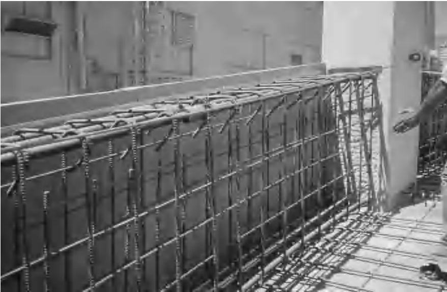
Photo 2.3 Composite frame beam, DDC connection to precast column, Staples Parking Structure, Los Angeles, CA. (Courtesy of Englekirk Partners, Inc.)
