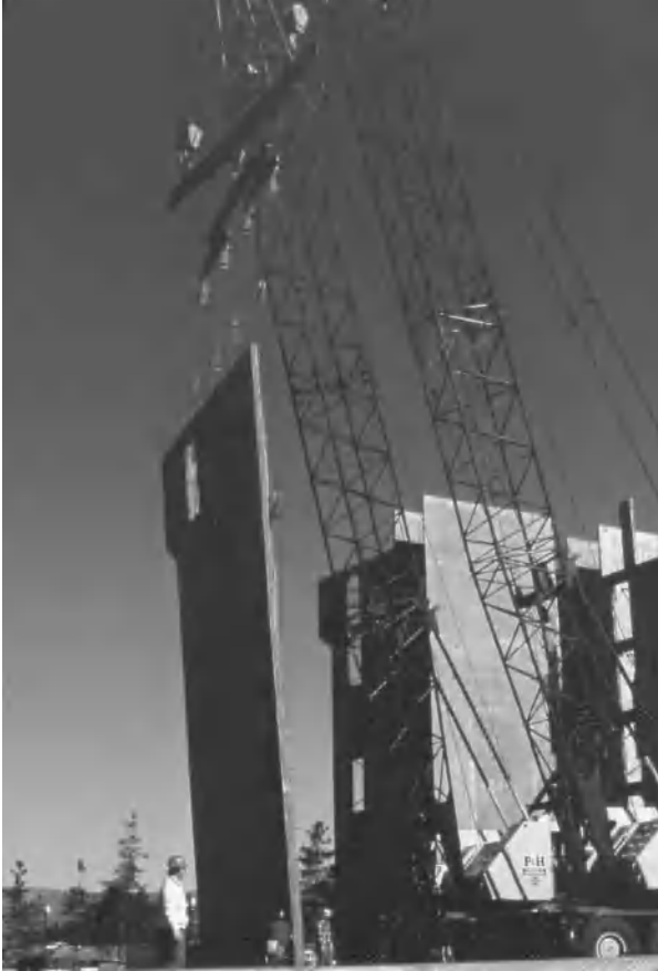
Photo 2.9 Six 6-story precast concrete wall panels, Hilton Hotel, Oxnard, CA, 1968. (Courtesy of Englekirk Partners, Inc.)
