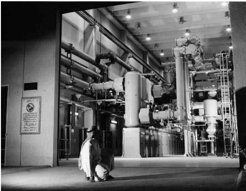
Figure 3.13 Example of 420 kV GIS equipment on a recent substation project in the Middle East (Courtesy VA Tech Reyrolle)
