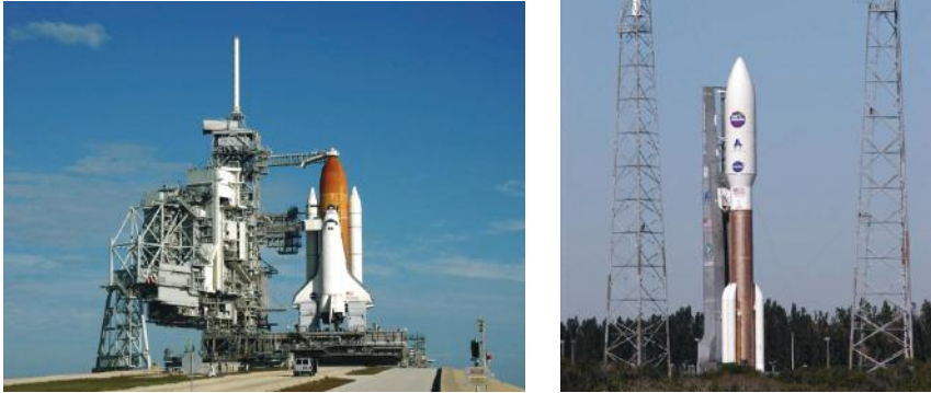
FIGURE 11.6 Lightning discharge towers. (Courtesy of NASA, Washington, DC.)
