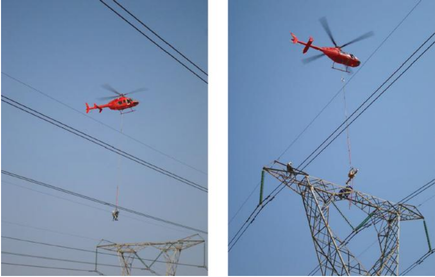
FIGURE 9.10 Helicopter transporting linemen to working site.
