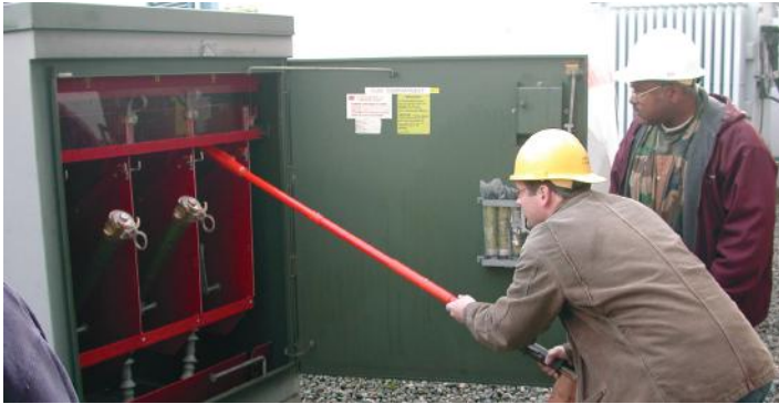
FIGURE 9.6 Using shotgun at ground level. (Courtesy of Seattle City Light.)
