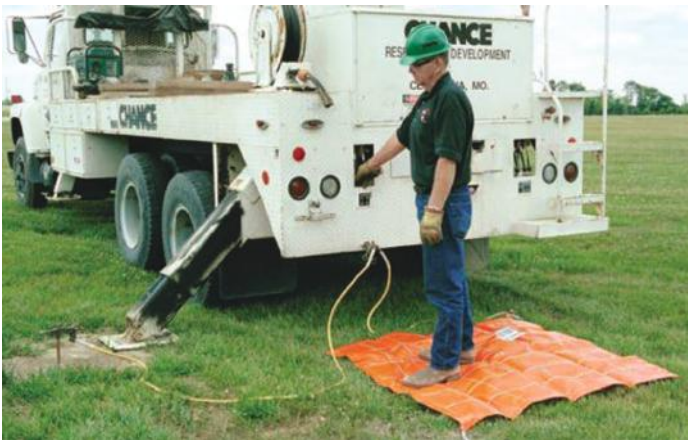
FIGURE 8.21 Worker standing on ground mat attached to truck. (Chance® tools and grounding equipment depicted courtesy of Hubbell Power Systems, Inc.)
