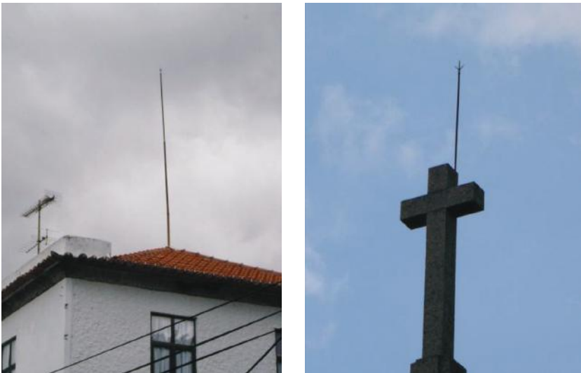
FIGURE 11.5 Lightning pole on top of buildings.
