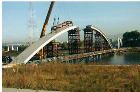
Left: Erection of arch spans Right: Footbridge walkway
