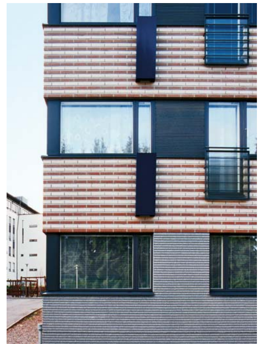
Ribbed finish to ground floor, brick faced above
