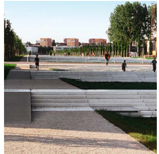
Precast terraces and central channel looking uphill
