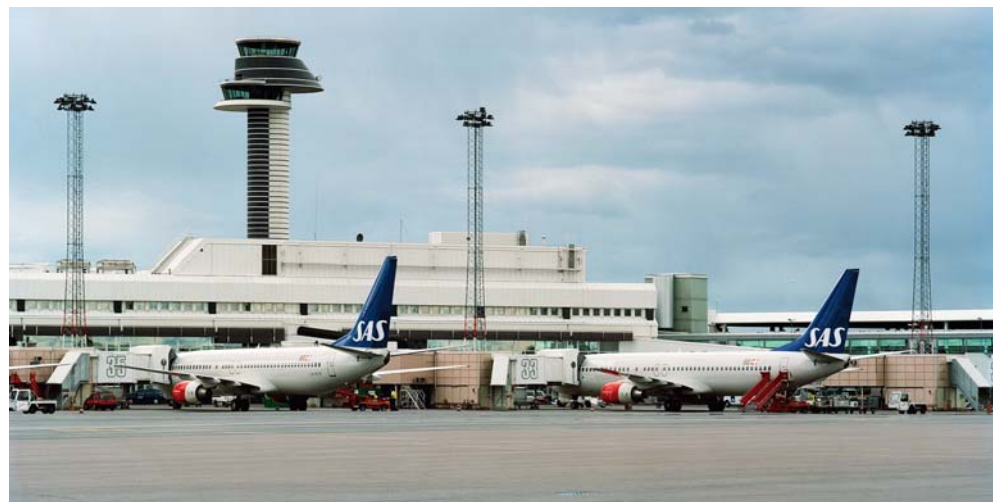
Control tower and aircraft parking apron
