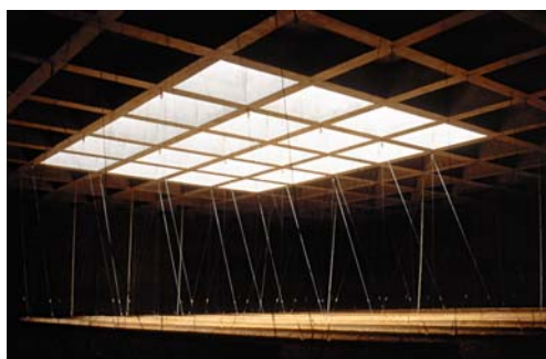
Suspended textile curtain and ceiling roof light
