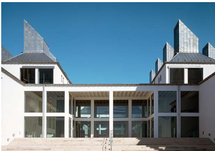
Main corridor and exit leading to waterfront
