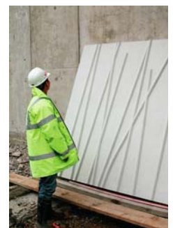
Panels in precast yard
