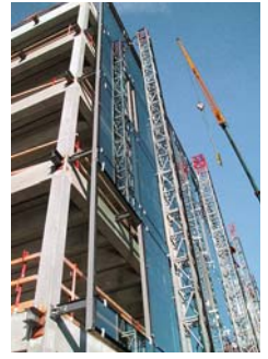
Installation of glass curtain wall
