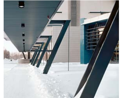
Covered walkway, cranked steel supports
