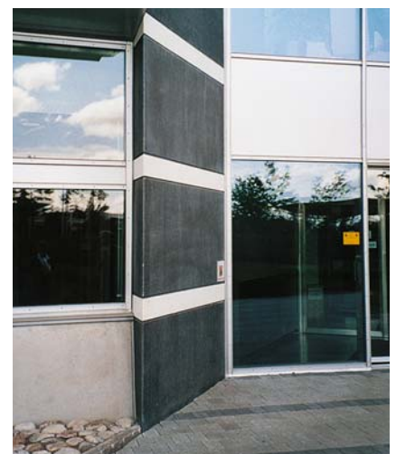
Views of base building façade
