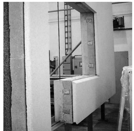
Typical sandwich panel construction
