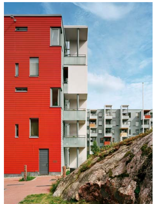
Gable wall with asymmetric window line
