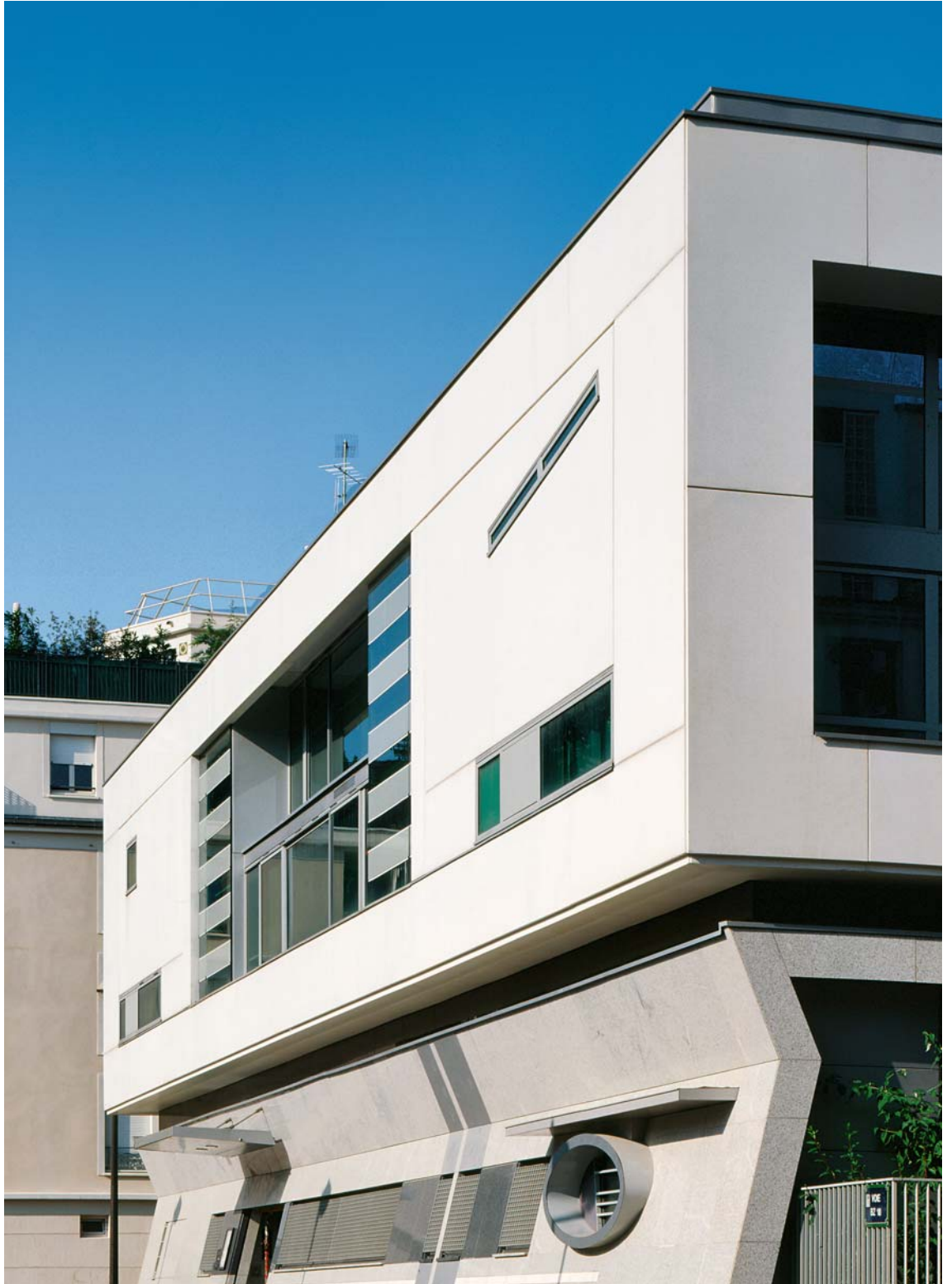
Front elevation facing square, with granite-faced ground level and white precast upper level
