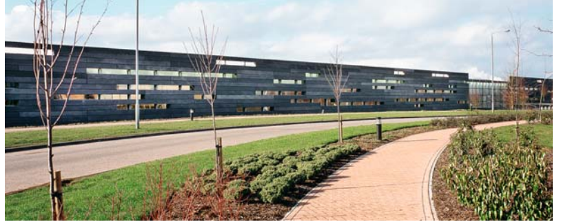
Strong wall and slotted windows
