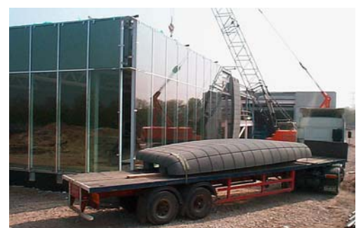
Erection of 17 tonne curved precast panel for Command Centre
