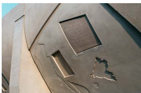
Canongate wall and CNC cut patterns
