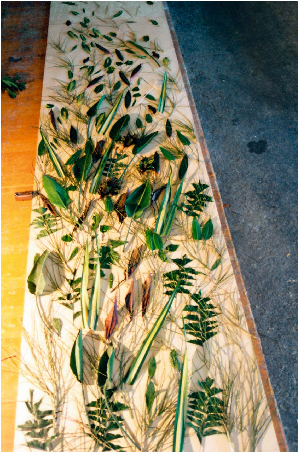
Leaves and branches laid out on the formwork
