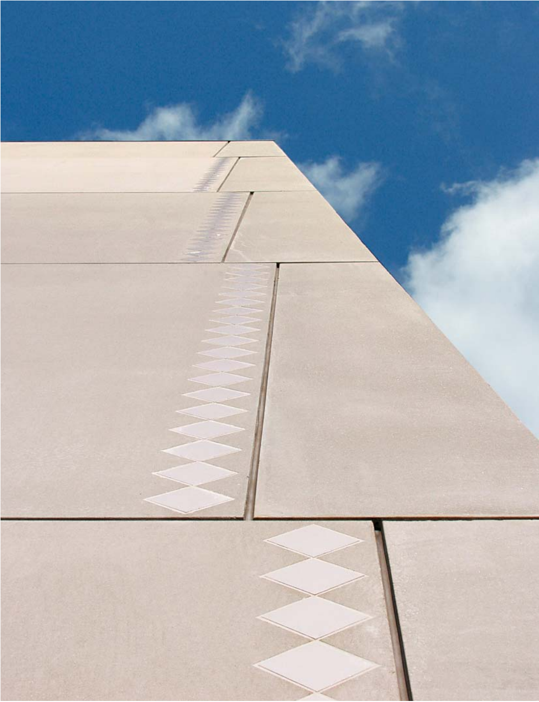
Load-bearing panels and diamond tile motif
