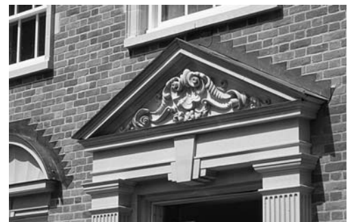
Bottom: Precast quoins corner and decorative features on Shillington Manor, England (dry cast)
