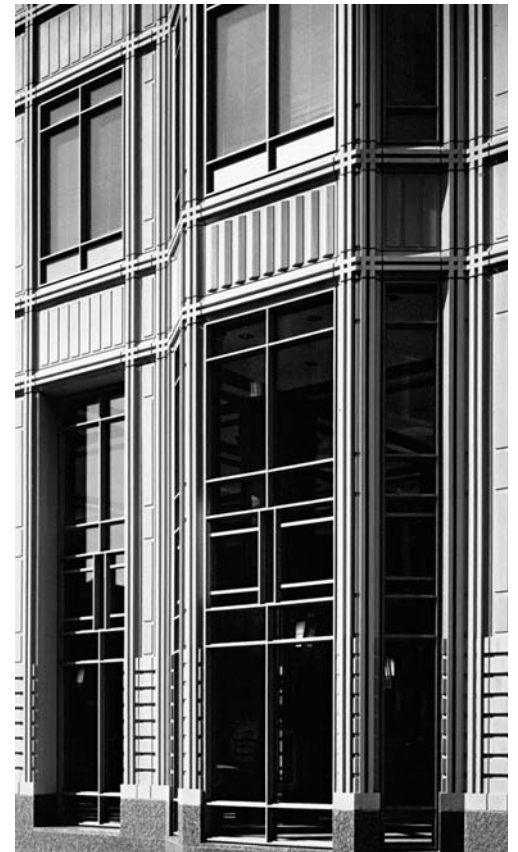
Examples of precast surface finishes Left: Plain white panel design (BDZ Building, Berlin) Upper centre: Surface profiled panel with partial bush hammering Lower centre: Contrasting plain and acid etch finish Right: Highly profiled pigmented panel design (Broadwalk House, London)
