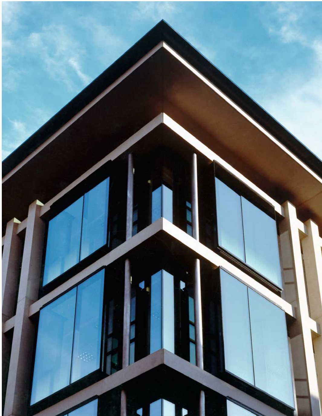
Building corner and cornice
