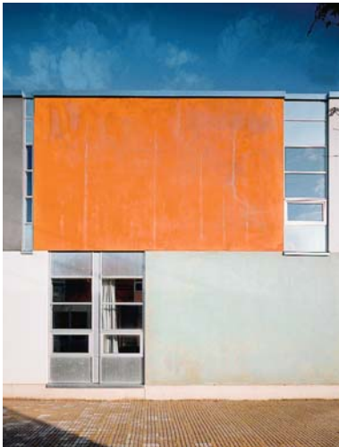
Chemically stained precast
