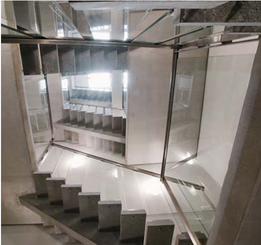
Interior of pylon tower
