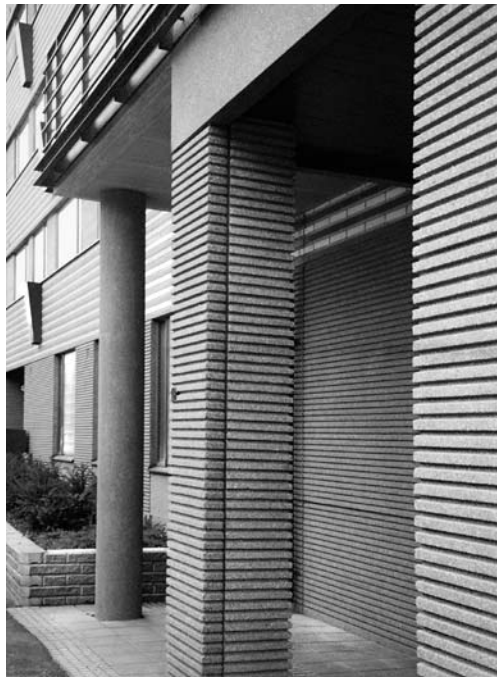
Pigmented precast ribbed and brick-faced panels
