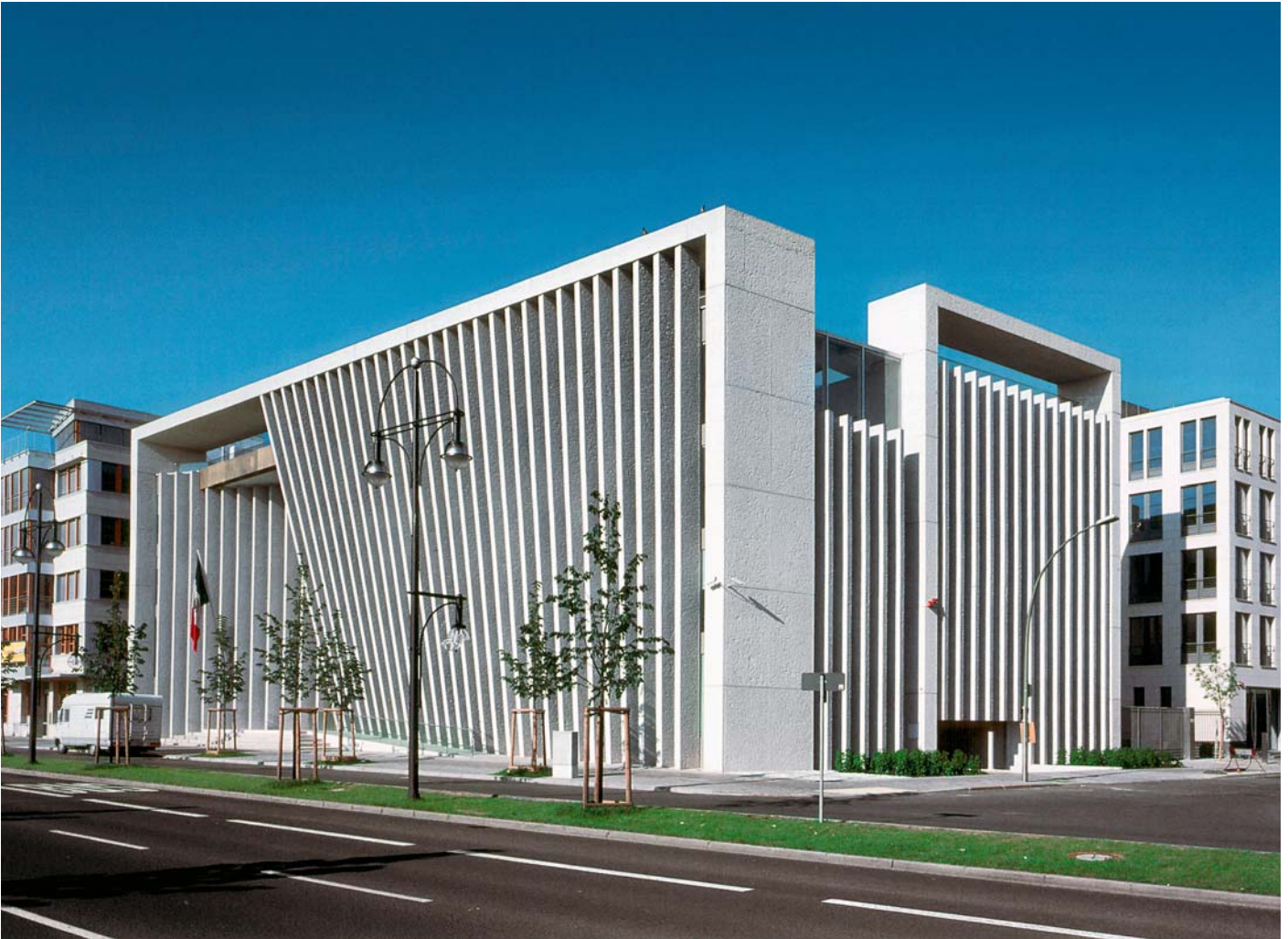
Portal framed blade beam elevations
