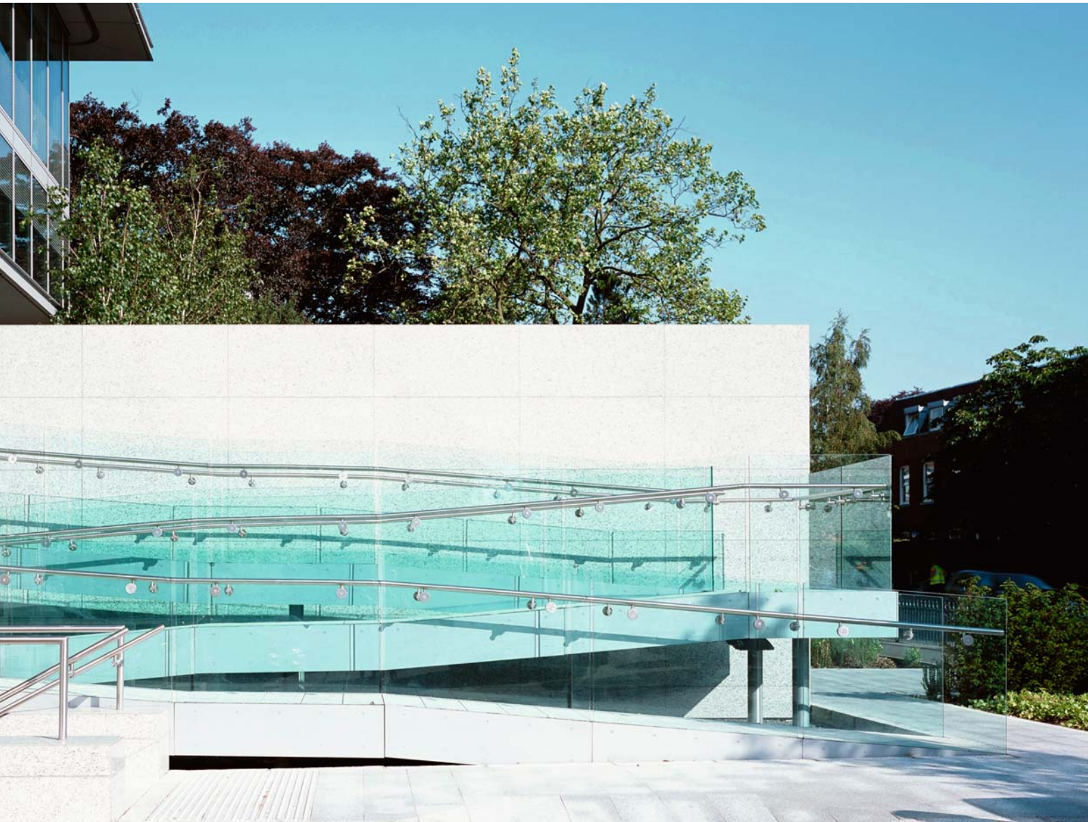
Ramped main entrance
