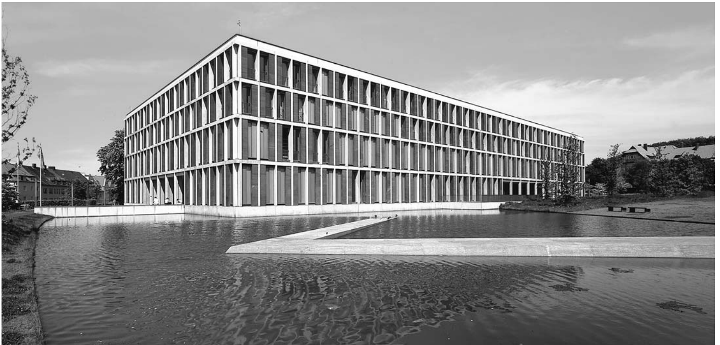
Precision and scale of modern precast design (Federal Labour Court, Erfurt, Germany)
