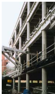
Erection of fascia panels
