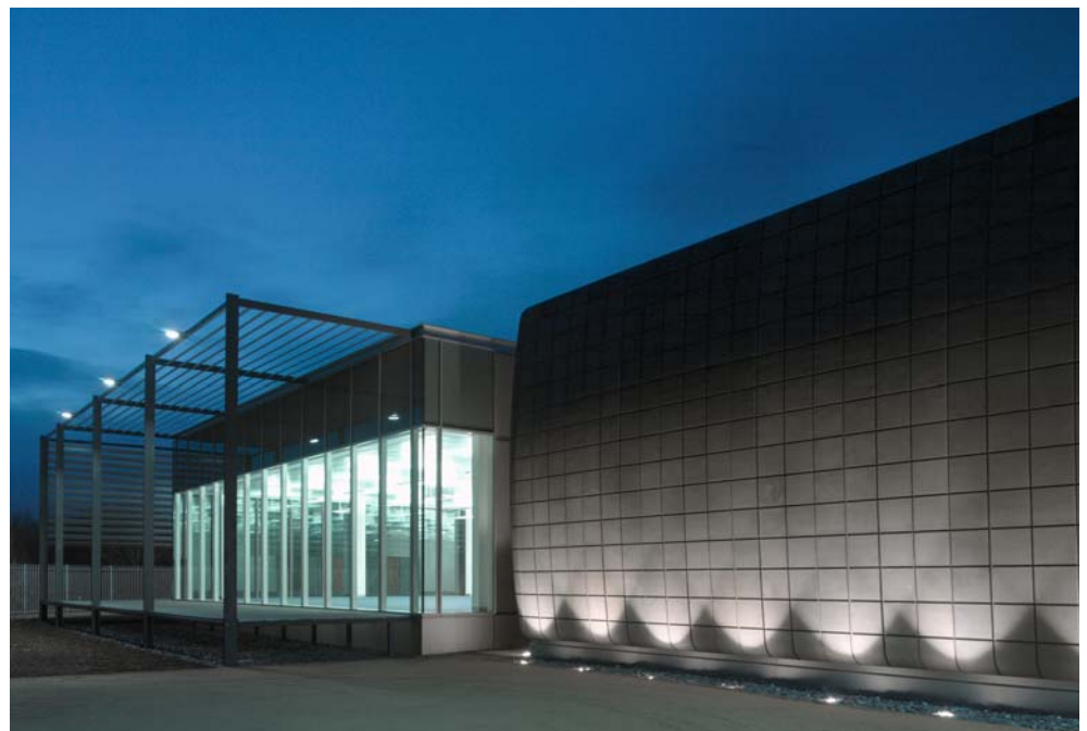
South elevation showing Command Centre and glazed office area
