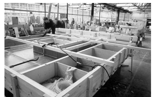
Forming timber master mould
