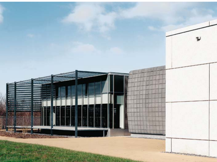
South elevation with white precast sandwich panels in foreground
