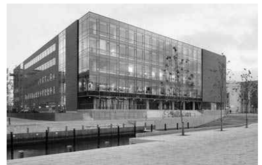
Main elevation, Tuborg 15 building
