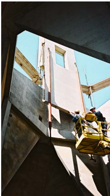
Construction of 'egg box' light well
