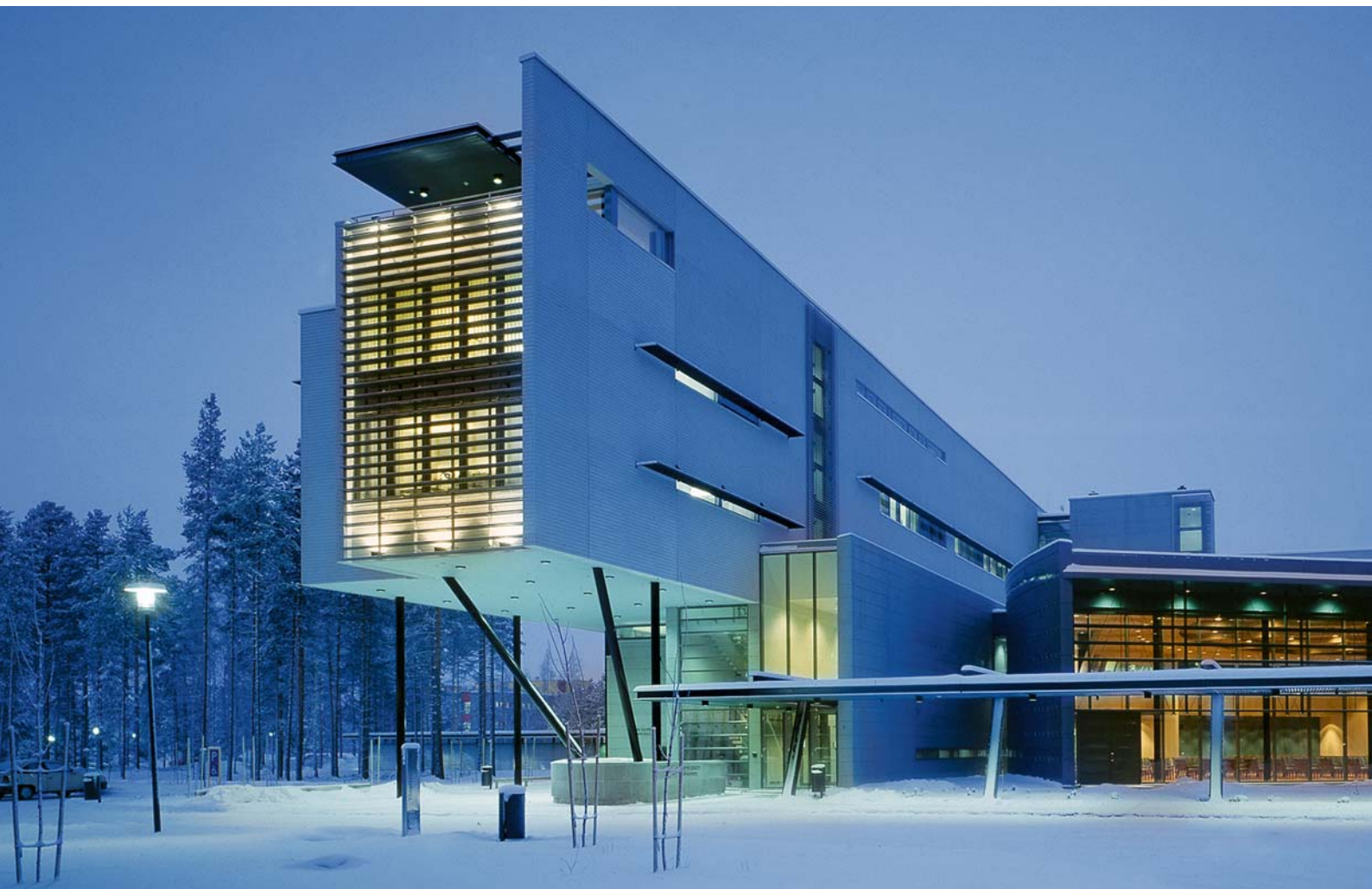
Cantilevered front of main building and splayed columns
