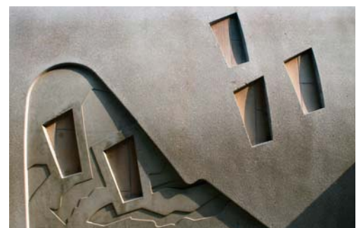
Canongate wall detail
