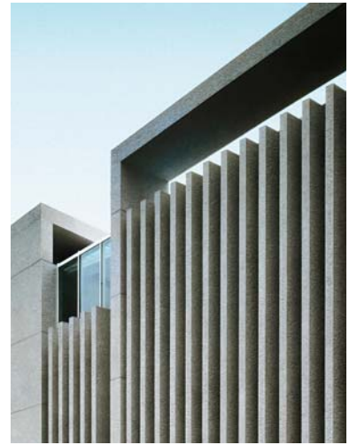
'Blade wall' elevation on the side street
