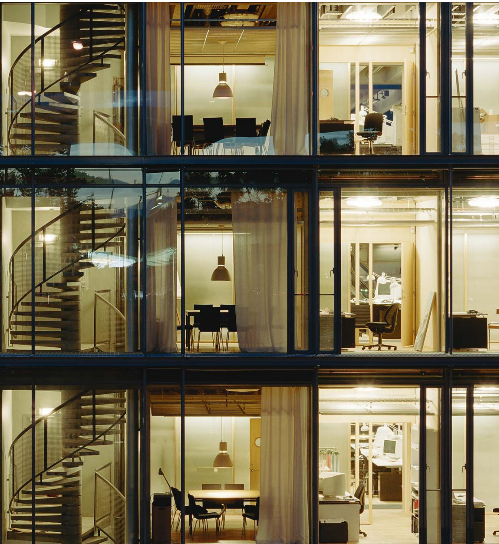
View of main façade
