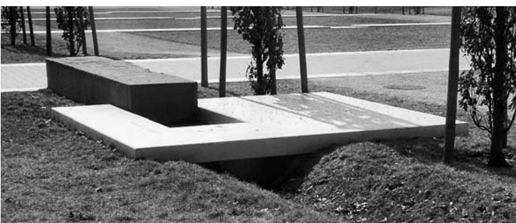
Detail of drainage outlet
