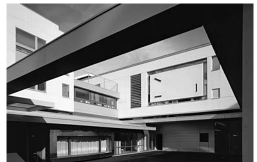
Courtyard space and activity area
