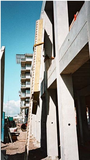
Construction of perimeter colonnade
