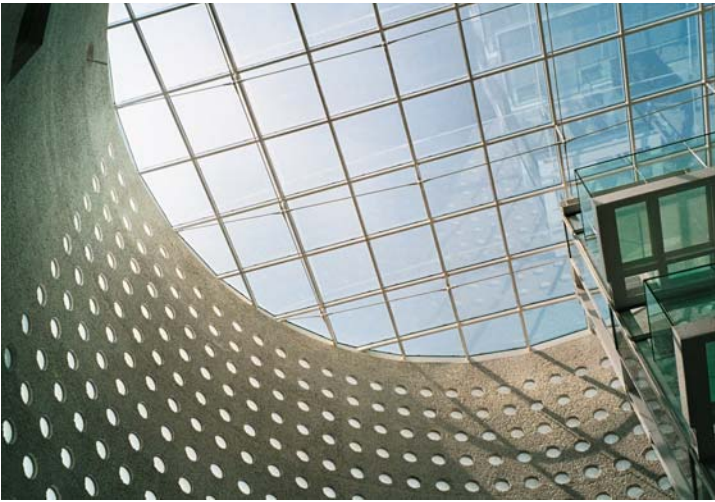
Glass canopy over atrium
