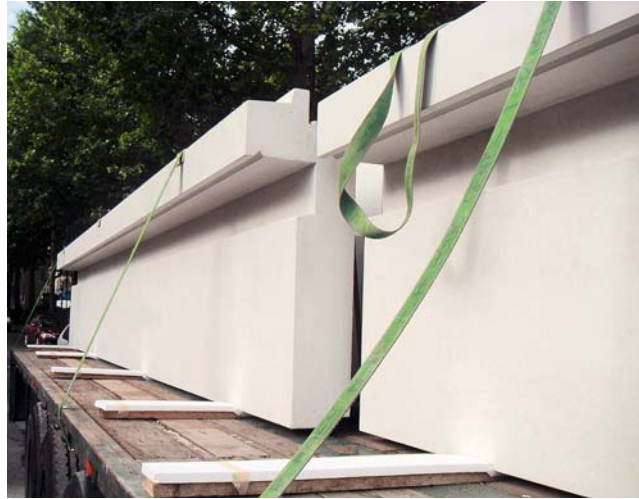
Left: Corner view of the building Right: Façade beams of lower floor
