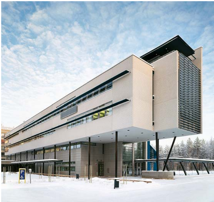
Administration building west elevation
