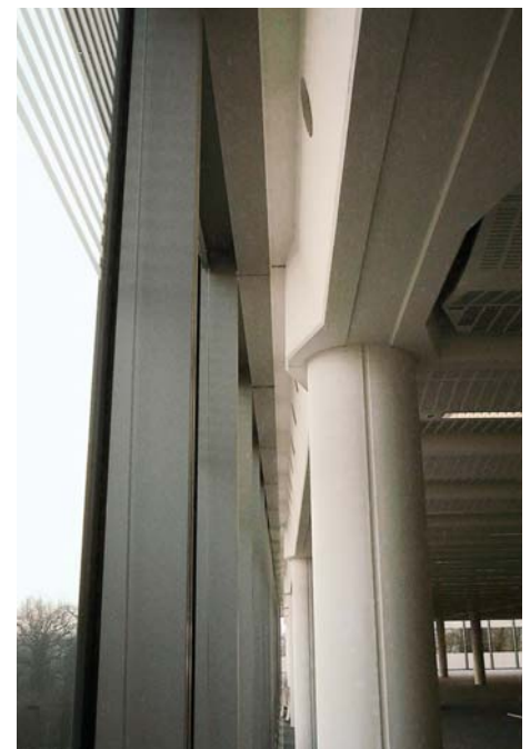
Precast structure exposed behind glass curtain wall
