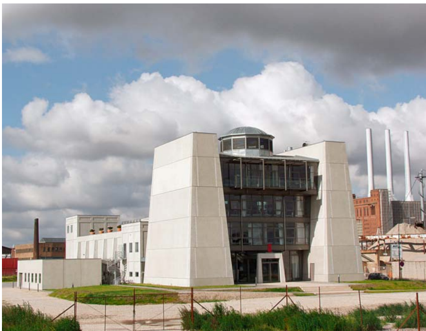
Twin pylon towers
