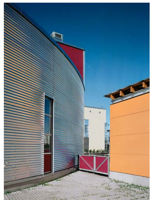
Metal cladding to day centre
