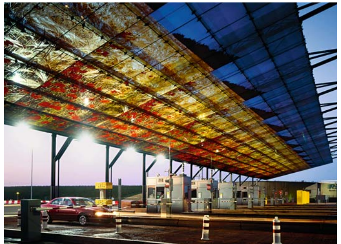
Glass canopy above toll booths
