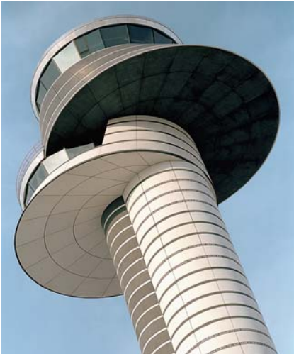
Black precast for the upper and white for the lower control room
