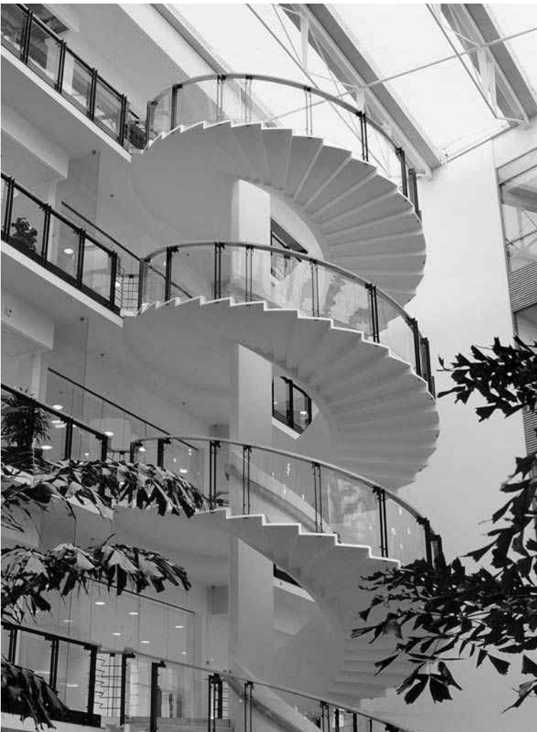
Cantilever treads and curved column profile
