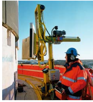
Installing the curved panels for the tower
