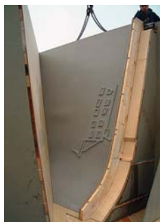
Casting the leading edge panel
