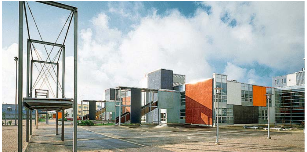
Rear elevation, playground and stair towers
