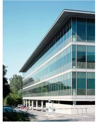
South-west long elevation and undercroft
