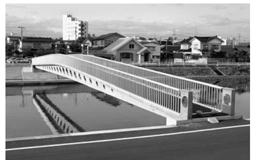
Examples of Ductal® applications: Brise soleils on apartment building Curved roof for train station in Calgary Sakata Mirai footbridge, Japan
