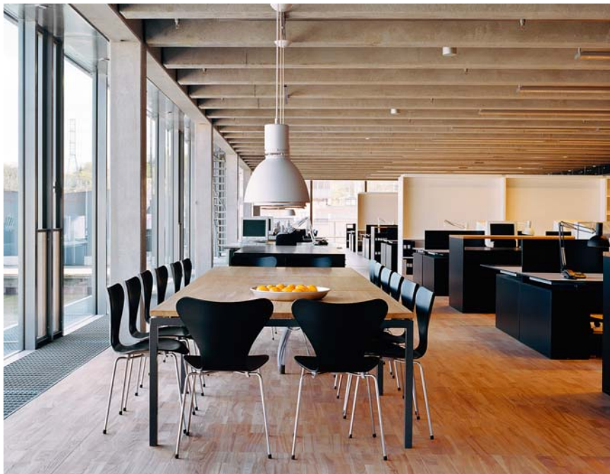
Exposed precast floor beams and columns
