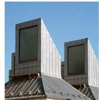
Completed lantern light well
