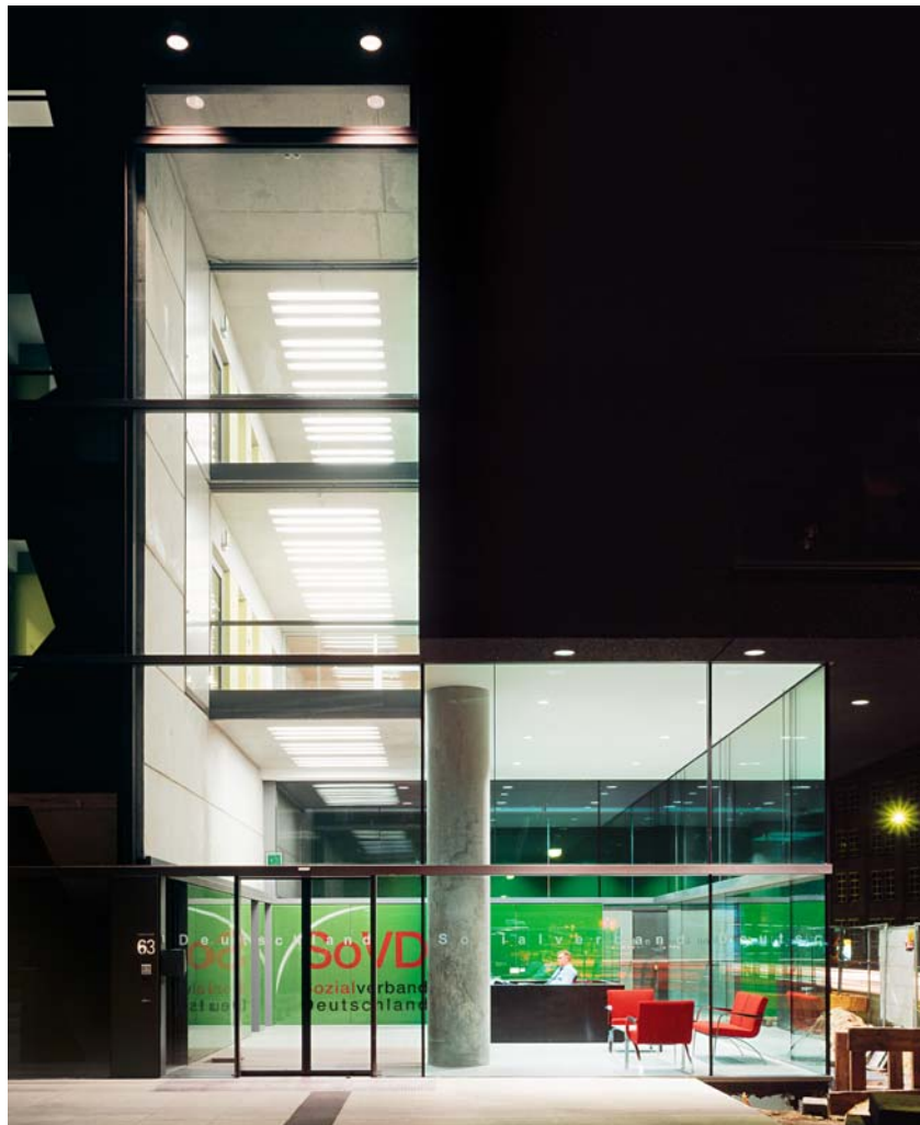
Reception and light well slots on the east elevation
