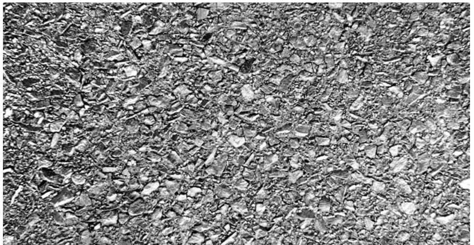
Exposed black aggregate finish
