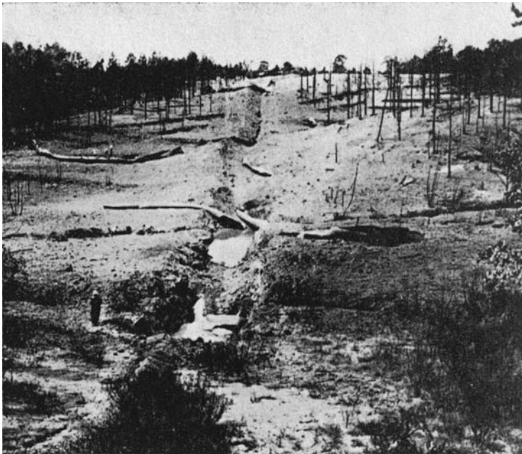
Figure 13.26. A natural gas pipeline that failed during field testing. From E. Parker, Brittle Fracture of Engineering Structures , Wiley, 1957, p. 269.
