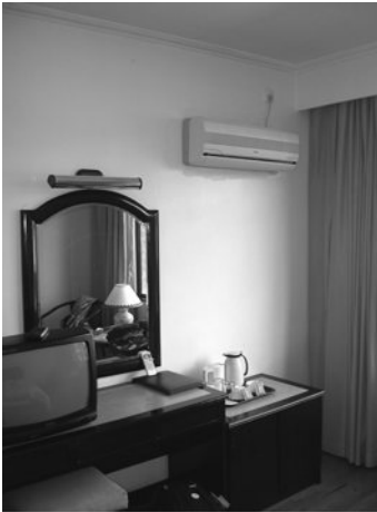
Figure 4-10 Indoor fan coil section of a ductless split system. This type of equipment with a variable-speed tangential fan can be very quiet.
