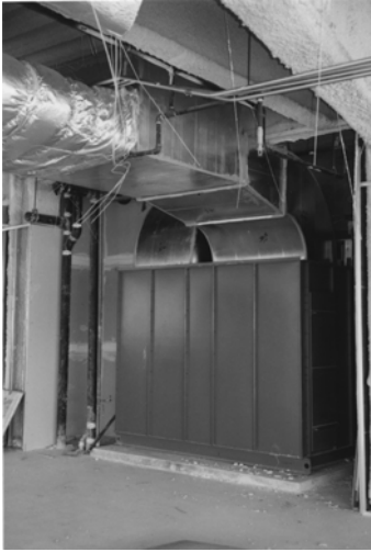
Figure 2-20 Plenum AHU with supply ducts attached to the top of discharge plenum.
