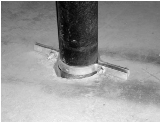
Figure 7-10 Pipe risers without vibration isolation. The pipe clamps transmit pipe vibration to the slab.
