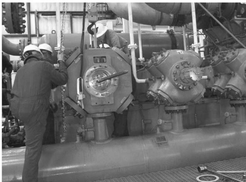
Figure 13-12. The first of six new high-efficiency bolt-in replacement cylinders [left] is installed on a six-throw, single-stage D-R 6HOS-6 frame. Two of the original OEM cylinders are shown on adjacent throws [right] prior to replacement.
