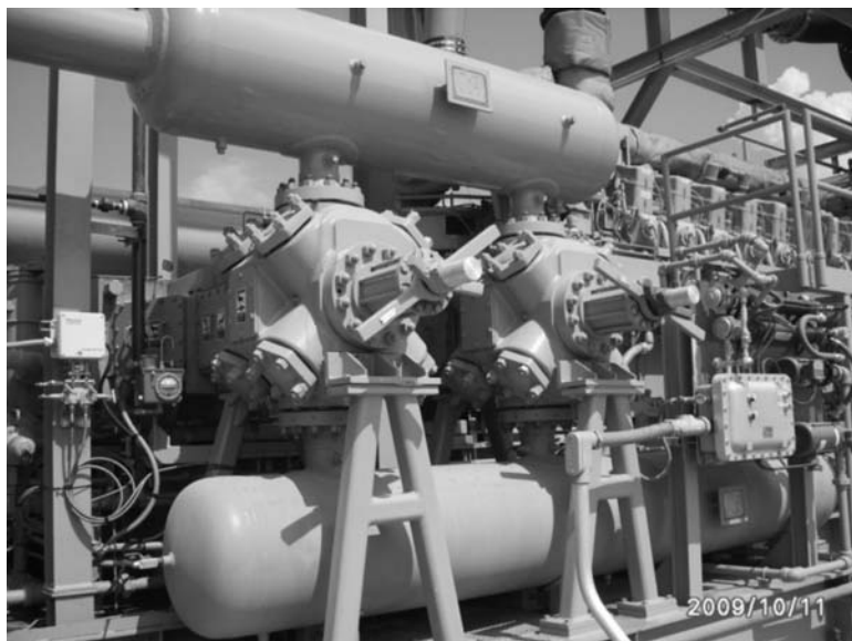
Figure 3-39. Dresser-Rand 7 HOSS-4 Compressors with Suction & Discharge Pulsation Bottles Courtesy of Power & Compression Systems
