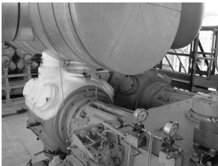
Figure 13-25. Adaptation of 5.5 in. (140 mm) stroke Ariel cylinders to a Superior 6.0 in. (152 mm) stroke Superior compressor frame.
