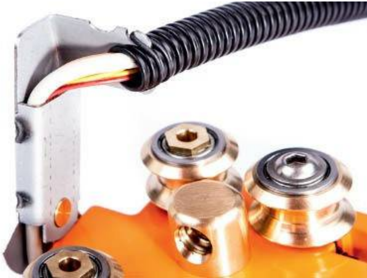
Fig. 2.56 Routing the cable from the gantry to the frame of the machine
