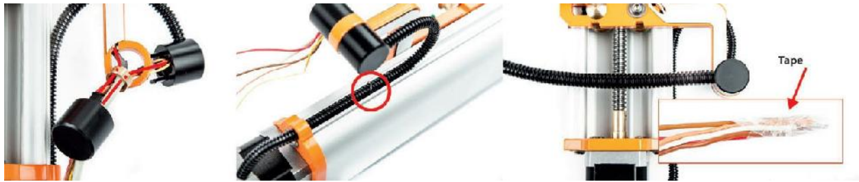
Fig. 2.29 Organizing the cabling
