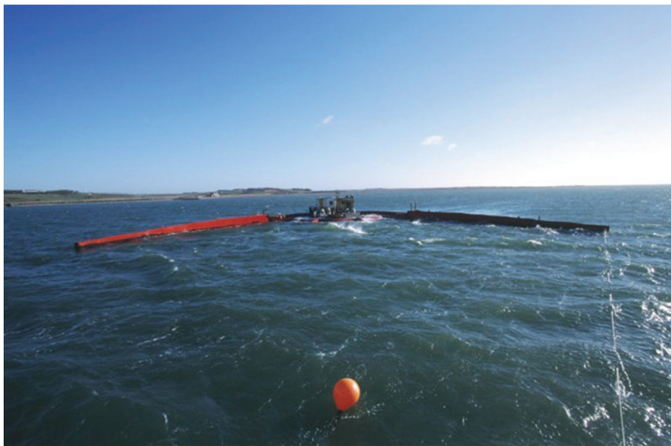
FIGURE 4.79 Front view of the Wave Dragon with wave reflectors in the sides and the reservoir in the middle. (Courtesy of Wave Dragon ApS, available online at http://www.wavedragon.net/ )
