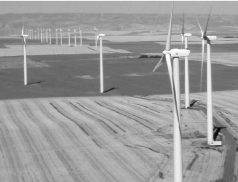
Figure 1.7 Turbine top view of the Klondike wind farm in Oregon, USA. Photo by Author
