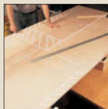
36 Laying Out and Cutting Plywood
